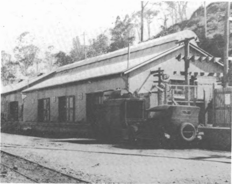
A diesel locomotive adjacent to the compressor house at Somerset Dam, c1937-38.
