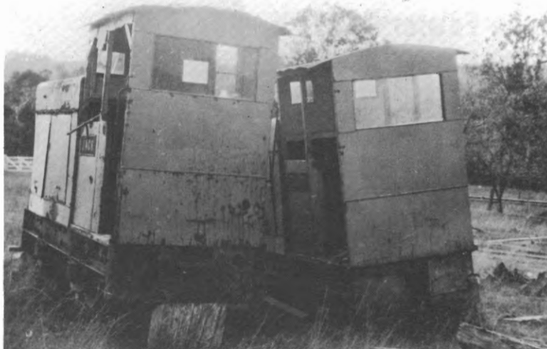
JACK and ARCHIE stored at Mt. Hallon, November 1958.
