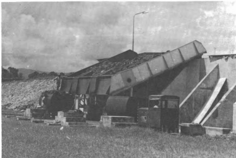
Loading hoppers at Mosa oil palm factory, November 1971. Photo: R. McKillop.
