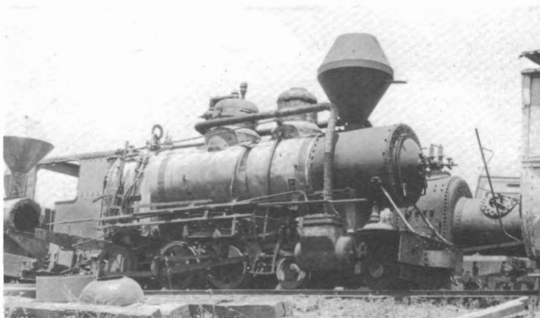
War Department Baldwin 4-6-0 locomotive 42155 or 45215 at Goulburn Waterworks, 24 January 1973.
