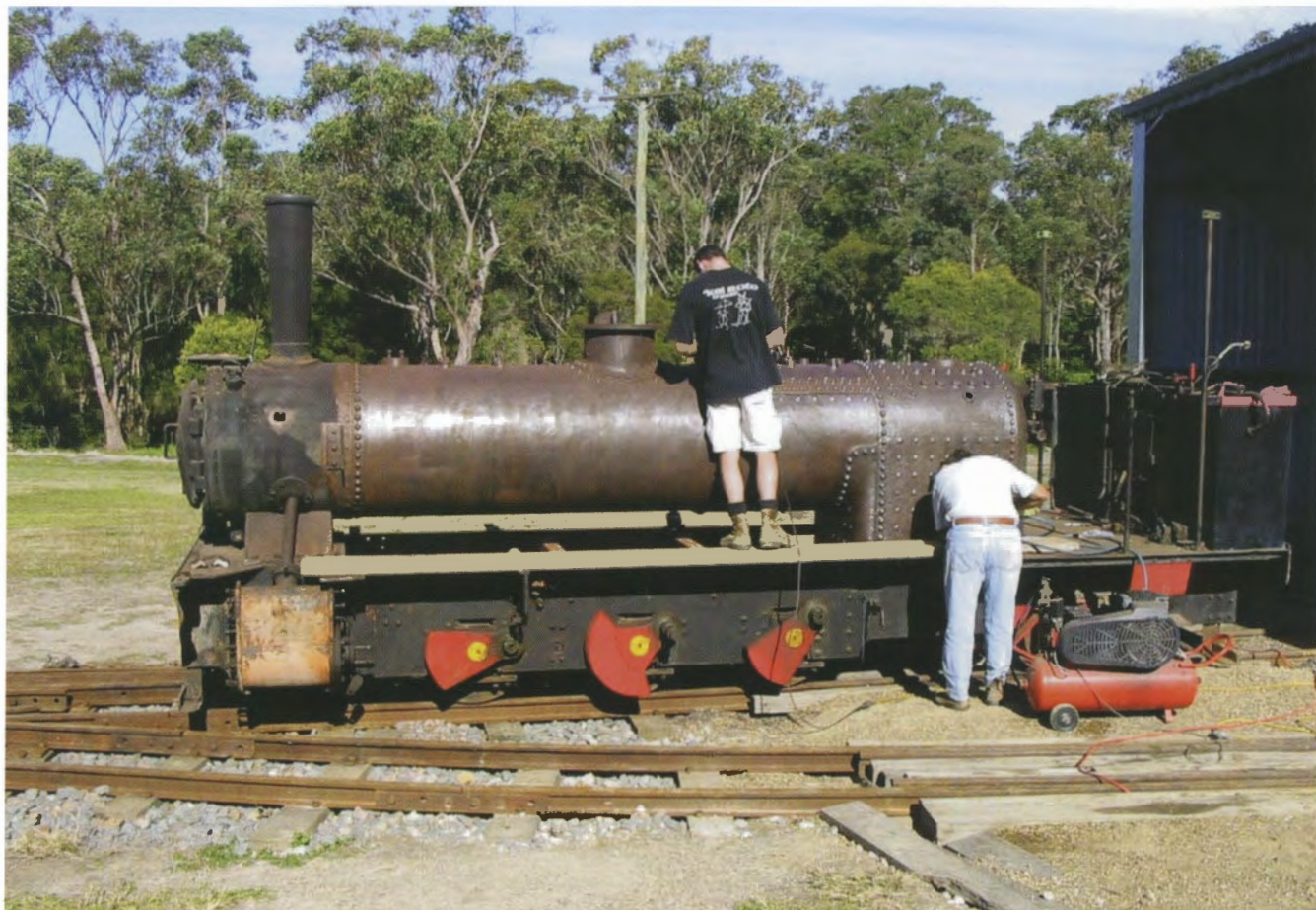
A good rubdown, then... Stripped right down, the boiler drum was thoroughly wire-brushed prior to the application of the protective coating. Meantime, the motion work is under refurbishment in the workshop and the cab is with the welders. Photo: Grahame Swanson
