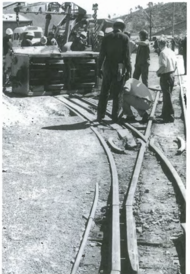
Ten-ton Gemco in trouble in 7 Level yard. A piece of timber was wedged in the road crossing, comprehensively derailing the loco. The battery box parted company with the chassis. Photo: L Johnson Collection
