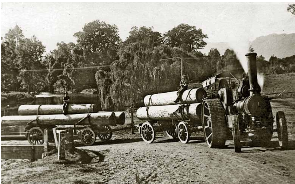
The Bellinger Timber Company first employed bullock teams to haul its pine logs to the Bellinger River for shipment to Sydney. Later it acquired a 7hp Fowler steam traction engine for the six-mile road haul. Photo: Bellinger Valley Historical Society
