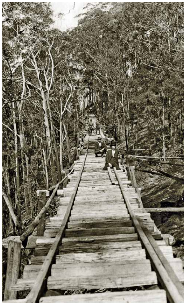
Frank Box and Jack Boulton pose on newly-built timber trestle work on the Gleniffer Incline Tramway during its construction circa 1912.
