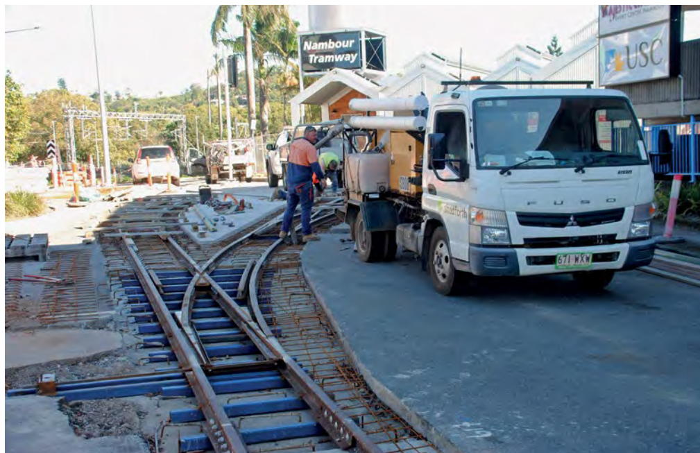
Extensive track work was under way in mid-August installing point work in Mill Street Nambour to connect the old mill tramway track to the various roads into the tramway depot. Photo: John Browning
