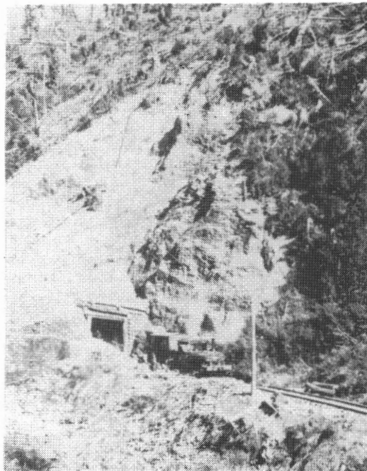
Photograph of North Mt Lyell tunnel through the Razor Back at 3 mile. The locomotive has been identified as MALVOLIO , a Sharp Stewart product (2030/1870) built for the Mersey & Deloraine Railway and converted at Launceston Workshops to 3ft 6in gauge and 0-6-0ST wheel arrangement. It was purchased by the Mt Lyell Company in 1896 and transferred to the North Mt Lyell railway in 1903.
