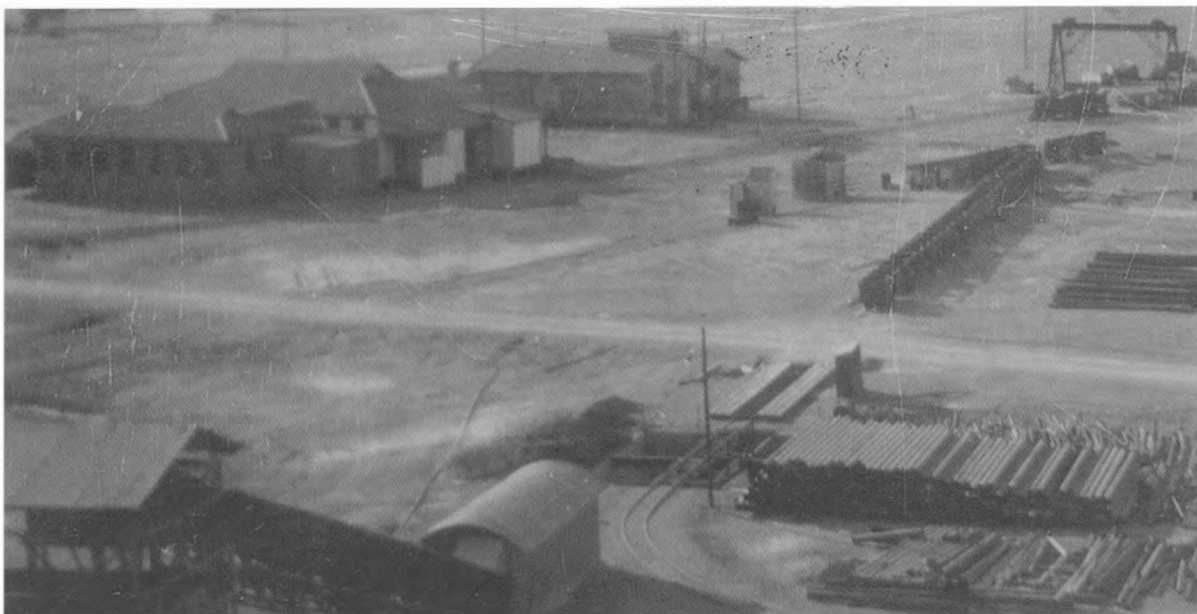
Wiluna Gold Mines Ltd in 1948. A detail of the tramway unloading grizzly with the mine and assay office in the background. The gantry is located over the WAGR 3ft 6in siding to the carpenter's shop. The Moonlight Tramway is almost parallel to the WAGR siding at this location.
