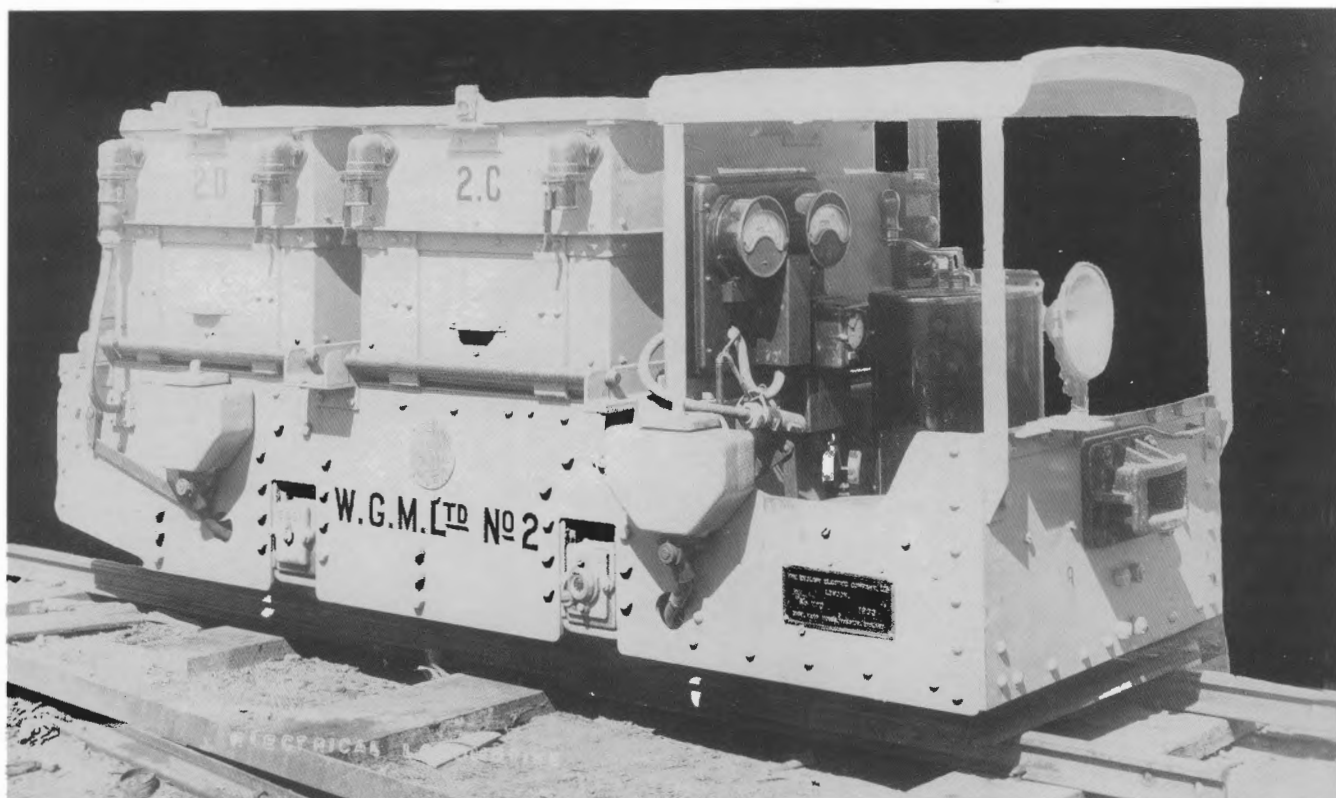
English Electric underground electric locomotives WGM No. 2 (770 of 1930)
