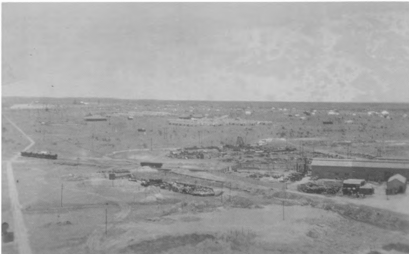
Wiluna Gold Mines Ltd in 1935. The lighter coloured road to the left of the photo is in fact the 2ft gauge Moonlight Tramway. The dogleg in the tramway alignment is to facilitate the WAGR Midland workshop-built diamond crossing. A rake of three Jf 5000 gallon tank wagons can be seen literally on the diamond crossing. The sheds at right were listed as stores for the mine accessed by a WAGR 3ft 6in gauge mine siding.
