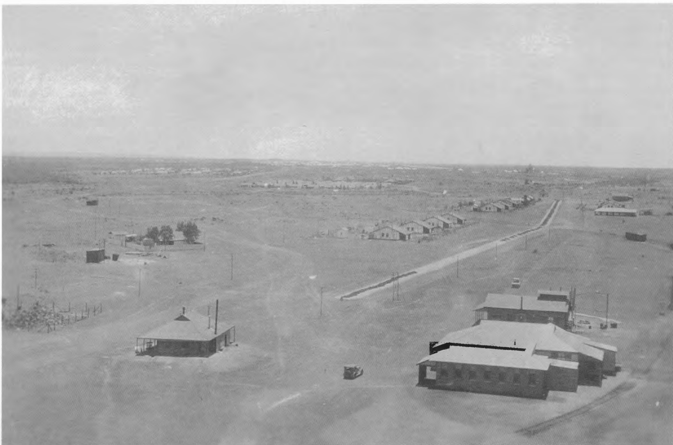
The photographer has rotated slightly to his left to take this second view showing the mine offices and Assay Office in the foreground. Just in front and barely discernable is another leg of the WAGR mine siding to the carpenters shop. Curiously, in the middle of the photo appears to be an attempt to site the Moonlight Tramway, with formation and sleepers still apparent. This was relocated to the right, just off the photograph.
