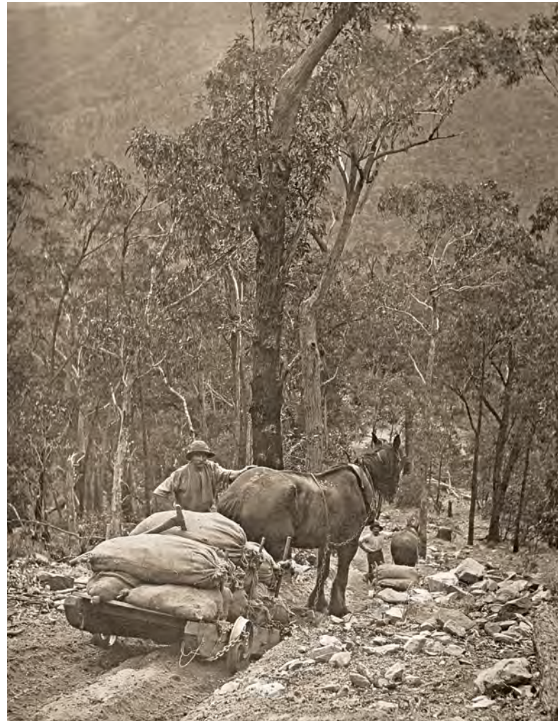
Sledging quartz down to the battery at the New Good Hope, before the machinery was shifted from Crooked River and closer to the mine in 1913. Of note are the tramway wheels on the rear of the sled. Photograph by John Jackson in 1911, State Library of Victoria image H21169.
