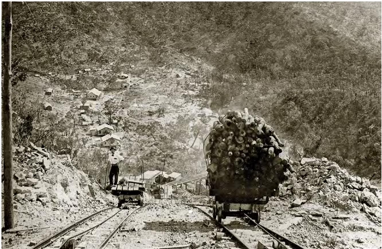
Above: The Arbouin or "18 Mile" siding and ore loading bins were located on a shelf above the Basin Gully ravine. Ore was taken from the mine along a horse-drawn tramway a distance of about 1 mile, then via a flying-fox 650 ft in length, with the tub containing a little over 1 ton of ore. This siding was installed in 1905 allowing the ore trucks to be loaded without blocking the main line, and facilitating the operation of a shuttle service to Rocky Bluff. The ore wagon hoppers are from Arthur Koppel, Berlin (along with some, perhaps all of the metal work) and the trucks constructed at the Stannary Hills workshop. The hoppers may look like "side tippers" but they would carry about 3 tons of ore, and other photographs show they are bolted securely to the wagon frame, the contents being emptied by the whole truck being hand propelled onto a tumbler, and upended over the ore bin at Rocky Bluff. The locomotive shunting the loaded ore-trucks is either Falcon (Brush) 291 or 292 of 1901. Photo: John Oxley Library, State Library of Queensland. Image No 27921-0001-0144
