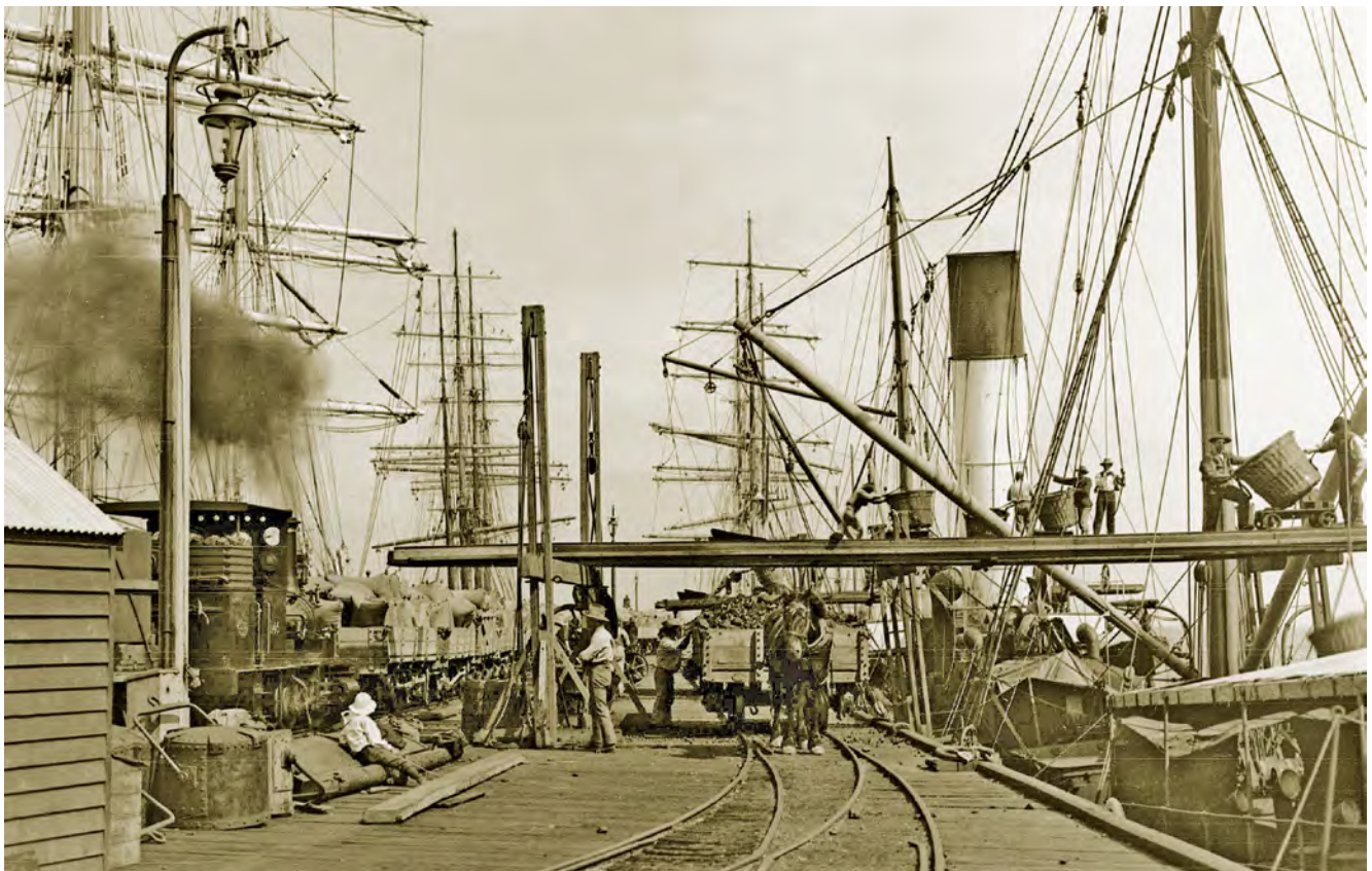
This undated (early 1900s?) scene on Wallaroo jetty in South Australia shows some of the dangers of coal-lumping using the “basket and tram” method described in the article. The staging is about ten feet above the jetty and possibly 20 feet or more, above the coal in the ship's hold. There is one trolley on each track and there are three tracks on the nearest staging. Each basket held a bit less than ½ cubic yard (approx 8 cwt) of coal. In 1905/6, some 73,200 tons of coal and 6400 tons of coke were imported to Wallaroo, all being unloaded as shown and most destined for the Wallaroo Copper Smelters. At left SAR 0-4-4T V145 (Martin 69/1893) is shunting a long line of trucks with grain for export, the whole scene being watched over by the inevitable young lad. At many ports a coal-lumpers' union was formed. In Sydney, by 1905, they had an Award that detailed pay per basket, basket size, meal times, smoke-oh's etc – but little about safety! Photo: courtesy History Trust of South Australia ref GN05330
