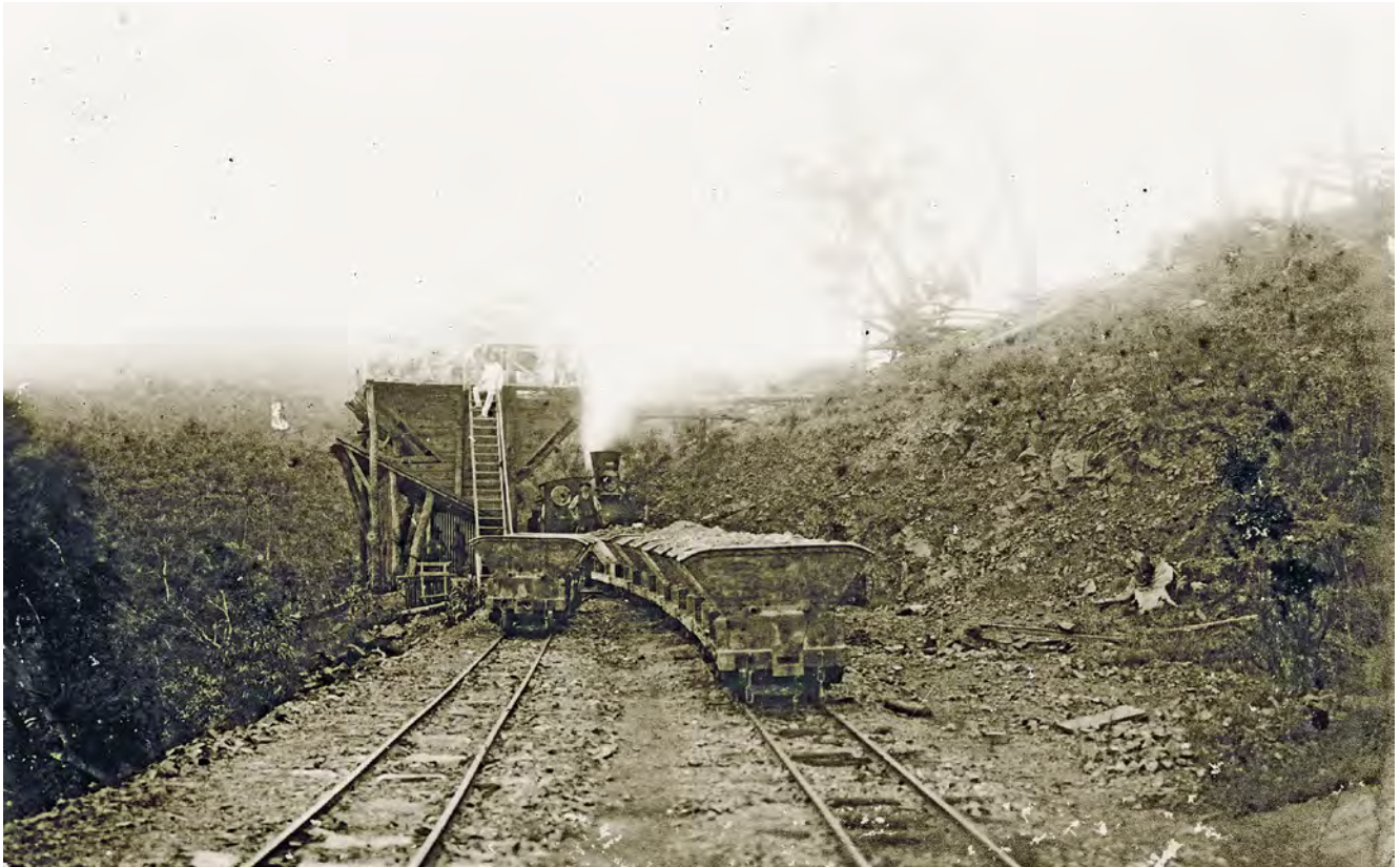
Above: The Arbouin or "18 Mile" siding and ore loading bins were located on a shelf above the Basin Gully ravine. Ore was taken from the mine along a horse-drawn tramway a distance of about 1 mile, then via a flying-fox 650 ft in length, with the tub containing a little over 1 ton of ore. This siding was installed in 1905 allowing the ore trucks to be loaded without blocking the main line, and facilitating the operation of a shuttle service to Rocky Bluff. The ore wagon hoppers are from Arthur Koppel, Berlin (along with some, perhaps all of the metal work) and the trucks constructed at the Stannary Hills workshop. The hoppers may look like "side tippers" but they would carry about 3 tons of ore, and other photographs show they are bolted securely to the wagon frame, the contents being emptied by the whole truck being hand propelled onto a tumbler, and upended over the ore bin at Rocky Bluff. The locomotive shunting the loaded ore-trucks is either Falcon (Brush) 291 or 292 of 1901. Photo: John Oxley Library, State Library of Queensland. Image No 27921-0001-0144
