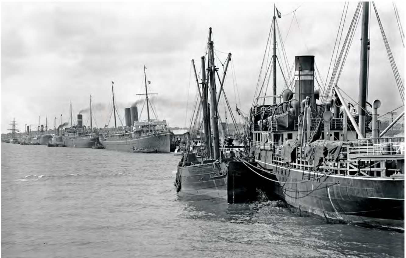
A busy scene in Fremantle harbour, c.1905. The nearest vessel is the ss Moira, with a coal hulk alongside. The accompanying enlargement of the centre portion (left) shows that the photographer captured the moment coal was being trammed across from the hulk to the steamship. The elevated nature of the tram line and the obvious risks involved is well illustrated – imagine doing this if the waters were unsettled and it was night time, during a sudden squall. Note the donkey engine on the left side of the hulk for powering the winches. The 2184-ton Moira was built by W Denny & Bros., Dumbarton, Scotland in 1901. She was 301ft long, and 42ft wide. Sold by AUSN Co Ltd in 1926 to Toyo Kaiun KK, Japan; she was sunk by a US submarine in August 1944 off the Ryukyu Islands. Photo: State Library of WA ref 009674PD
