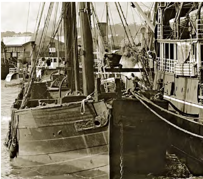
A busy scene in Fremantle harbour, c.1905. The nearest vessel is the ss Moira, with a coal hulk alongside. The accompanying enlargement of the centre portion (left) shows that the photographer captured the moment coal was being trammed across from the hulk to the steamship. The elevated nature of the tram line and the obvious risks involved is well illustrated – imagine doing this if the waters were unsettled and it was night time, during a sudden squall. Note the donkey engine on the left side of the hulk for powering the winches. The 2184-ton Moira was built by W Denny & Bros., Dumbarton, Scotland in 1901. She was 301ft long, and 42ft wide. Sold by AUSN Co Ltd in 1926 to Toyo Kaiun KK, Japan; she was sunk by a US submarine in August 1944 off the Ryukyu Islands. Photo: State Library of WA ref 009674PD
