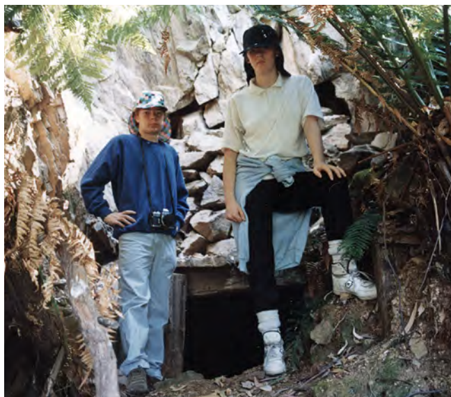
The entrance to the No.4 adit at the time of survey in January 1992. Photo: Peter Evans
