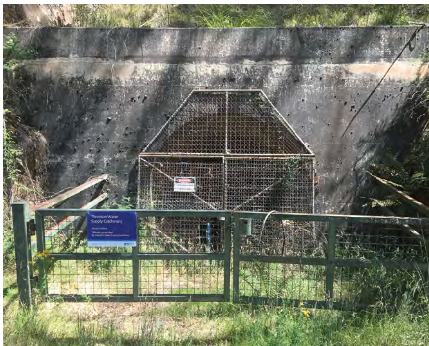
Thomson portal tunnel entrance. Photograph: David Malady.
