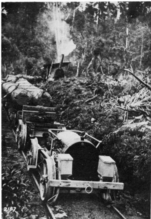
Nattrass tractor with Cadillac engine on test run at Pukeweka Sawmilling Coy, Manunui, NZ 1928.
