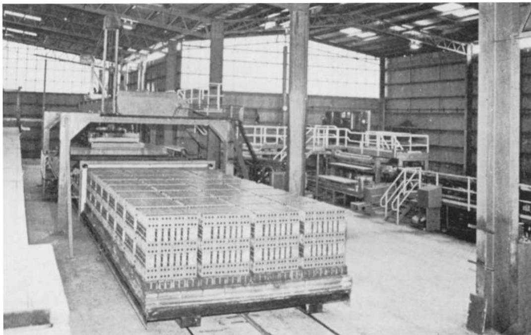
Bricks set on kiln cars awaiting drying and firing at Selkirk brick plant No. 2 in 1982.
