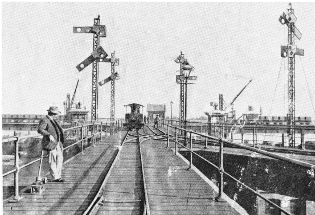
View looking towards wharf showing track layout of 1890 with route indicator signals applying in both directions.
