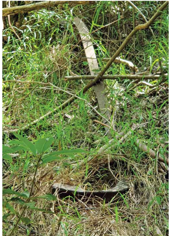
Section of light rail at the top of the cutting at the southern-most loading point on O'Keefe's ballast pit tramway, demonstrating that a separate tramway system very likely delivered ballast to the loading bins. Photo: Peter Evans.
