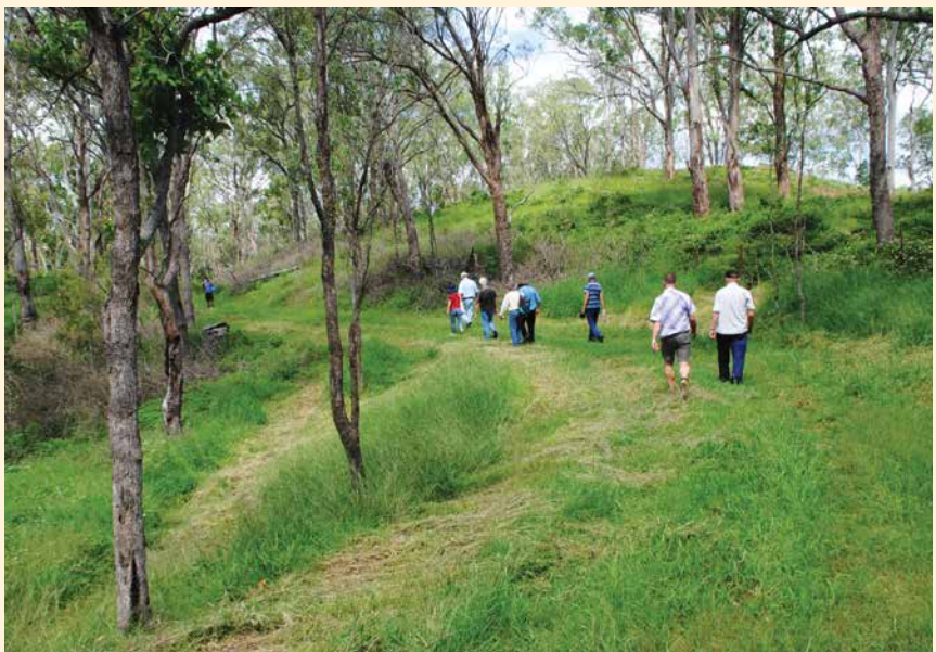
Munro's Hampton Tramway formation near the McQuillan's bridge site. Photo: John Browning
