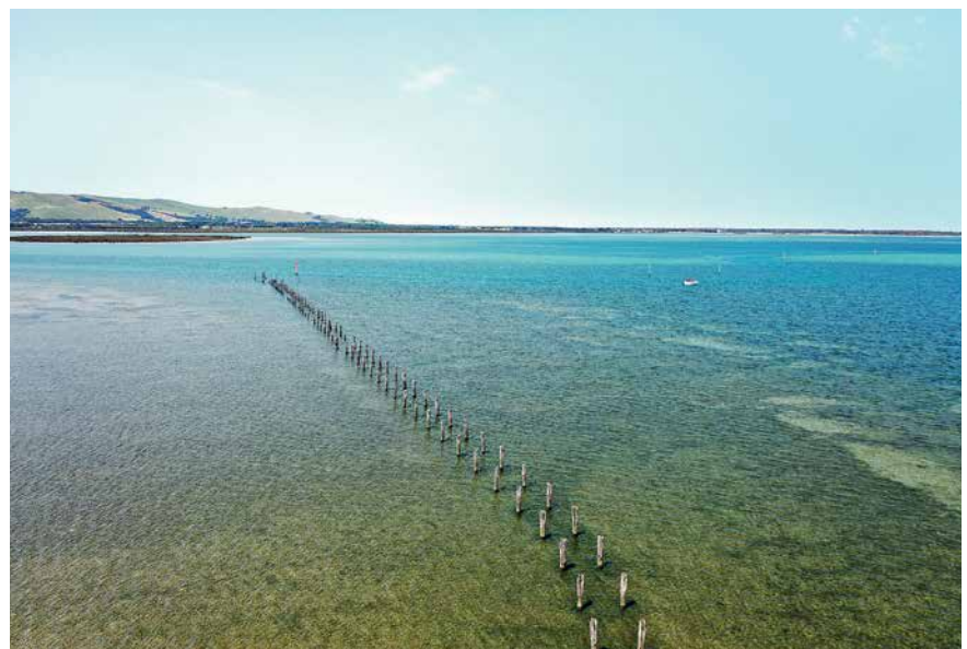
Remains of the 'New Jetty' at Toora are only visible at low tide. Photo: Mike McCarthy (via drone).
