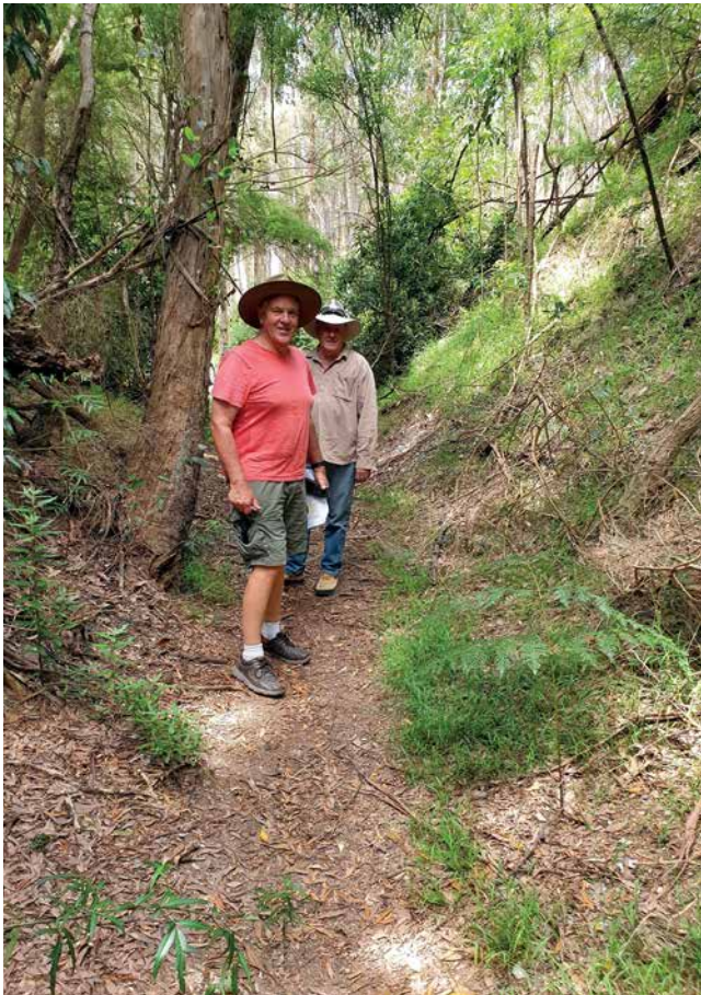
Mike McCarthy and Chris Wurr in the cutting at the southern-most loading point on Andrew O'Keefe's 5 ft 3 in gauge ballast pit tramway at Foster. Photo: Peter Evans.
