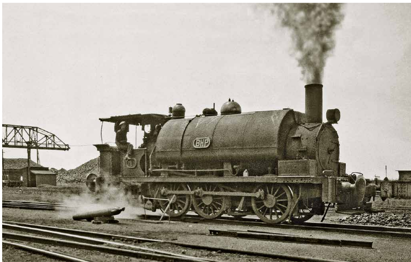
Vale & Lacy 5/1870 had a long and varied career. Starting as a NSWGR 0-6-0 tender locomotive, No.40 of the class 17, it was withdrawn from service in 1892. Subsequently it was used by the PWD and later Smith & Timms on railway construction work before being acquired by BHP in 1913. Numbered 1, it was converted to a saddle tank the following year with a rather spartan cab as shown. In a later rebuilding it received a more stylish cab. It was generally known as 'Old Lizzie'. Sadly, it was scrapped in 1960 after ninety years' service.
