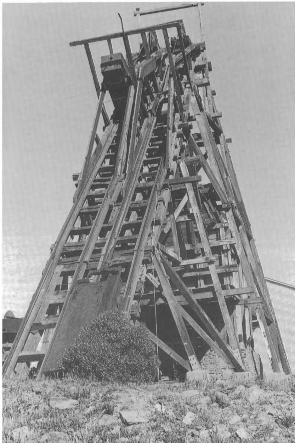
Sons of Gwalia head frame in current re-erected position at Gwalia, 1991 Photo: David Whiteford.
