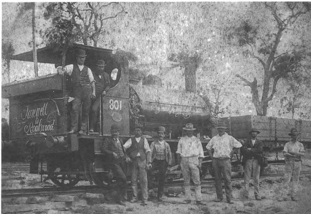
Above: Vulcan Foundry 801 at Potts Hill Reservoir 1890? Photo: Bruce MacDonald Collection.
