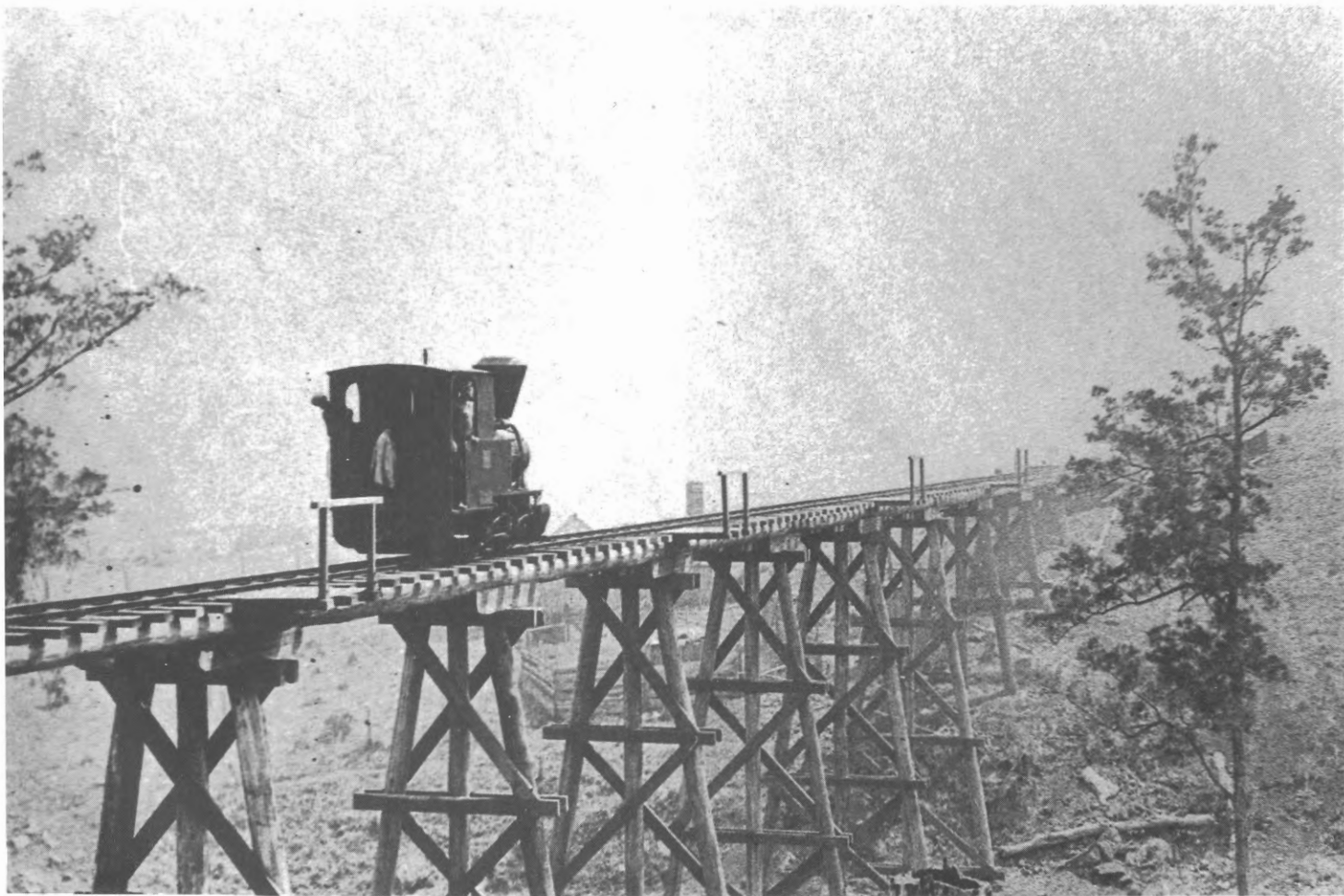
Trestle bridge over Smelter Creek, recently completed with the locomotive making a crossing. The photographer faces west. Although Cangai village is shrouded in mist, it is warm enough for the driver's jacket to be hung on the rear cab sheet. Could this be the trial run? Photo: Clarence River Historical Society Collection.
