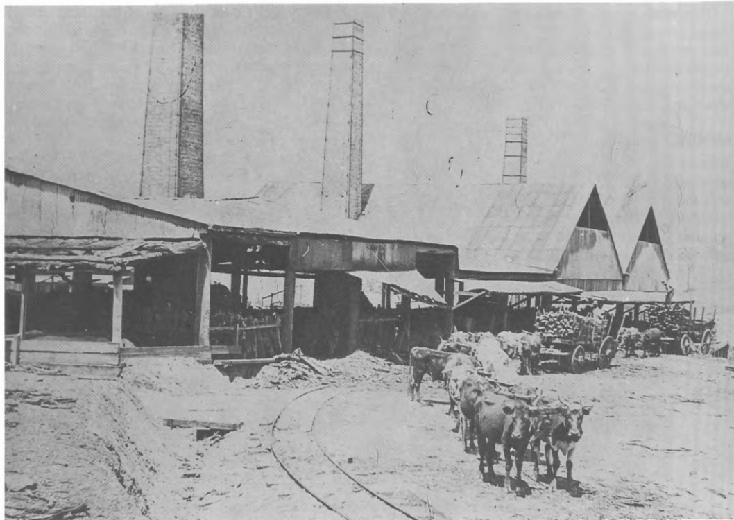
A closer view of furnaces 3, 2 and 1 at Cangai Smelter. Bullock teams are delivering firewood and, judging by the excavated earth, the rail track has not long been laid. Note the firewood billets stacked on end under cover, ready for firing. Photo: Clarence River Historical Society Collection.
