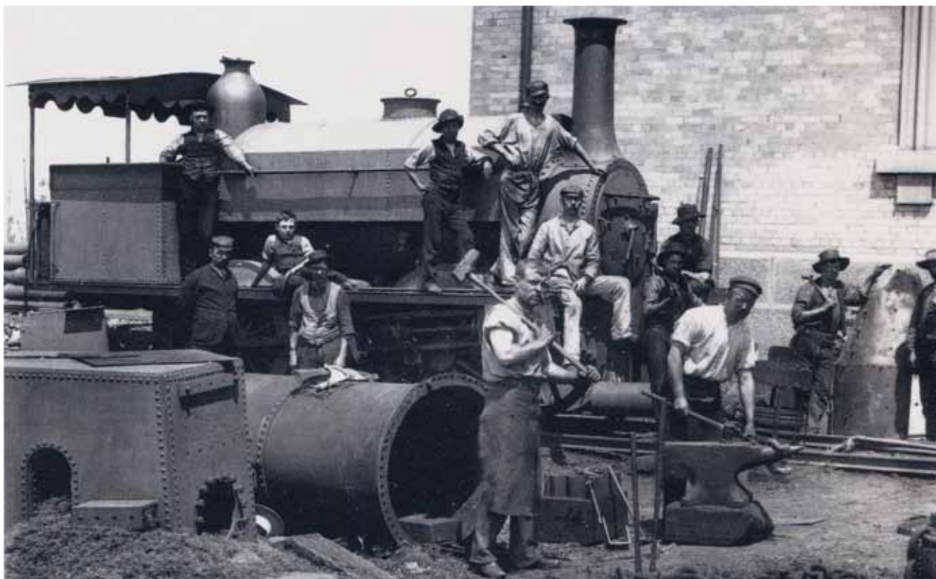
In 1877, workers at Morison and Bearby's engineering works at Carrington gather around one of the Newcastle Coal and Copper Company's Neilson 0-4-0ST locomotives, in the works for overhaul. The building in the background is the Carrington Hydraulic Power Station, which is still standing and currently heritage-listed. Photo: Ralph Snowball, Newcastle Regional Library
