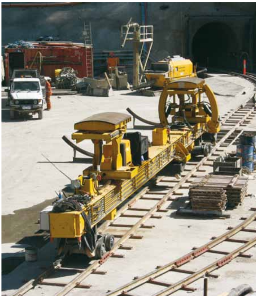
Outside the new Bogong high-pressure tunnel on 30 March is the Muhlhauser bogie pipe carrier, which was used for carrying and placing the 12m long steel liner sections into the tunnel. When loaded, there is not much to be seen except pipe!
