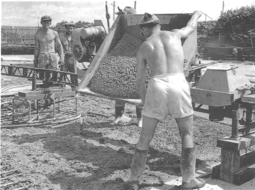
Unloading concrete from a monorail wagon, Allawah Reservoir
