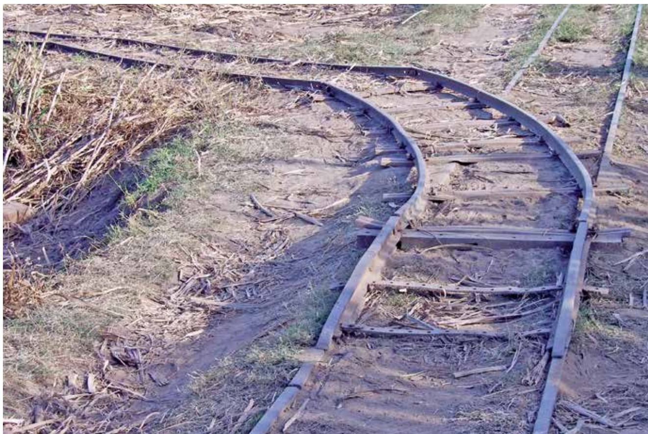
Assembagus Mill, Java: a short inclined plane, followed by a section of tight radius curved track leading into a field from the permanent way. In Queensland, these were known as 'riding points'. It's impossible to tell from the photo, but the permanent way probably incorporates some timber sleepers and is ballasted with dirt claimed from the area beside the track.
