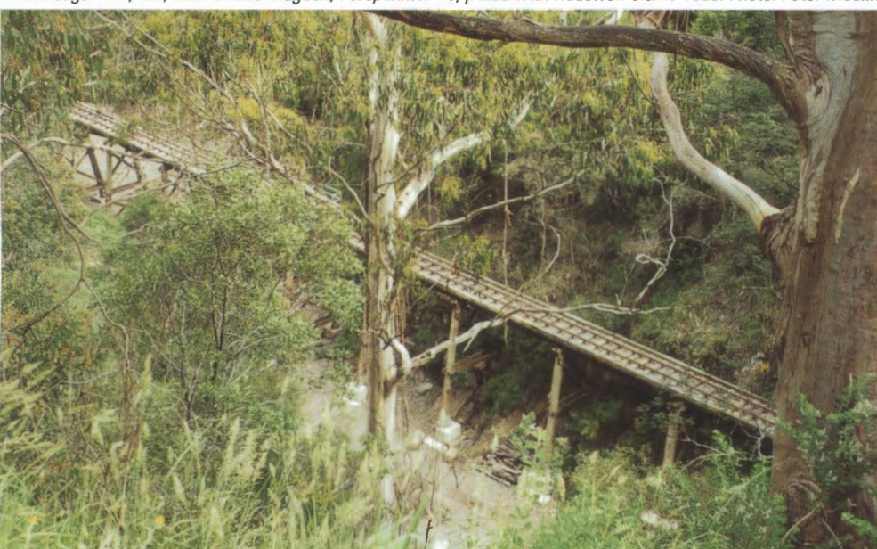
Walhalla Goldfields Railway, Vic: Bridge 6, newly restored (to its original style, as a 'fish belly' bridge), seen from the road on the opposite side of the valley, 18 November 2000.
