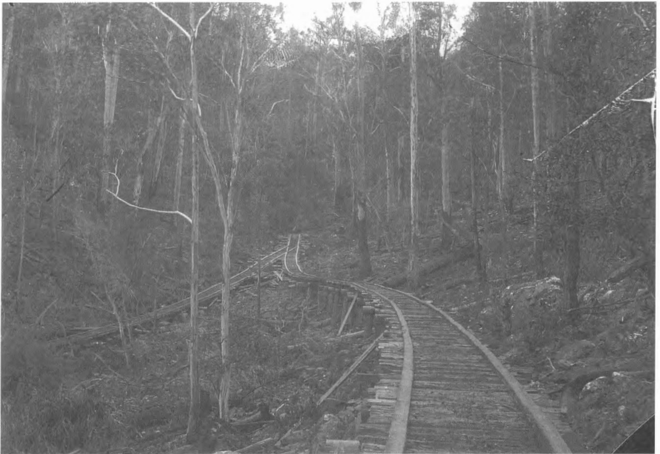
The 'Y' at the 12-mile point. Gradients were 1 in 14 on the right and 1 in 11 on the left.
