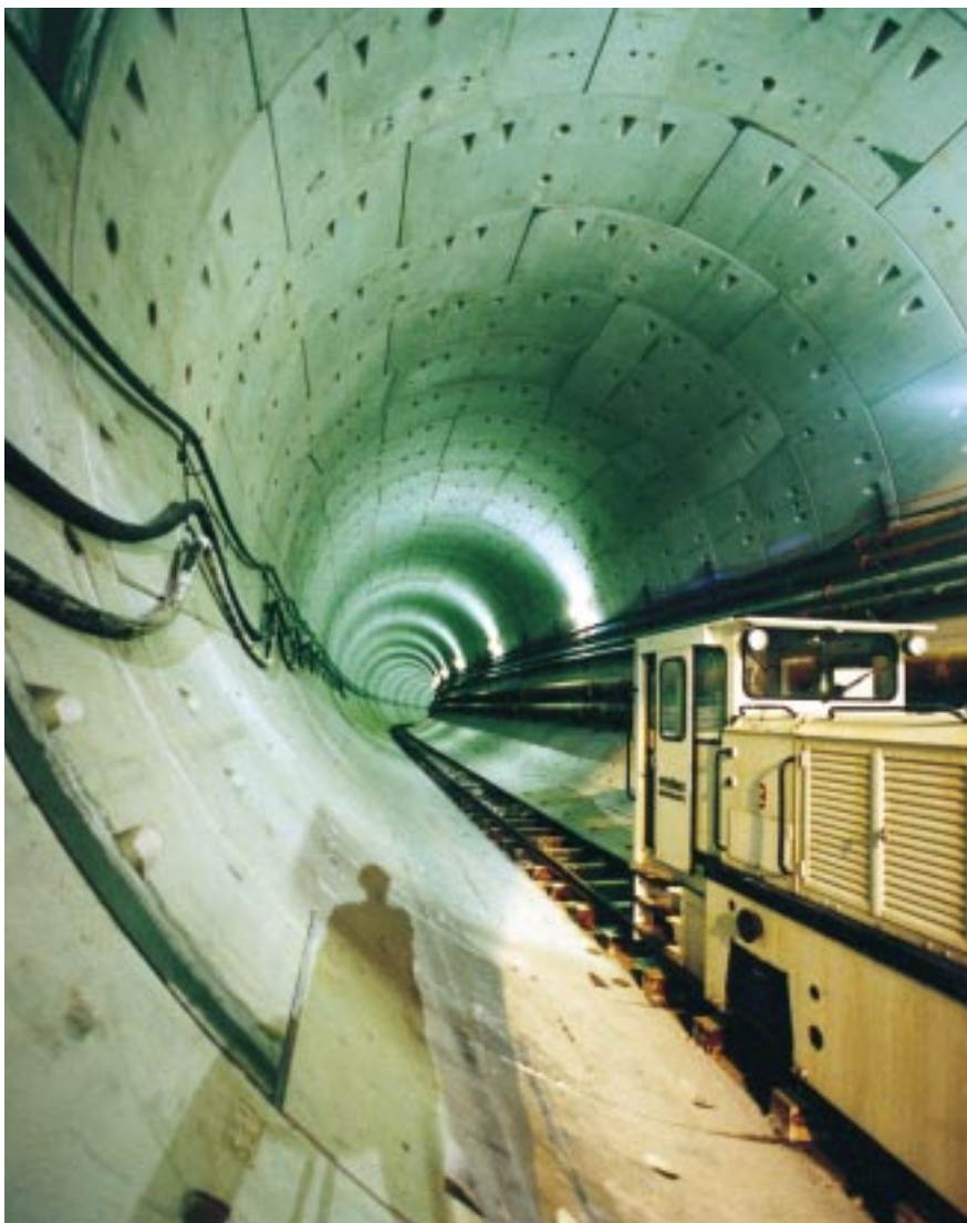
900mm gauge Schöma 4wDH 3 (4860 of 1985) in the Airport Link Tunnel.
