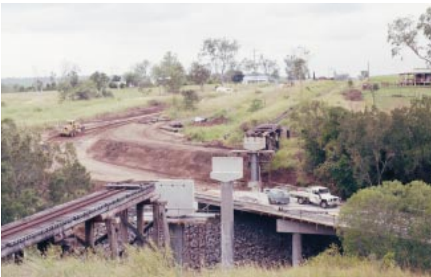
Bingera Mill's Currajong Creek bridge at Wallaville (see LR 141): the main timber and steel sections have been removed and new concrete piers installed, while a new road bridge is under construction below, 2 April 1998. Photo: John Browning
