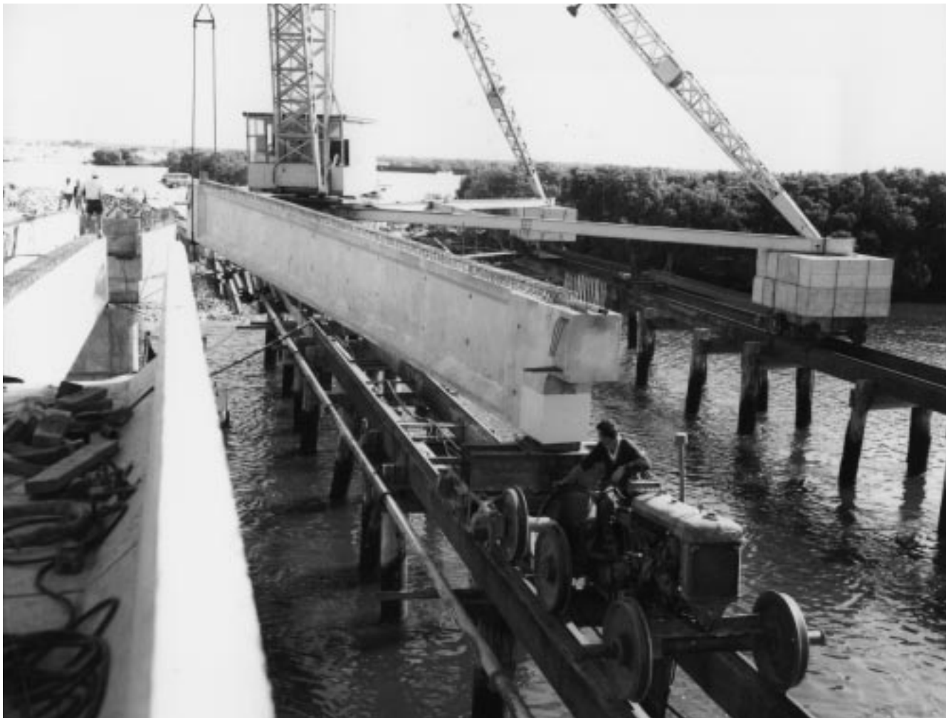
The Fordson rail tractor has just propelled a 30 ton bridge beam into place for the Garden Island to Torrens Island bridge on the Port River. Photos courtesy ESTA, A Lockyer Collection.
