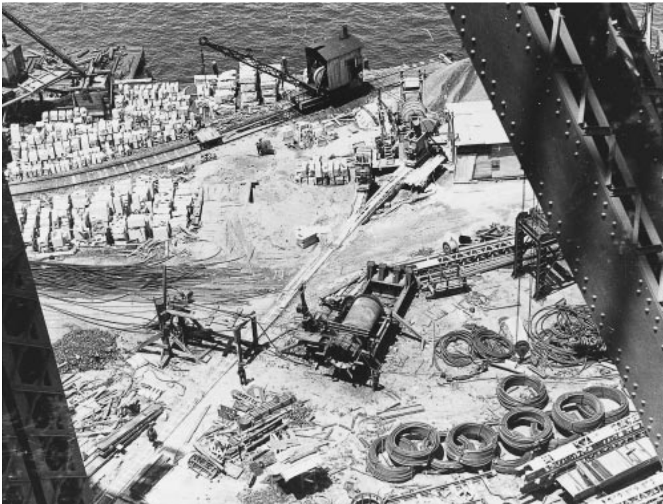
A fascinating variety of light railway operations is in view as the erection cables used in the Sydney Harbour Bridge construction are coiled for shipment and reuse elsewhere. December 18th 1930. Photo: Archives Office of NSW (The Rocks Branch) courtesy Jim Longworth
