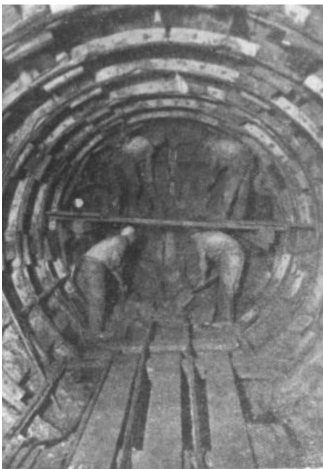
Working at the shield face in the Stony Creek tunnel, 1930. The left hand 16-inch gauge track is intact on the tunnel floor, but the right hand rail on the right track is absent.
