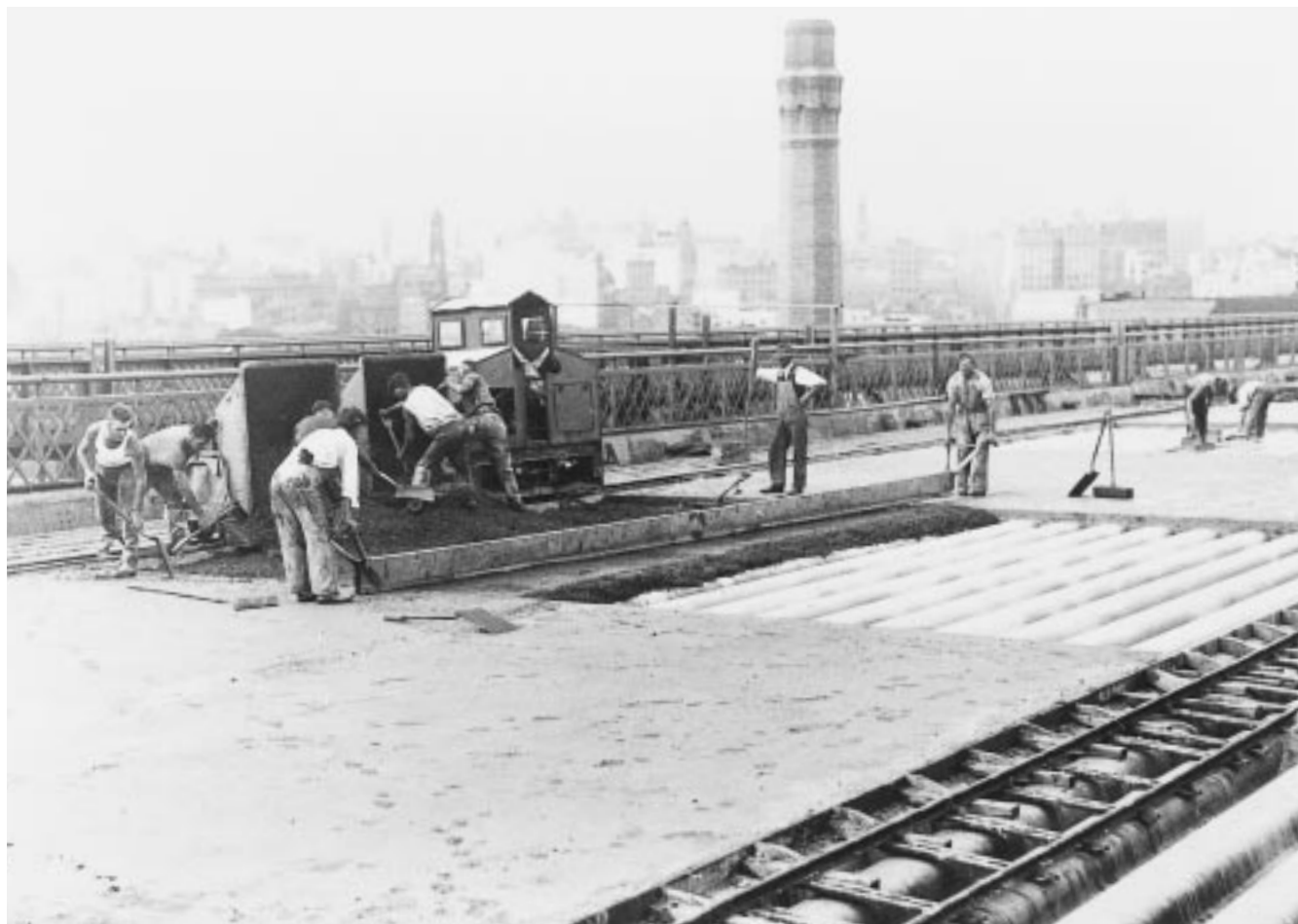
This scene is a reminder of the job creation benefits of the Sydney Harbour Bridge construction during the misery of the Great Depression. The laying of the coke concrete on the bridge decking is very much a manual job as the City of Sydney forms the backdrop for the Crossley locomotive and its train of two skips. March 20th 1931. Photo: Archives Office of NSW (The Rocks Branch) courtesy Jim Longworth
