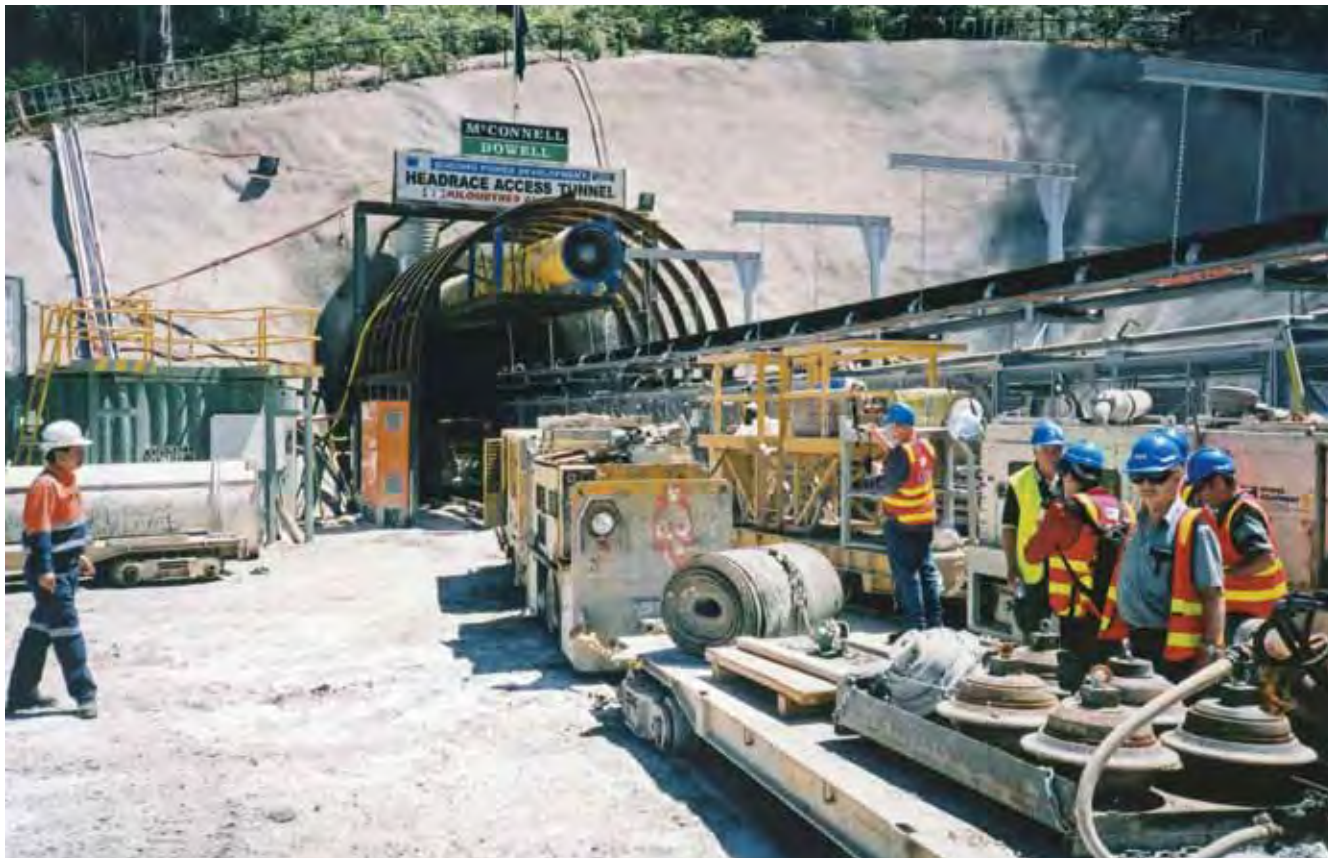
A view of the tunnel entrance. The flat car in the foreground has several cutters from the TBM. The locomotive centre is the Clayton and the white one on the right is the Plymouth. Photo: Simon Moorhead
