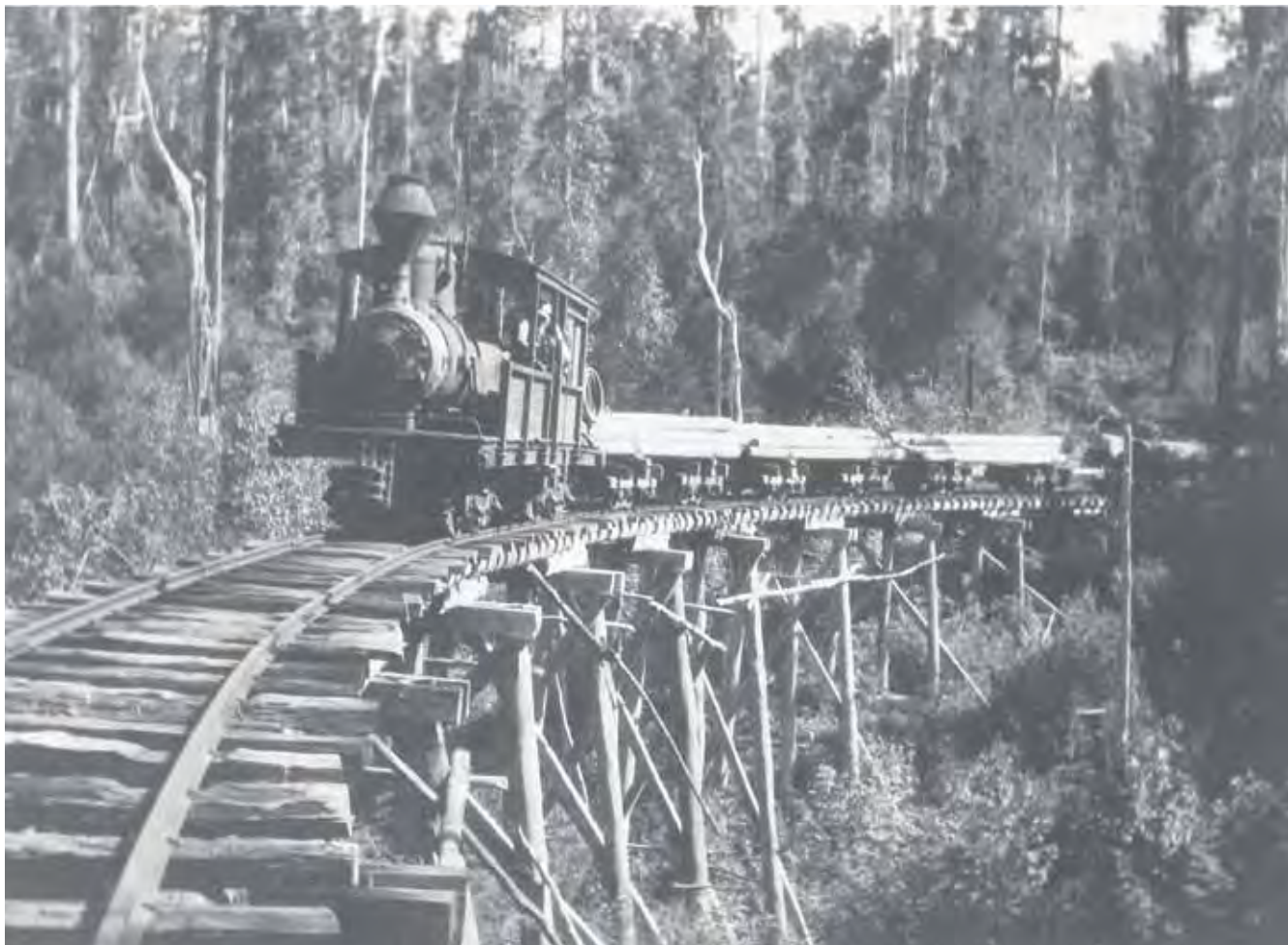
A-class Climax locomotive 'Corry-Pa' (1676 of 1926) on one of the large trestle bridges near the Gap. As the Wootton Tramway was extended towards the headwaters of Horses Creek, trestle bridges became bigger and higher. The larger bridges were a headache during bushfire weather, and required more maintenance. After a 1929 bridge derailment involving 'Corry-Pa', check rails were installed on the larger bridges.
