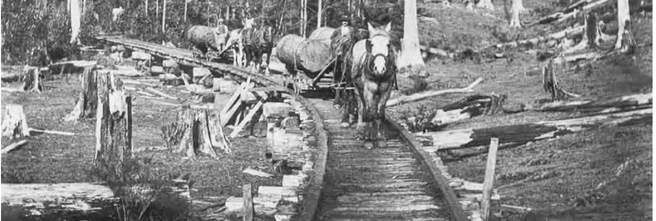
An early example of two horse-drawn log trains on fully-decked sawn timber track, thought to be crossing a bridge over Rileys Creek on one of the 4ft gauge lines of the Liverpool & Honeywood Tramroad Co. The whole length of track visible is elevated on pigsty piers, and the relatively easy curvature has allowed some springing of the rails, and thus kept the degree of faceting to a minimum. Compared with many timber-railed systems, this is therefore of a relatively high standard. The pigsty piers are shown in some detail in the inset photo, and the wheels, although wider than railway profile, are not as wide as the later spar wheels. The two photographs were taken of the same pose. Photos: unknown c1880
