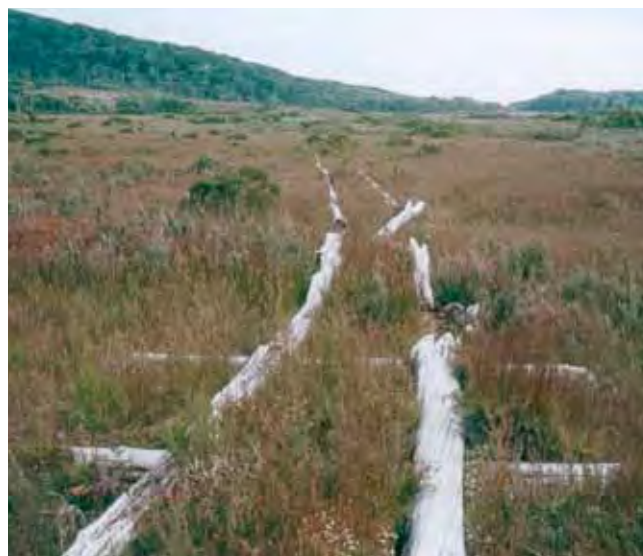
This photograph, dating from c1975, shows a section of abandoned tramway running southwards from Cockle Creek along the Blowhole Valley. It gives a good idea of the crudeness of spar track, particularly of the irregularity of the spars themselves, of the discontinuities in the track, and of the wide spacing of the bed-log sleepers. Photo: Wayne Chenoweth
