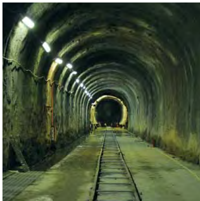
Inside the drill and blast tunnel with the rail laid on grade; later this rail was lifted, the invert cleaned, blinding concrete placed and the rail re-laid.
