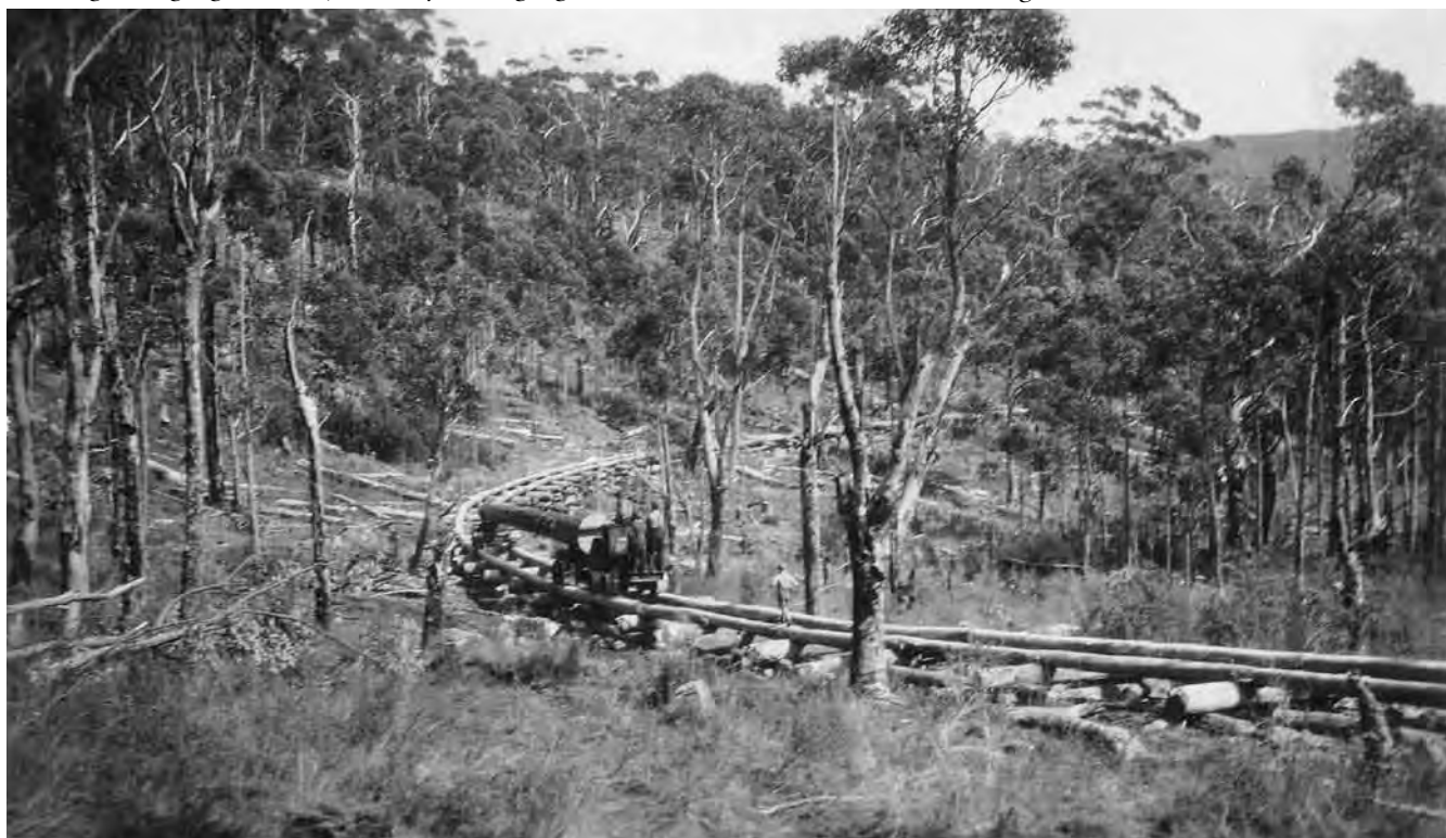
Another example of spar track, this time carrying a tractor locomotive with a driven log-bogie propelling a very long log along an elevated pigsty section. It is on the remarkable Pebbly Bight line out of George Heather's Cockle Creek Mill, a line that was built by George, two teenage daughters and two younger sons in five months at the end of World War II. The open nature of the construction would certainly not have suited horses, but note the confidence of the person walking along the spars behind the unit. Photo courtesy Jean Burgess (nee Heather), one of those daughters
