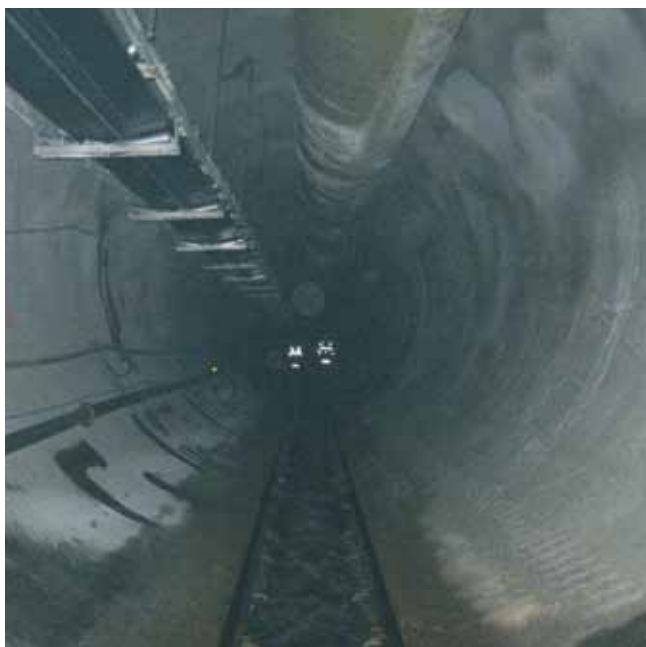
Inside the TBM tunnel where the profile is circular due to the cutting of the TBM. The sleepers are curved for this purpose.
