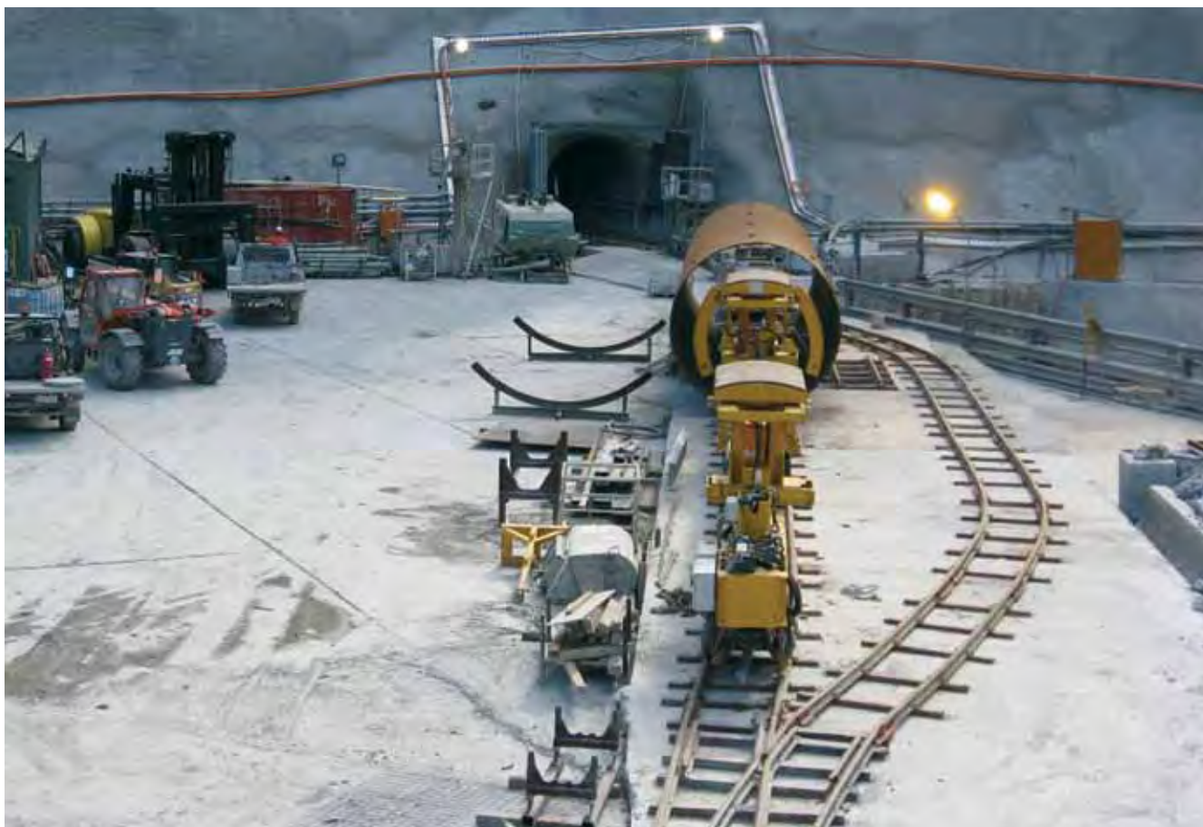
The Muhlhauser bogie pipe carrier used for transporting the 12m long steel liner sections into the tunnel, seen outside the new Bogong high-pressure tunnel on 30 March 2009.
