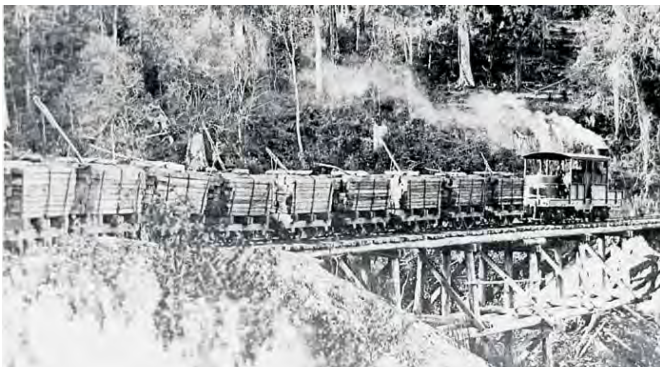
A-class Climax Aleda (1297 of 1913) at the head of a sleeper train in the Wootton forests. The lightweight Aleda could pull a heavy load but was slow, averaging only 5 mph on the trip to Mayer's Point with loaded trains.
