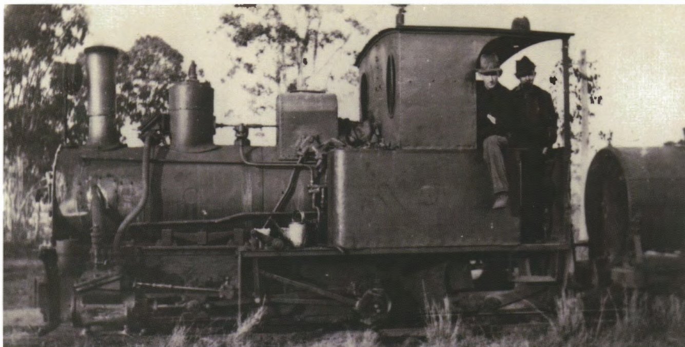
Bunyip has received further modifications but its final rebuild is yet to come. Note the changes to the boiler mountings. Photographed at Tookie (near Gin Gin) in August 1941.
