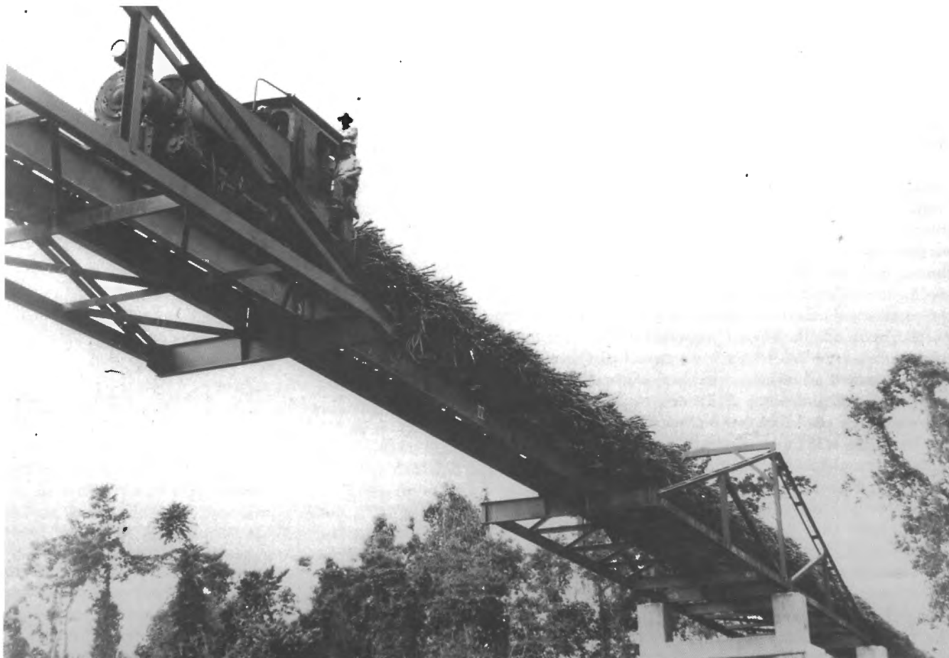
The Liverpool Creek bridge at Silkwood was a spectacular crossing. The old low-level timber bridge was replaced in 1953 with a 123.5 metre structure featuring a pair of cantilevered trusses with a 13.7 metre central span between them. The total cantilevered span was 68 metres and there were also four 13.7 metre individual girder spans. John Fowler 0-4-2T No.10 (17881 of 1928), with the author on board, as fireman, heads away from Silkwood with the first loaded train over the new bridge.
