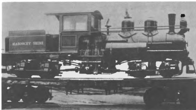
New Lima Class 'A' Shay 2823 of 1915 sits on a flatcar awaiting shipment to the docks, then a long sea journey to far-off Australia. Photo: LRRSA archives
