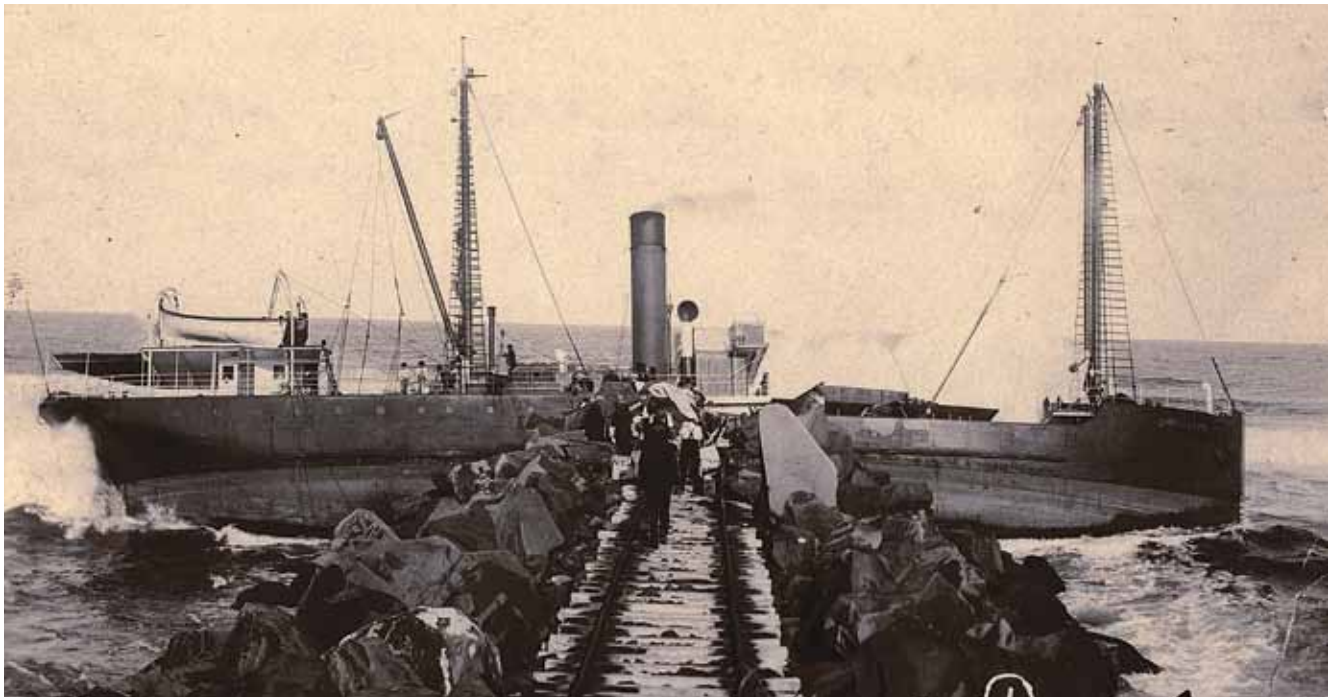
While attempting to enter the Manning River during heavy weather in April 1910, the two-month old NCSNC steamer Minimbar was swept onto the end of the breakwater and broke her back. All passengers and crew were saved but the vessel was a total wreck.
