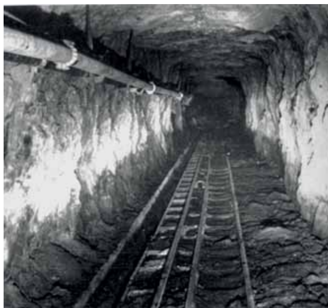
Looking north along the 1480 level in the British-Junction section, not far from Browne shaft. 2ft gauge track was laid along the drive for 2¾ miles from No.7 shaft, but a third rail of 15-in gauge was necessary from Browne shaft to the point of breakthrough so as to carry the 11 cubic feet box trucks, which were the largest size that could enter that shaft's small gate. Photo: Author's collection
