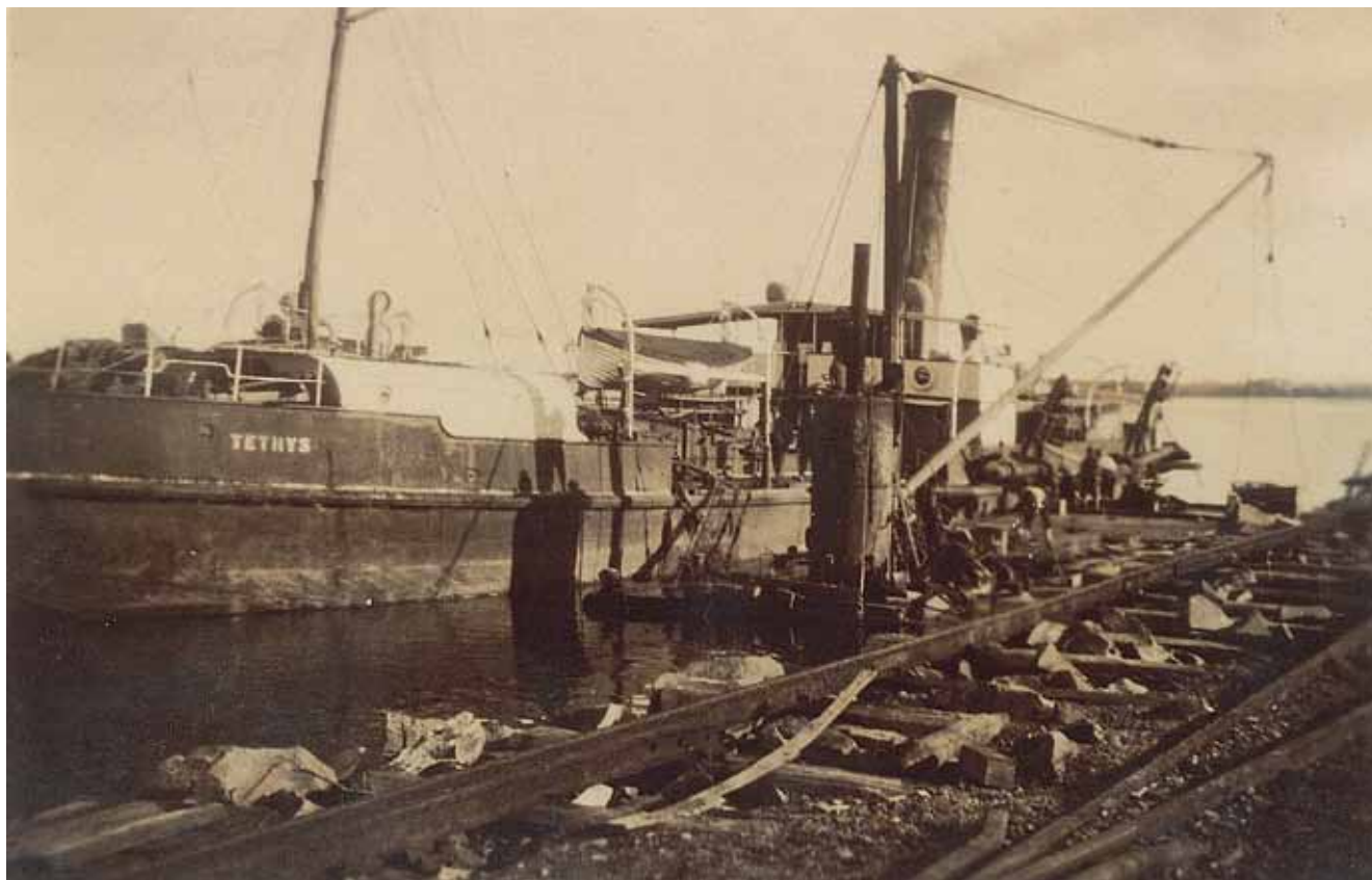
The PWD sand-pump bar-dredge Tethys moored at the public wharf alongside the northern training wall. The Tethys was one of two modern dredges built specially for work on the outer sand bars of coastal rivers, but it was no match for the capricious Manning River.
