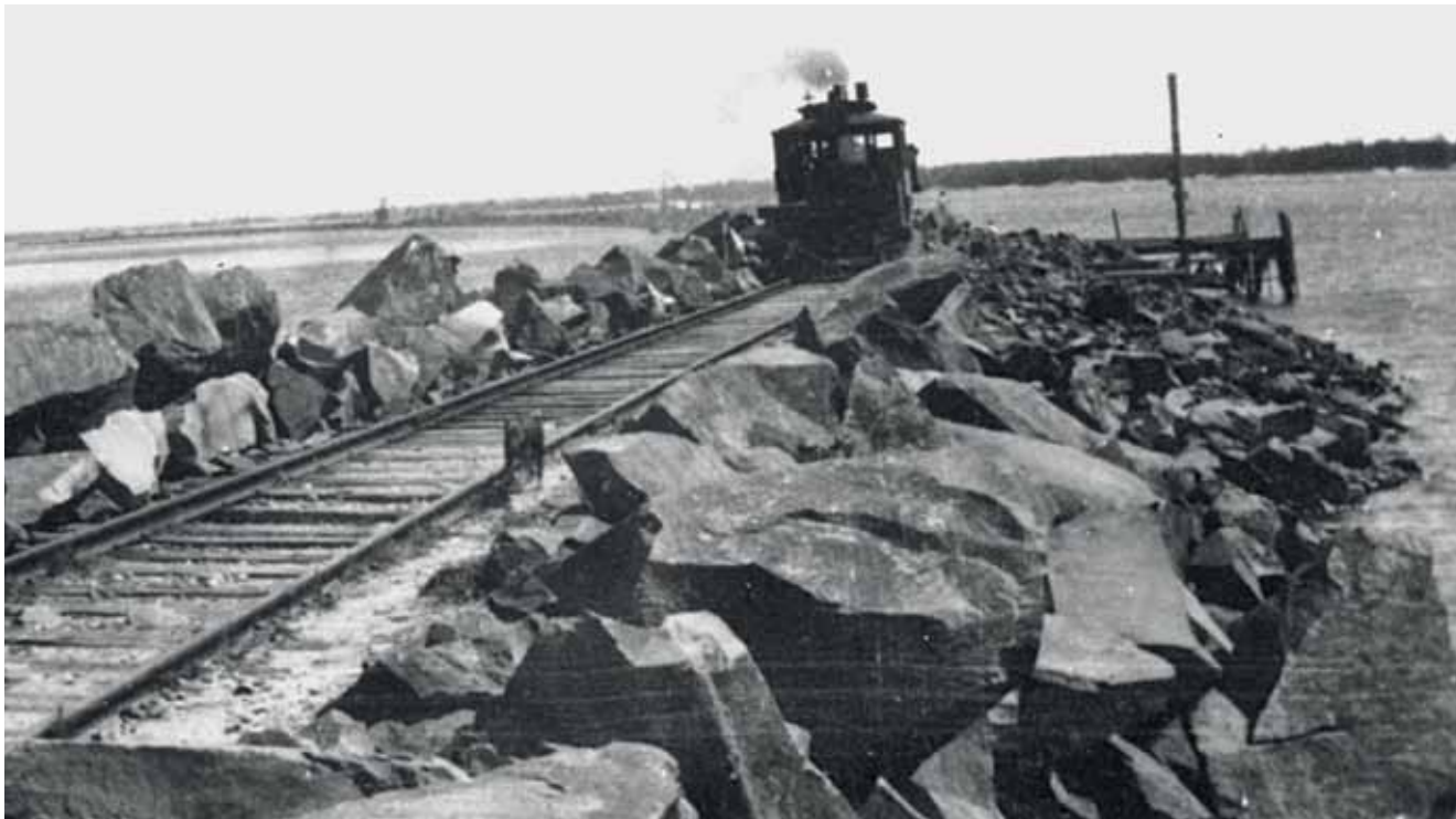
Steam Tram Motor 33 at work on the Manning River Training Wall in the 1920s. Just visible in the left background is the crane wharf where rail trucks of stone destined for the south spur wall will be lifted into punts to be taken across the river.
