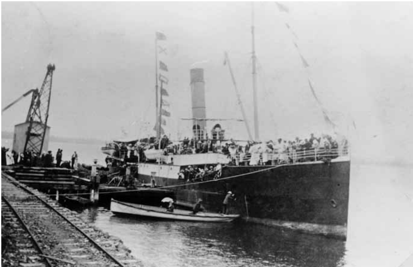
For many years the SS Electra was the regular coastal steamer on the Sydney to Manning River run. It is seen here alongside the crane wharf on the river's northern training wall. This wharf was equipped with a 20-ton capacity steam crane designed to load heavy boulders for the construction of the southern breakwater wall which, though started, was never finished. Photo: Manning District Historical Society Collection
