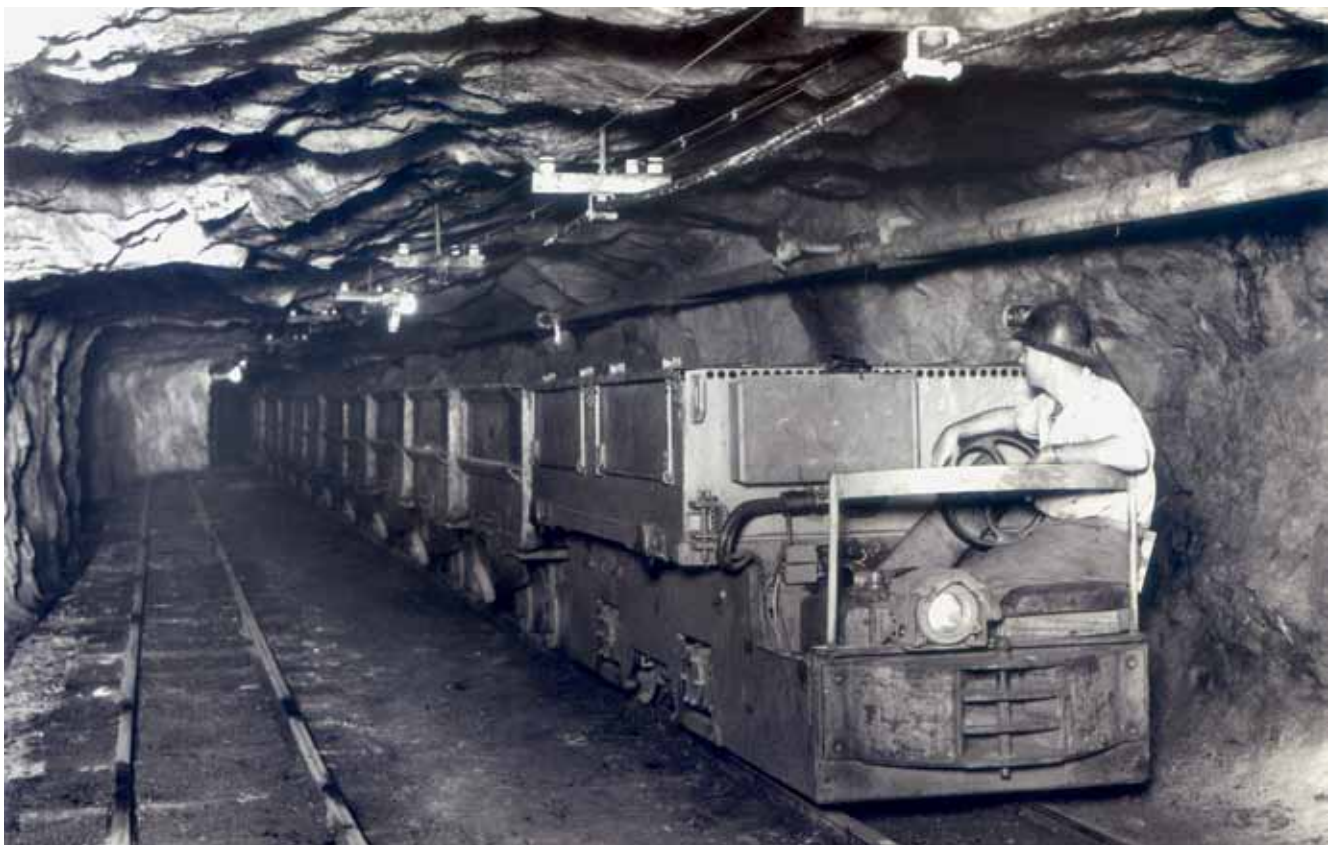
A 24-in gauge Goodman storage battery locomotive on a rake of Granby cars underground at the South mine. The 'mule driver' has his right hand draped around the brake hand wheel. This 8 ton, 38hp American built locomotive worked the subterranean mainline drives and crosscuts of the mine.
