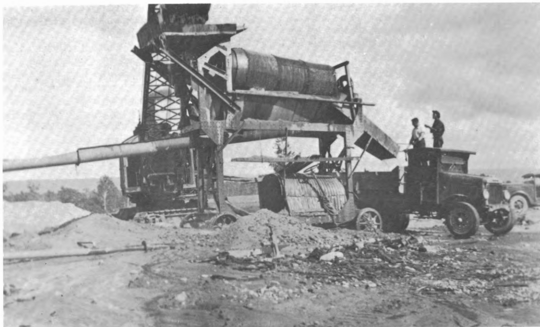
On the Island, circa 1940, one of the Camasanees , now converted from rail, loads Cleary Bros lorries. Under the chute is a Model 54 International with Stan Davis and Stan Smart on top, while behind is Len McLeod's International 63. The Marion, loading here, had received a new 70ft. boom and a 1¾ yard bucket. Photo: D. Smart
