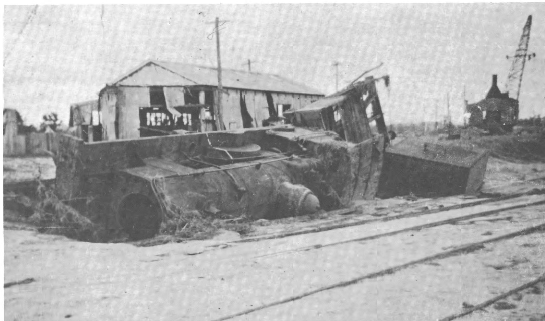
1630 overturned after being undercut by flood waters in 1956. The workshop behind it had been given a pointed end to minimise flood damage. However, trees cut down in the construction of the Warragamba Dam were carried downstream and punched holes in the walls. Photo: D. Clemson
