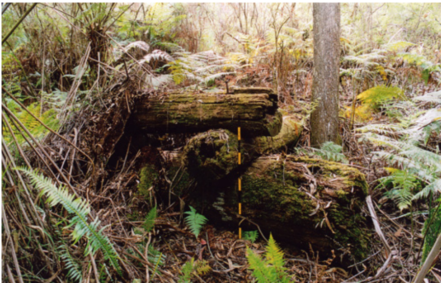
The abutment of a crib log bridge along the lower section of Cameron & Barton's tramway. Photo: Peter Evans, 9 December 2012
