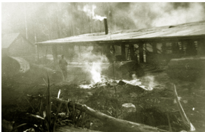
Cameron & Barton's mill alongside Keppel Creek in 1937.
