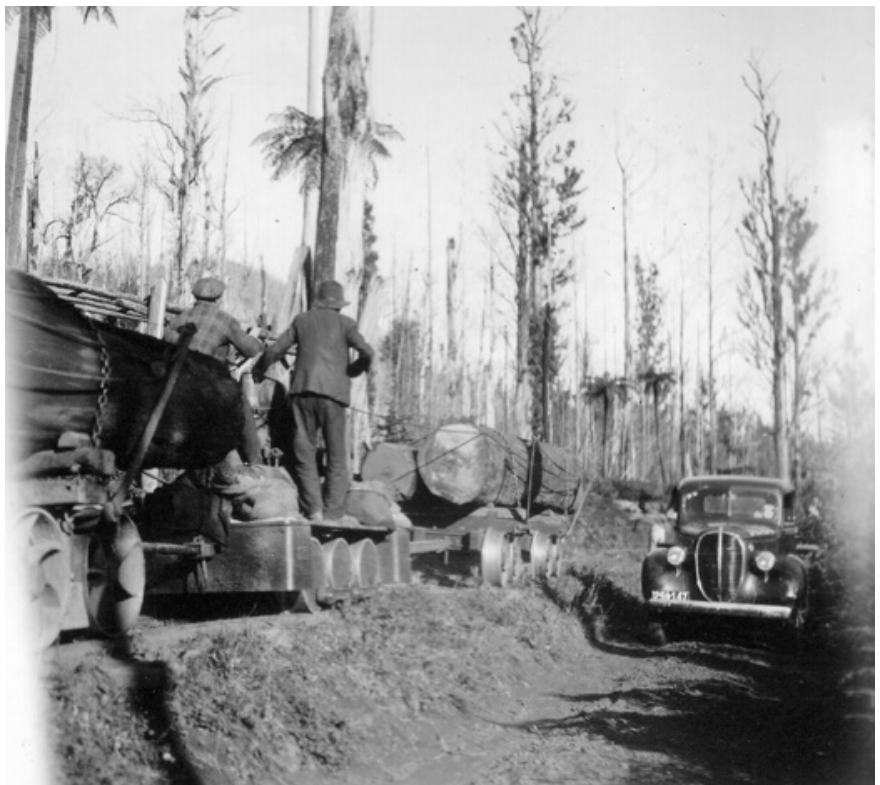
In early May 1941, Johnson visited the Granton Mill tramway, north of Healesville, Vic. In this image the 6w Days rail tractor, powered by a McCormack Deering engine, is seen in its usual position with 'two logs behind, one in front'. It managed one or two return trips a day from Granton Mill to the road landing, where logs were transferred to trucks. The line ran east beyond the Granton Mill to Granton Dindi Mill, which had been burned out in the 1939 fires. At the time of his visit, Johnson reported that the tramway and Granton Dindi Mill were being rebuilt and expected to recommence operation in the spring.
