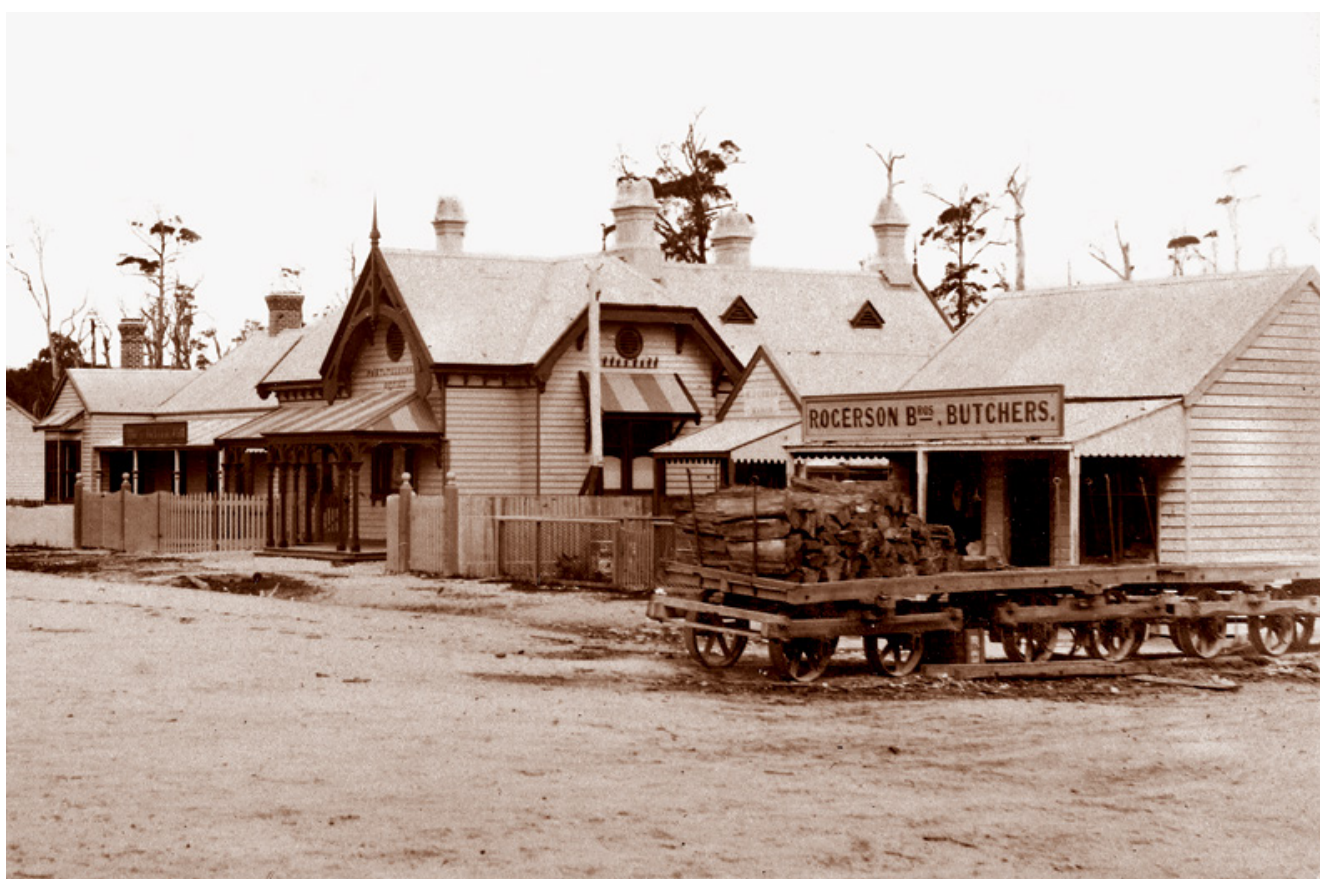
The only known photograph showing the trucks used on the Stockyard Creek Tramway. This view depicts the Main Street corner opposite Thornley's hotel c1888. The light framing of the trucks was adequate for the freight and passengers transported. Benches were placed on board when people were carried.
