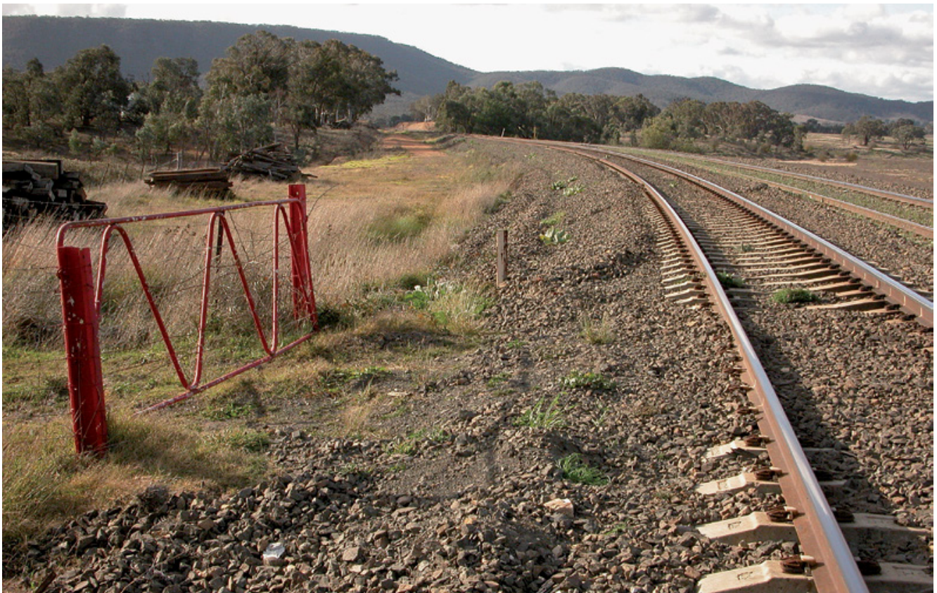
A recent view of the site of Mannafields Station on the Great Southern Railway, north of Goulburn. The view shows the double main line looking in the up direction, toward Sydney, and the single platform would have been on the left or 'up' side of the line. This is possibly where the tramway of the Cookbundoon Slate Company terminated, under its authorising Act of 1881, and is currently being further researched. Photo: Leon Oberg
