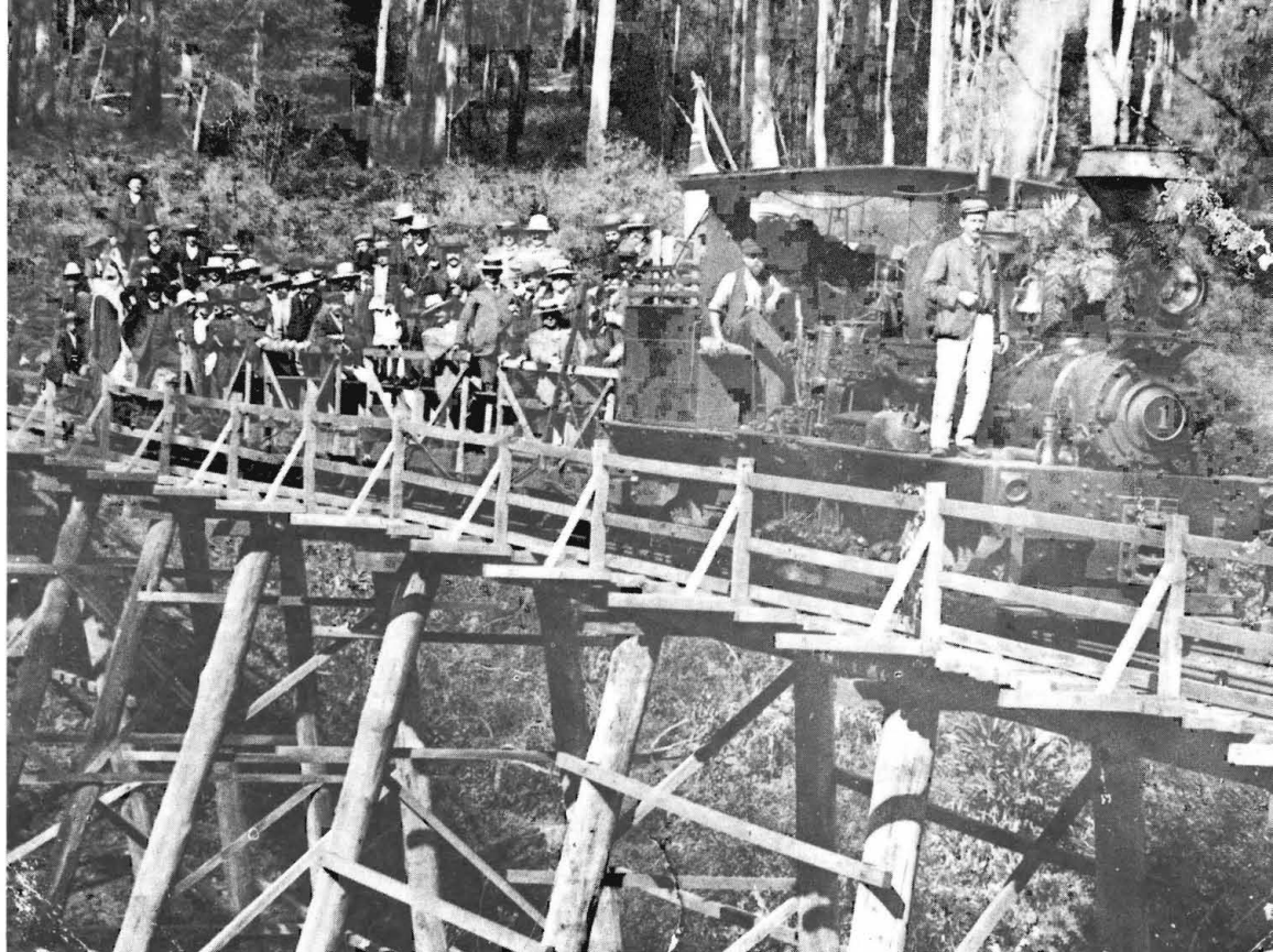
A special passenger train, possibly on the occasion of the visit of Mr H. P. Somerset in 1910; or the visit of Lord Lamington, Governor of Queensland. Note the timber bogies modified to carry passengers.
