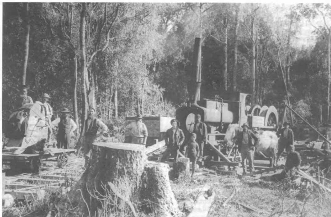
Andrew Barclay 0-4-OST locomotive with hauling gear on William Brownlee & Sons tramway, Havelock, New Zealand. Photo: NZ Forest Service
