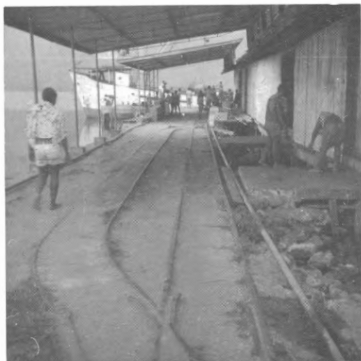
Soraken tramway, Bougainville: Passing loop on the wharf causeway. Photo: M Pearson
