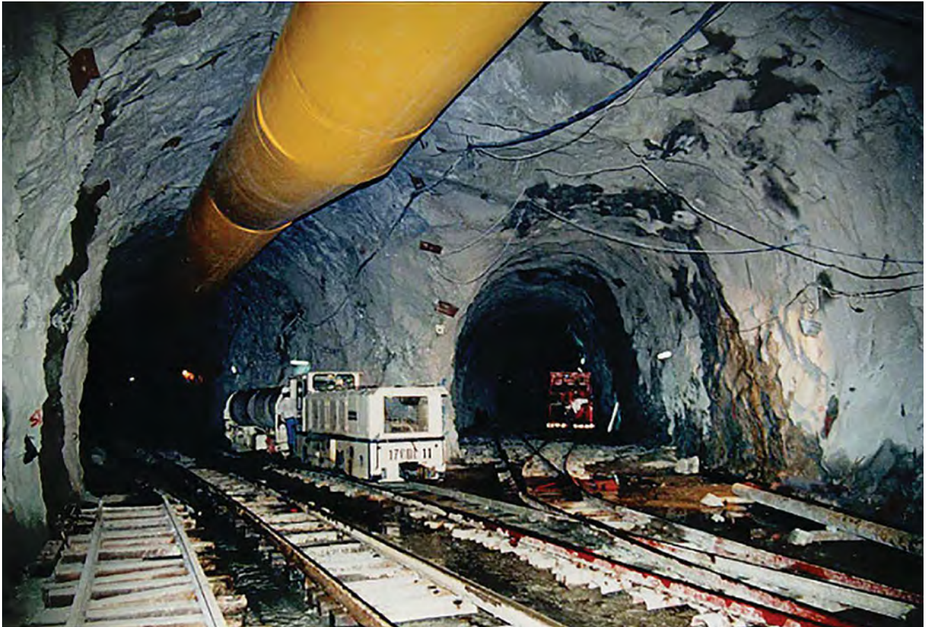
Deep in the Singkarak Hydro Electric Power Project power station caverns in Sumatra, access to the construction of a 16.5 km long headrace pressure tunnel is serviced by #176DL-11 (Schöma 5286 of 1992), one of ten Model Type CFL180DCL of which three will be destined for further service in Perth, WA. Photo: The late Ray Gardiner Collection
