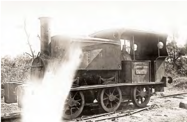
Above: No. 18 later as NSWGR No. 29. The funnel has been extended upwards, probably to reduce smoke from entering the trailing passenger carriages, leaving the number 29 in a broad shallow groove at about half-height Below: No. 18 with its connecting rods on the ground. Photo: Author's collection Bottom: No. 18, still retaining the faded 'N° 18', derelict in the Newcastle area on an unknown date. Photo: J L N Southern
