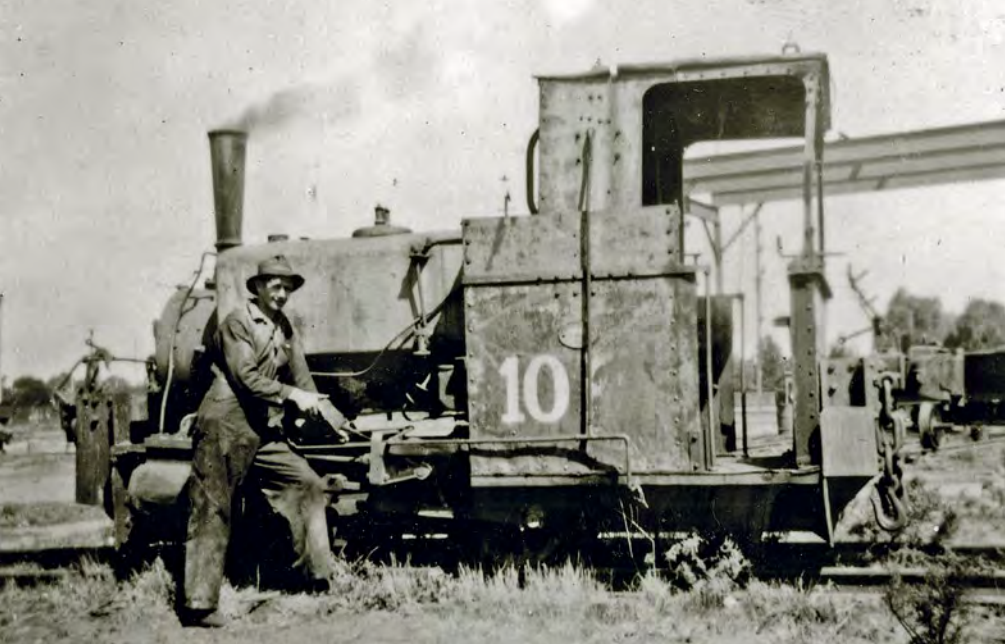
Locomotive No. 10 at Whyalla in 1951. It had been withdrawn around 1945, and this was actually a posed photo with burning rubber tyres in the smokebox to give the smoke effect. No. 10 was built by Baguley (B/N 2525/1922), and the enclosed cab and funnel came from 1 st No. 9 (Arnold Jung B/N 680/1903) at Whyalla. Photo: David Griffiths collection.
