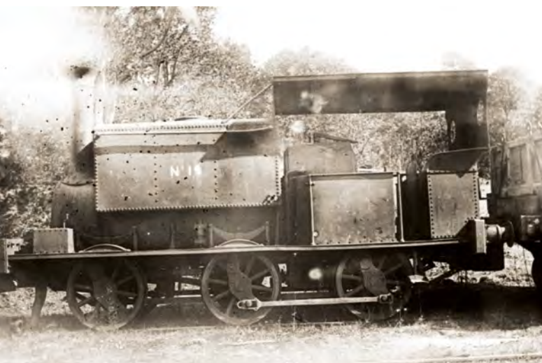
Below left: No. 19, retaining the faded 'No. 19', after conversion into a 2-4-0, date unknown. Photo: Author's collection Below right: Close up of No. 20 as an 0-4-4 saddle tank hauling small sized rock in the Angourie quarry, date unknown. Photo: Author's collection
