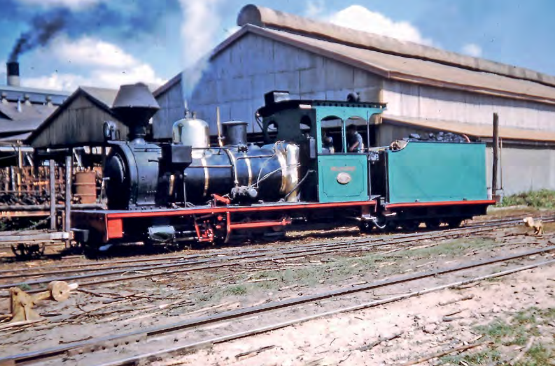
Hudswell Clarke 0-6-0 Melbourne in the empty yard at Victoria Mill in the nineteen fifties. The Melbourne was a 1956 combination of 1552, 1659 and 1701 and carried the builder's plates from 1701. Photo: P.G.Dow
