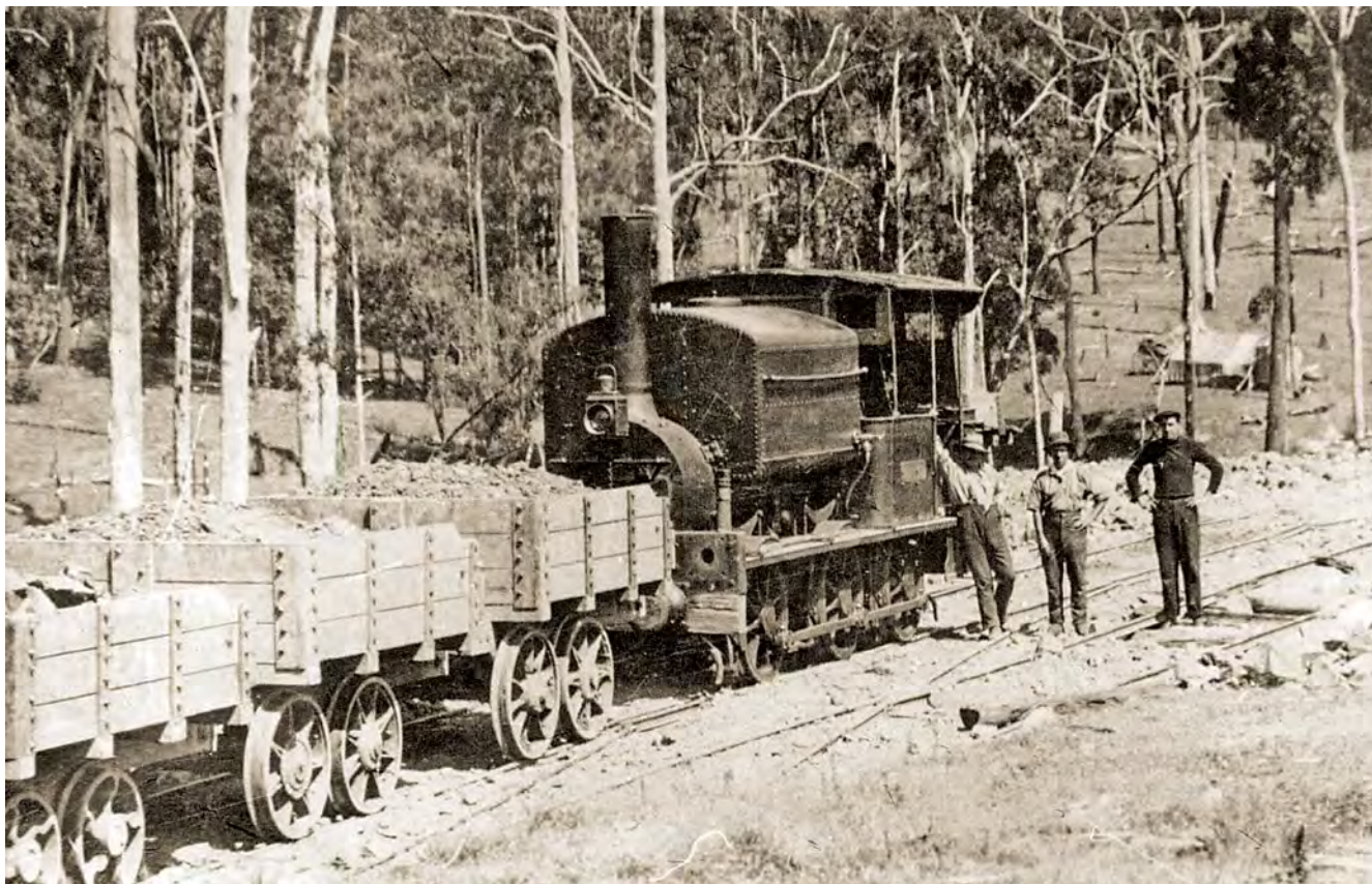
Above: No. 15 at work on building the North Coast Railway at Stroud Hill in the Dungog region. The square window openings in the front spectacle plate and rear cabin screen are distinctive. Photo: HWright collection Below left: No. 15 later as NSWGR 394x. Photo: ARHSnsw RRC 009877 Bottom left: PWD tram motor No. 16 at Harrington. The number '33' was the motor's original NSWGT number; not the PWD's number. Photo: GH Eardley collection
