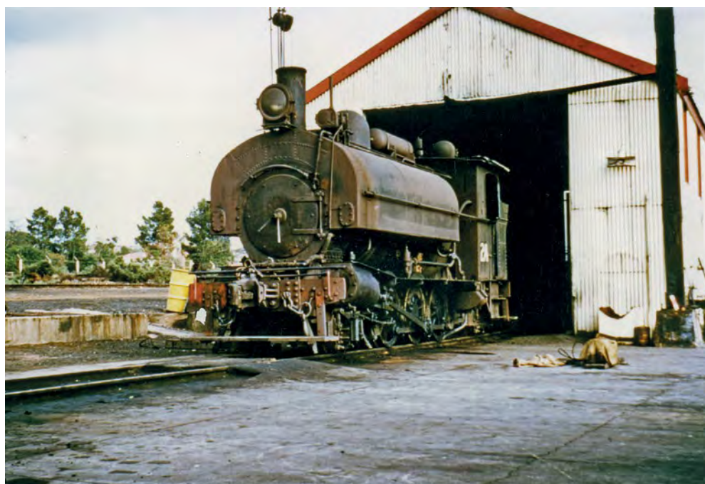
Locomotive 2A at the loco shed at Whyalla, probably c. 1960. This loco is another interesting BHP Whyalla hybrid. Apparently in the last several years of steam at Whyalla, the boiler and saddle tank from No. 1 (2-6-0ST Beyer, Peacock B/N 4723/1905) were fitted to the frame and running gear of side tank 2A (2-6-2T Beyer, Peacock B/N 5125/1908), resulting in this 2-6-2ST. Both locomotives were scrapped by late 1962. Photo: George Bishop collection
