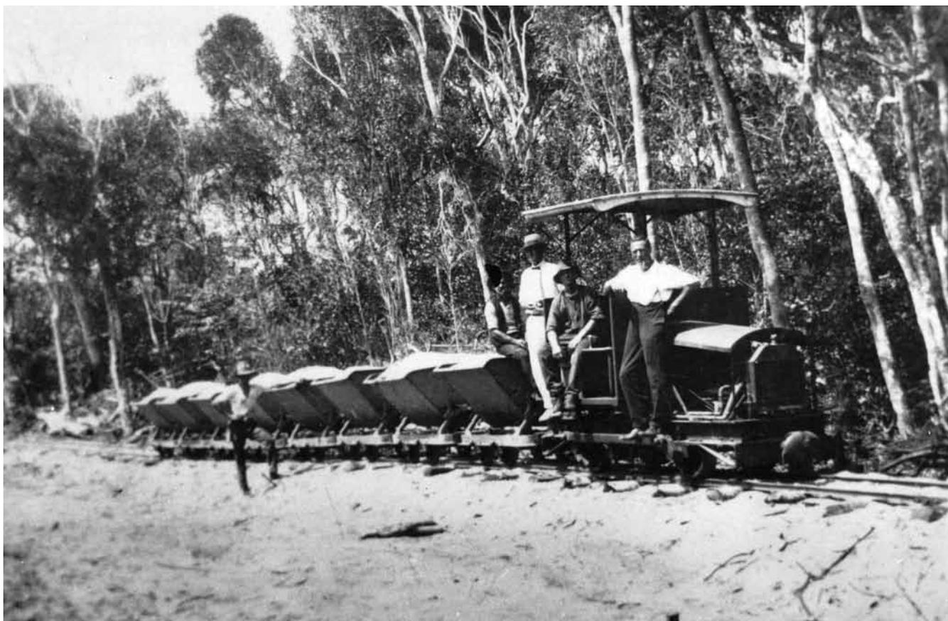
*This lovely posed photograph in a bushland setting where today bitumen, concrete and high rise dominate shows clearly the Model T front radiator on the petrol locomotive.*
