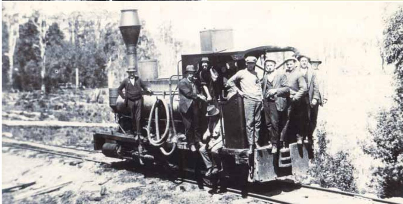
1 January 1923: Loco Cameron idle. This plant is very severe on the line. Wheel base too long consequently she knocks the line about considerably especially the curves. Haulage capacity limited, say 25 to 30 tons. In future to be used in case of emergency.
