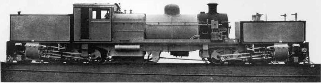
TRACTIVE POWER AT 75% BOILER PRESSURE 23,690 lbs. MAXIMUM AXLE LOAD 9.45 tons. 2' 6" GAUGE.
