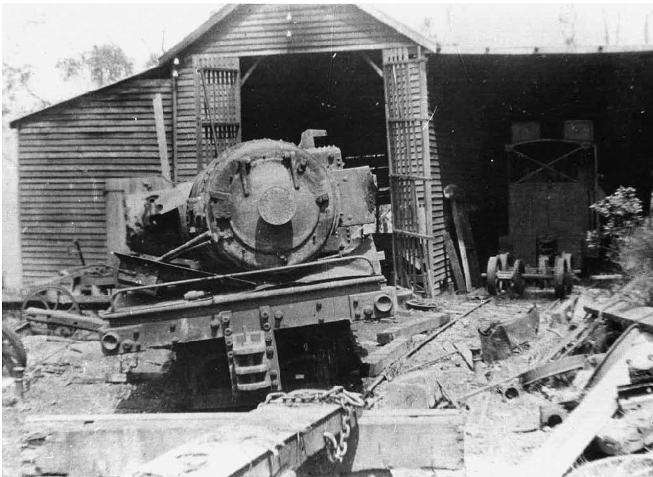
*'Corry-Pa' was dismantled at the wreck site and taken to Mayers Point for repairs. The steel frame was sent to Sydney to be straightened. This scene shows the wreck in front of the Mayers Point engine shed and the Andrew Barclay steam loco Cameron stored out of use but still serviceable.*
