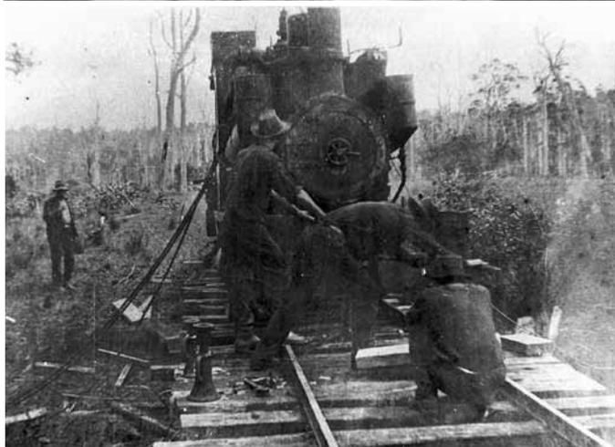
Cameron, Andrew Barclay 253 of 1882, ready to leave Wootton Depot with a mixed train of bridge girders and railway sleepers. With small 11 inch diameter cylinders and maximum boiler pressure of 125 psi, the loco's haulage capacity was limited to 30 odd tons, less than half that of the A-Class Climax Aleda. Photo: HB Moyle
