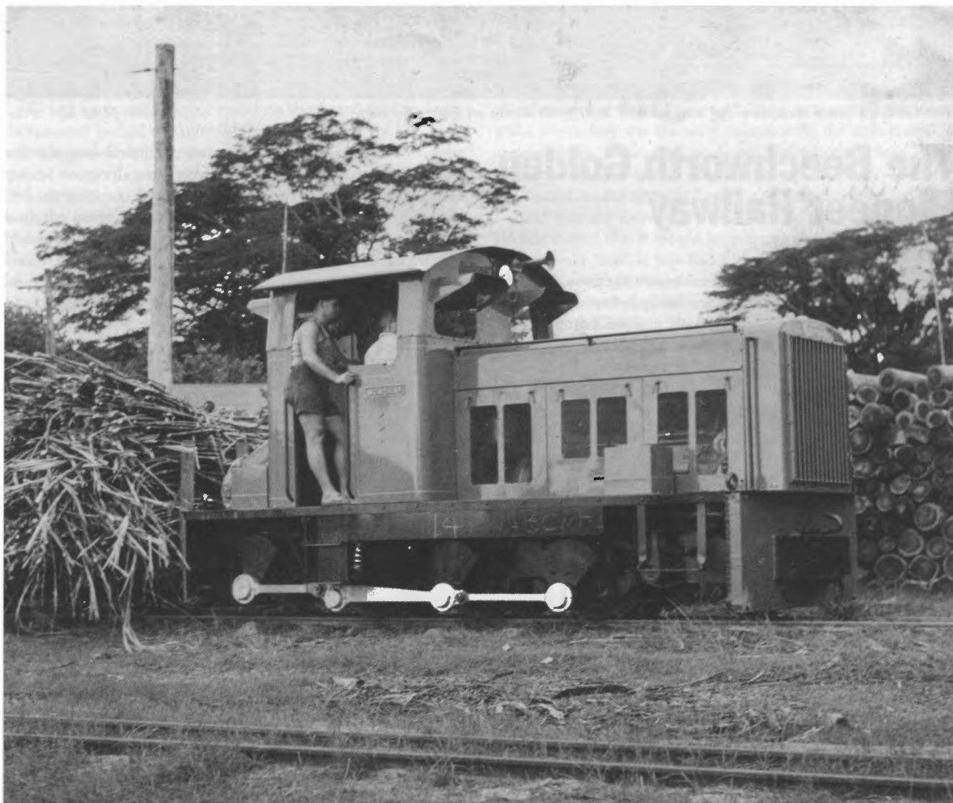
The photograph above, showing Com-Eng 0-6-0DM B1719 of 1957 hauling a load of wholestick cane, appeared in the pages of Railway Transportation magazine, with the caption 'First run for Com Eng diesel "Mowbray" at Mossman with a load of 42 cane trucks easily fulfilled the expectations of the Mill Manager who rode the loco with Com Eng service personnel'. It would appear that the manager was impressed, as over the following eight years Mossman Mill purchased a further four locomotives from Com Eng.
