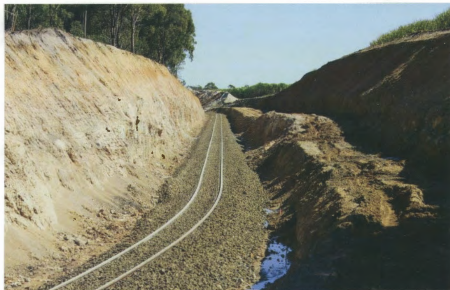
Substantial earthworks have been required to achieve satisfactory grades on the line linking the closed Fairymead Mill with Bingera Mill, and particularly so at Pitt's Hill, near Splitter's Creek, where a significant deviation has been built. The work was practically completed by mid-June 2008. Photo: Lincoln Driver
