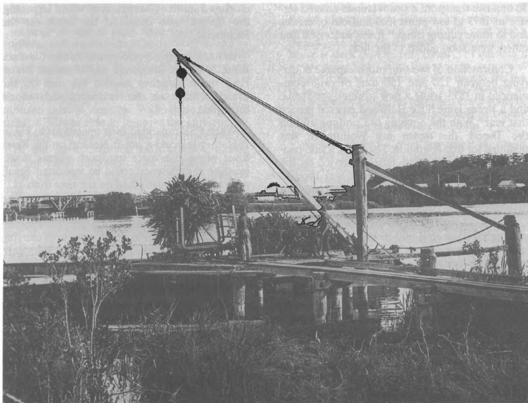
Short tramways from the farm to riverside jetty fed cane to the “river highways” of the northern NSW sugar mills. In this typical scene, a derrick loads cane from railway trucks into a punt on the river.
