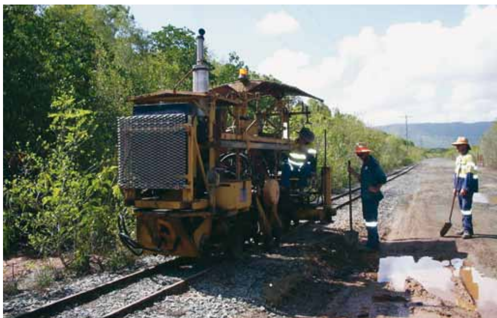
The Mossman Central Mill track crew in action with the track repair task on the Ballyhooley Steam Railway at Port Douglas in December 2009. Tamping machine is Mossman's Plasser Model KMX-06 111 of 1976. Photo: Peter Lloyd
