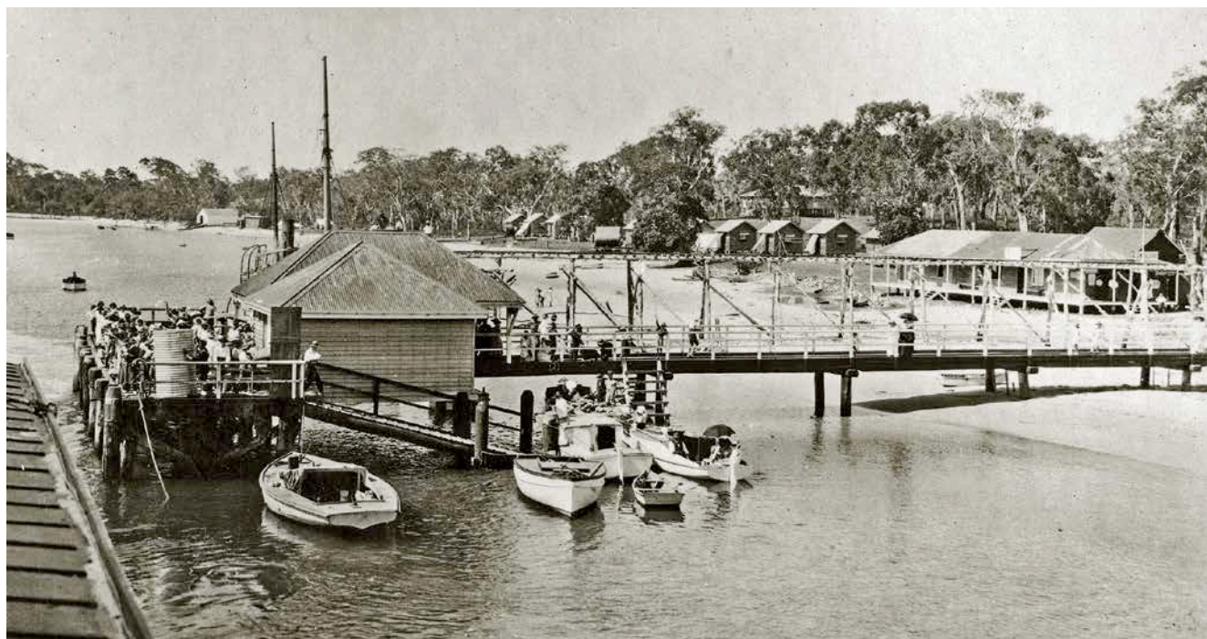
Arriving at the Bongaree jetty; taken from the promenade deck of the ss Doomba, March or April 1924. The temporary staging, to facilitate the import of stone and gravel for construction of the company’s private road, is clearly seen – with one skip visible – beyond the passenger jetty. The ss Porpoise is largely hidden behind the jetty shelter shed. Three men and the top of the skip being filled, can just be seen above the roofline. Compare with photo on next page. The row of huts in the background were built by the Brisbane Tug Company and often referred to as the ‘Twelve Apostles’. Photo: APA-114/2 Campbell Family Photograph Albums, John Oxley Library, State Library of Queensland
