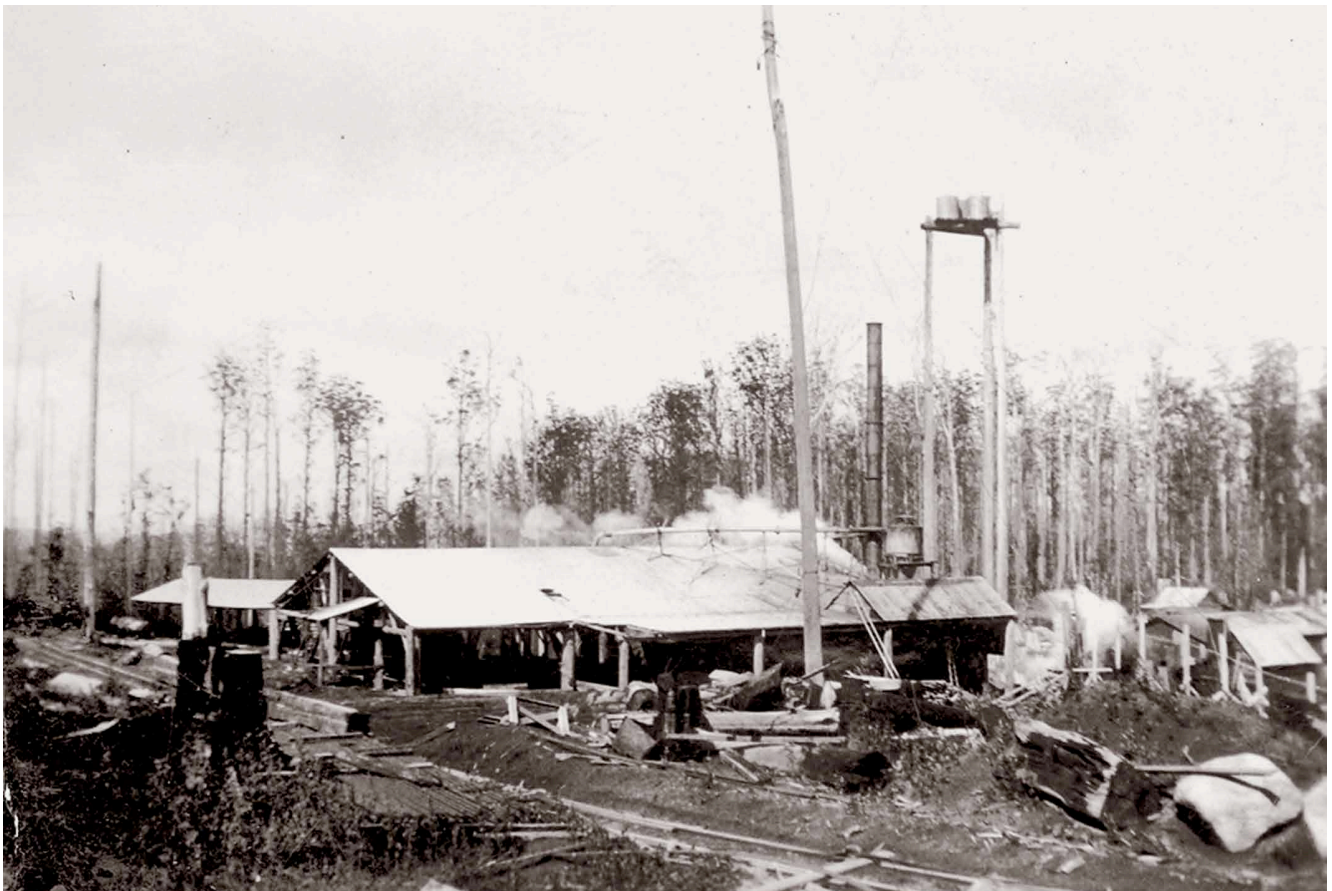
The Federal Mill in the early 1940s with three feet gauge log tramway in foreground. The earlier four feet gauge line to the south had been removed by this time.
