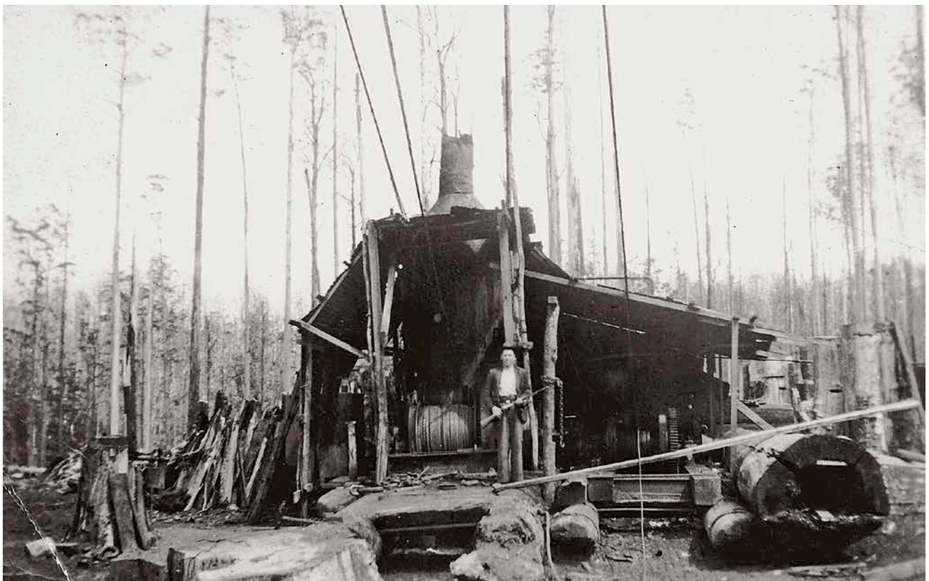
The Washington Winch with smaller motor winch alongside at the Federal Mill. The winch hauled logs from the surrounding bush using the high lead system where the logs were raised at the front to aid passage through the bush.
