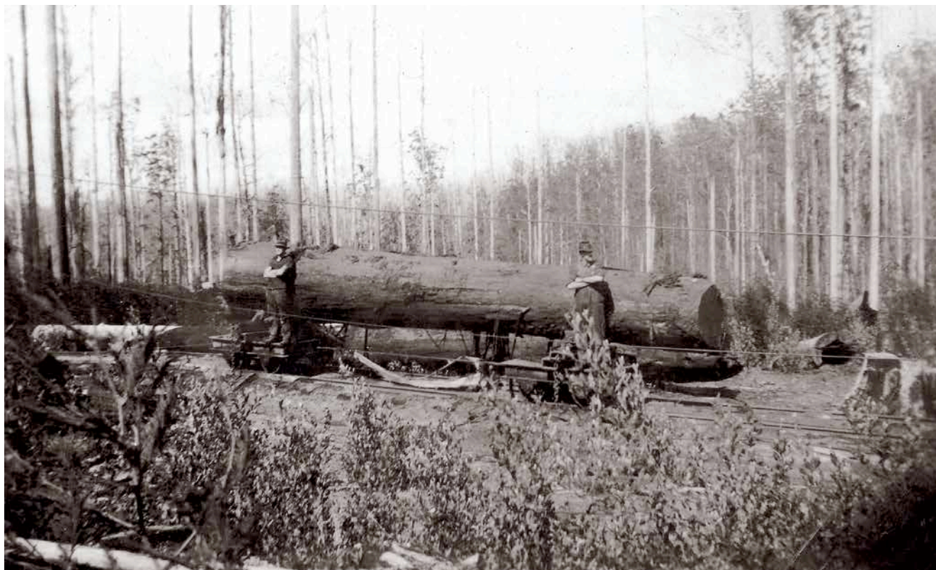
Log under haulage on the Federal Mill winch operated four-foot gauge log tramway that ran south from the mill until around 1940. Photo: D Morrish
