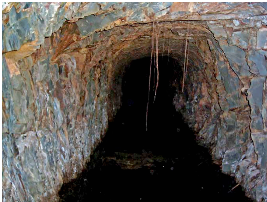
The commodious Vulcan tunnel, approximately 1.4 m wide and 1.7 m high and designed to take two parallel tracks.
