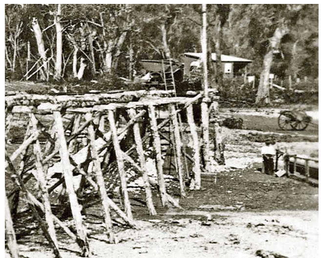
Enlargement of the land end of the temporary staging, showing a small heap of gravel, with skips above. Height to rail level is about 13ft; the sea end being some five feet higher. For full picture, see Light Railways No.251. Photo: John Oxley Library, State Library of Queensland, Neg: APA-114-0002-0007
