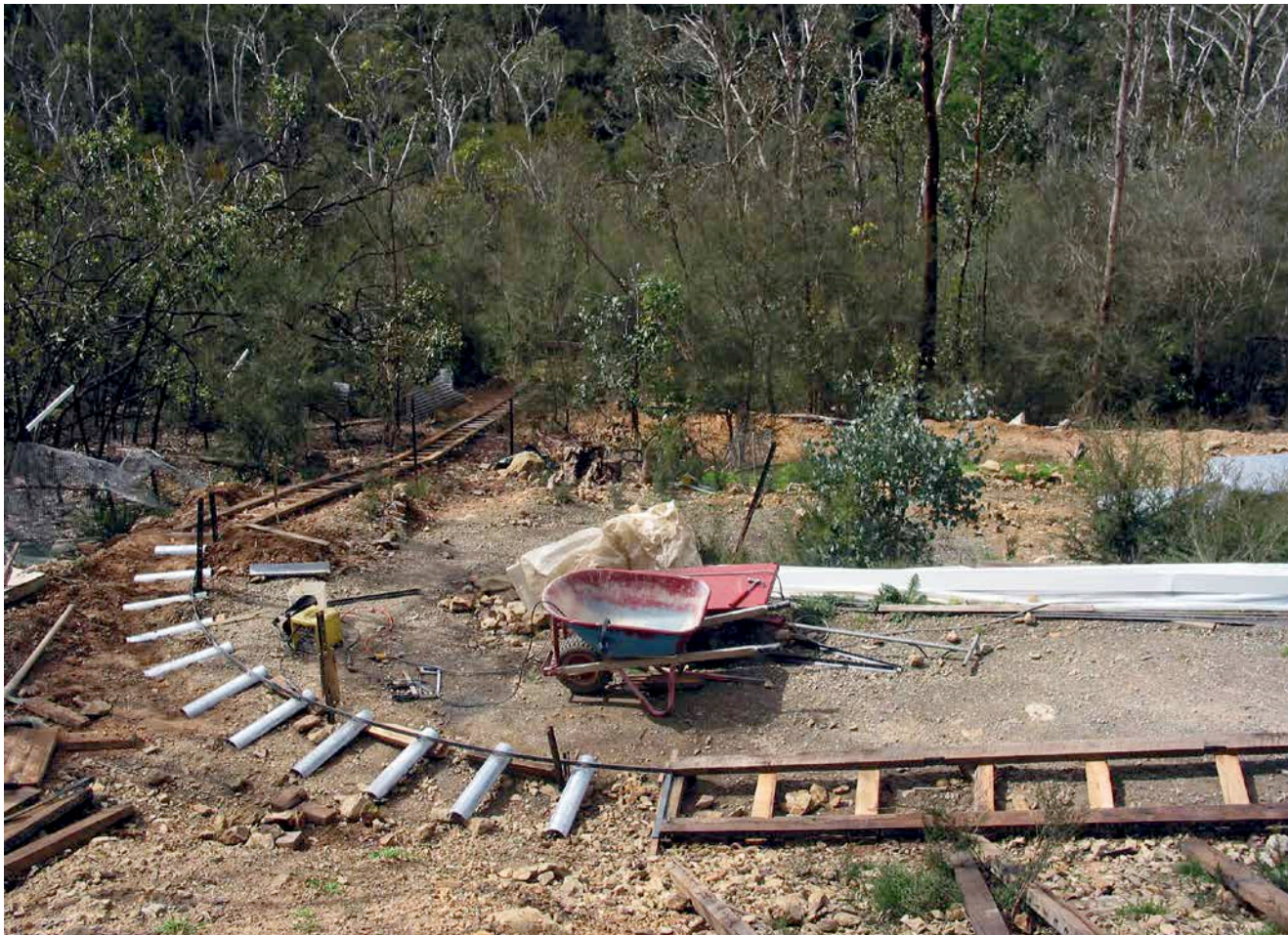
The tramway under construction. The sleepers on the curve were 100 mm water pipe cut in half longitudinally. Steel rail welding is in progress.
