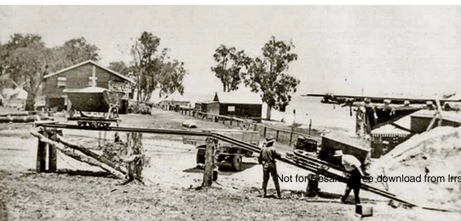
Adjacent to the gravel heaps at the base of the elevated staging (and hidden in the other photos) was this reload ramp. A couple of skips would be filled with gravel and hauled up a short ramp using a block and tackle, with a horse (out of sight to the left) providing the motive power. One of Blake Bros' motor trucks will then be backed under the structure and filled. Photo: courtesy of the Blake family, Bribie Island Historical Society W09_888012
