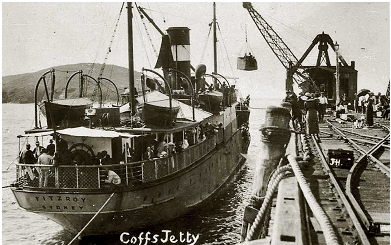
Langley Bros' SS Fitzroy, commanded by Captain James Colvin, taking on passengers at Coffs Harbour Jetty c1913. The steam jetty crane transferred timber, general cargo and passengers to ships which had to be held off the Jetty by heavy hawsers. The same crane loaded CHTCo's timber onto the SS Belbowrie. Captain Colvin was one of the Exclusive Right No.1 Syndicate members. He went down with the Fitzroy when it sank off Tuncurry Beach in June 1921.
