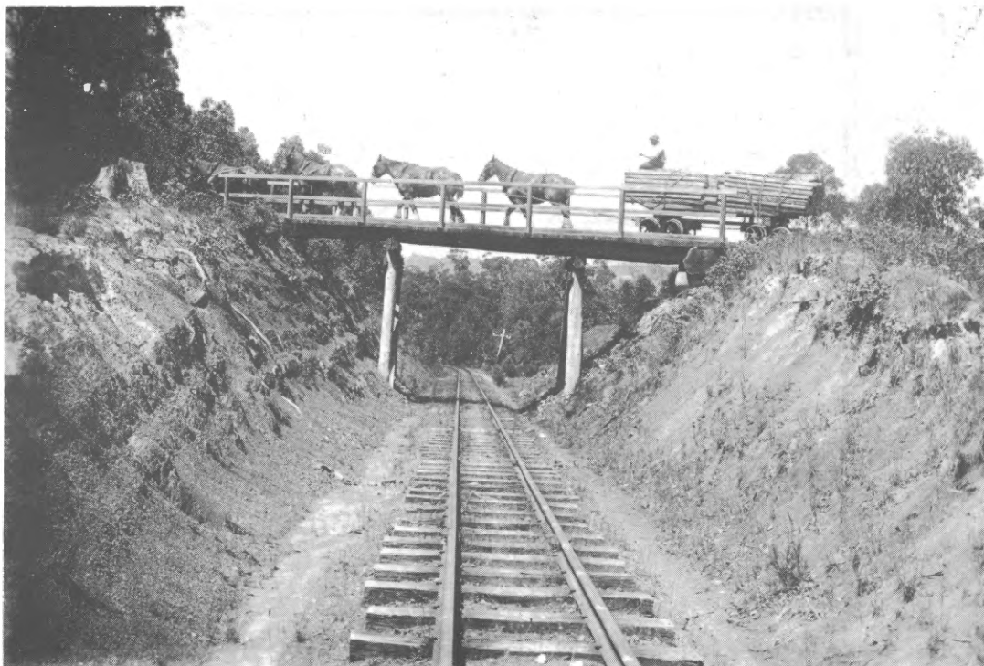
Tommy Brown's tramway bridge over the railway near Gould was the result of some lateral thinking by him in 1929 following the dispute with Tommy Veale over access rights to his tramway. It is the only known instance of a pure tramway bridge being constructed over a VR railway line.
