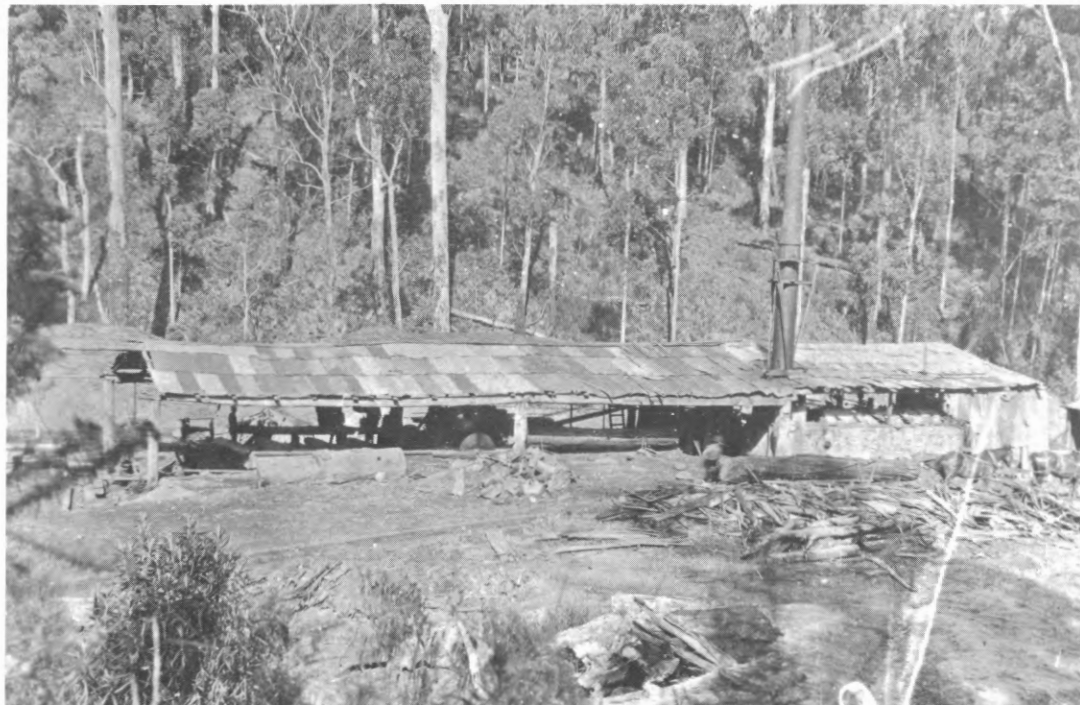
Morgan's bottom mill in the early 1920s. Note the log tramway in the foreground and the large stationary boiler from the Coopers Creek copper smelter. Photo: MJ McCarthy Collection
