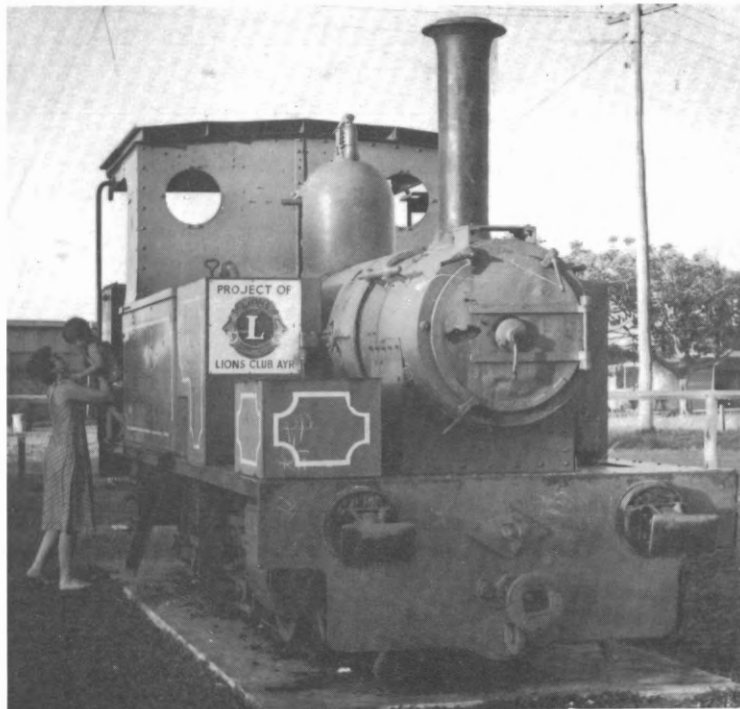
Left At Brandon, near Ayr, Airedale , a 3ft 6in gauge Avonside locomotive can be seen preserved in the park. Despite care and attention, the elements here are too taking their toll and the locomotive is deteriorating. Airedale is unusual as it is a representative of the sole mill system to use 3ft 6in gauge for its plantation haulage, at least in modern times. Some other mills operated 3ft 6in portions of their systems but in conjunction with hauls partly on the QGR, while generally retaining 2ft gauge light railways or tramways for plantation haulage purposes.
