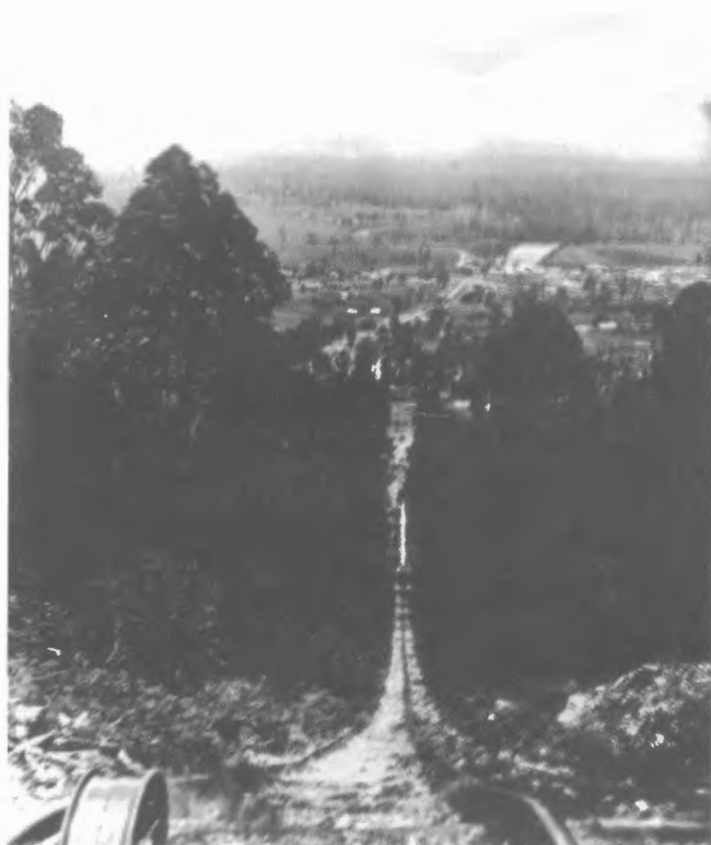
A view looking down the Alum Mountain Incline with Buladelah village in the background. The cast iron roller once carried the rope over the brow and the absence of the latter leads to the conclusion that the photo was taken after the incline closed.
