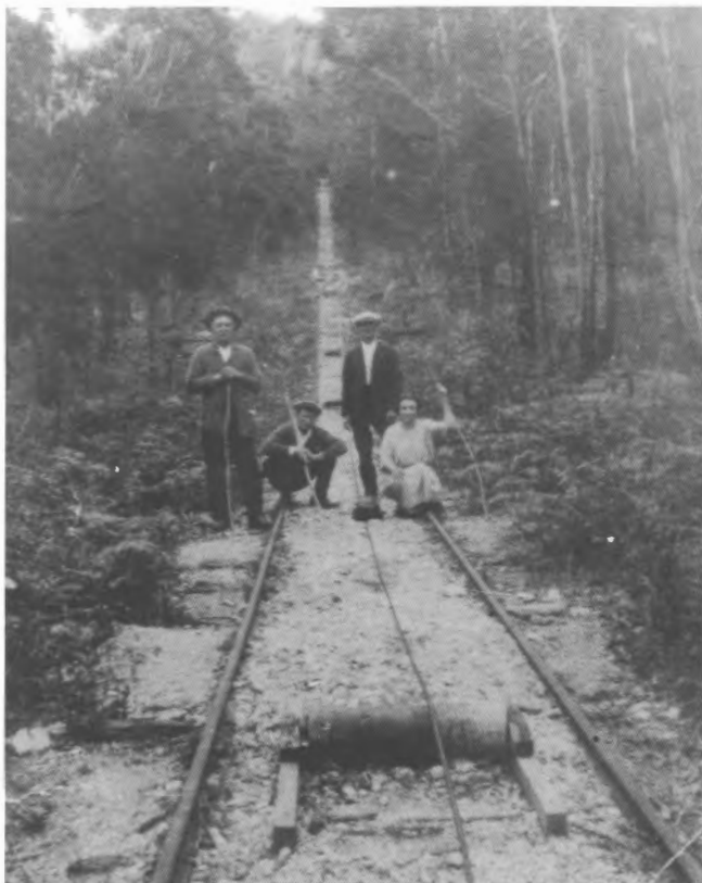
Looking up the Alum Mountain Incline, well strewn with spilled alunite. The track gauge can be estimated by comparison with the figures in the group. Of note is the (very) light rope and the wooden roller. The centre passing loop can just be discerned up the hill, and the style of clothing would indicate the photo was taken in the 1920s.
