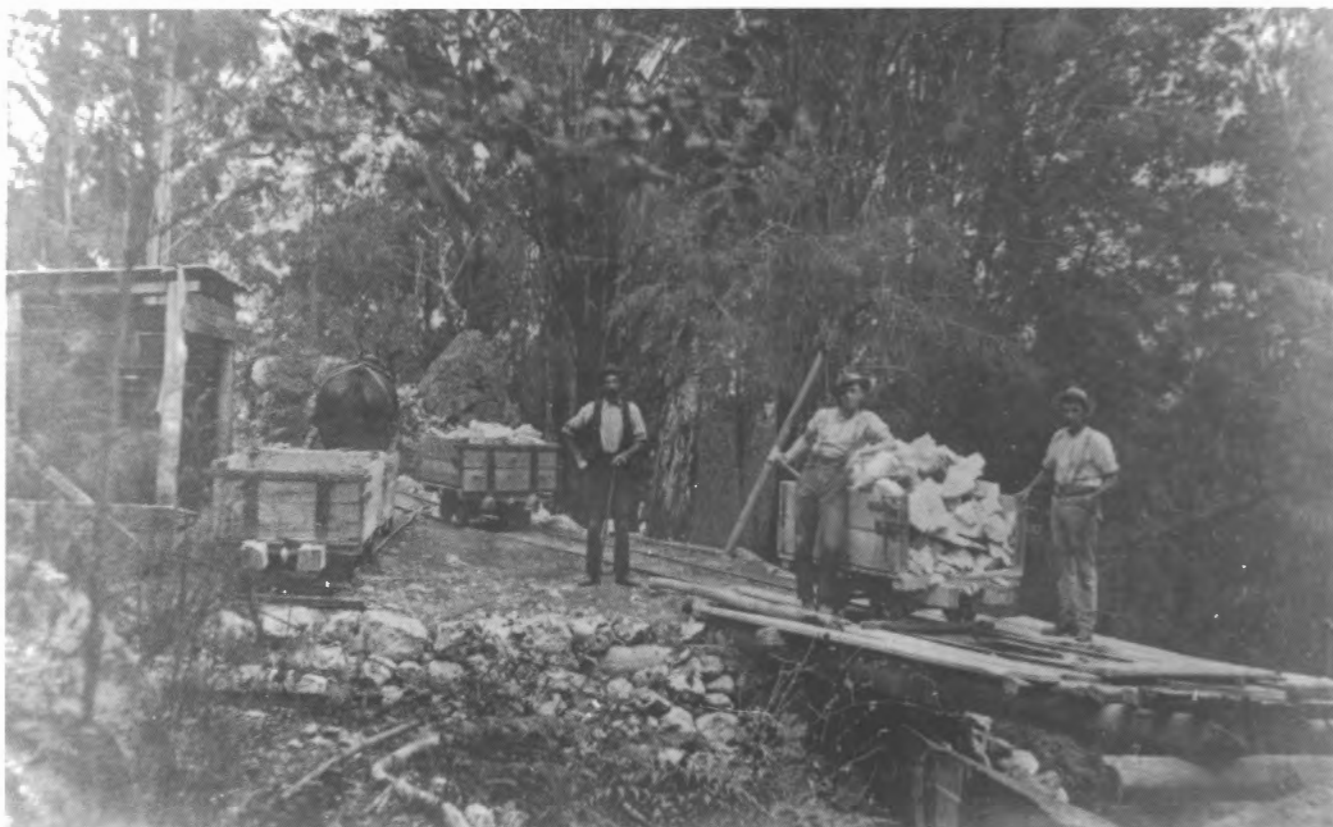
The incline loading point which served the Tunnel and Myall Quarries. The horse has brought in two loaded skips and is now hooked onto two empties in the shunt outside the smithy. The driver (in waistcoat) will soon take him back to the faces. Meantime one of the loaded skips has been run onto the staging and the end door removed and thrown aside (by the man leaning on the skip holding the hammer). Next the two brawny young fellows will use the long poles to lift the rear of the skip, (the sleeper across the rails across the rails acting as a fulcrum) so the remainder of the 30 cwt load will fall through the hole in the staging directly into the (just visible) incline truck. Photo: Bulahdelah Historical Society Collection
