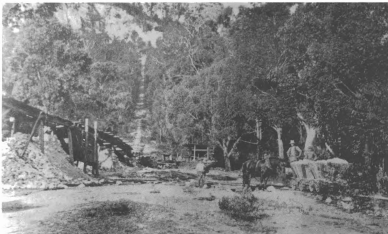
The incline foot site around 1924. The trestle has been shortened and the wharf line has been in use for 15 years. Two loaded trucks are about to gravitate to the river, the set rider on the back truck operating the brakes. The horse has pulled the trucks from under the bins and now waits with the driver to follow down and bring back the empties.
