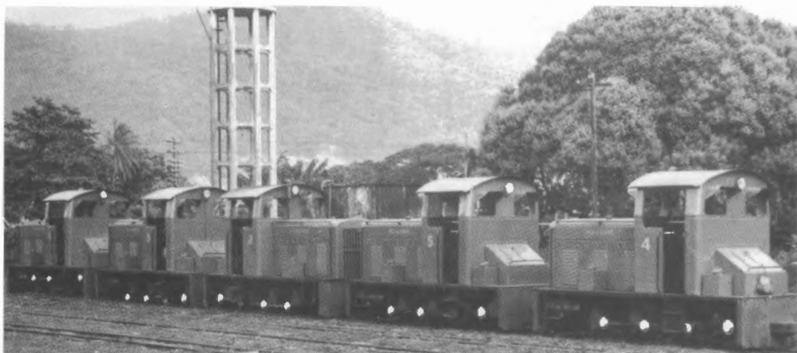
Mulgrave sugar mill became interested in the benefits of diesel power quite early and, in 1953, imported a Baguley/RMP model BG6 0-6-ODM from Britain. Two years later, it became the first mill to completely dieselise its tramway system, with the bulk purchase of five ComEng model A 0-6-ODM machines, here seen lined up in the mill yard shortly after delivery. Photo: John Dunn collection
