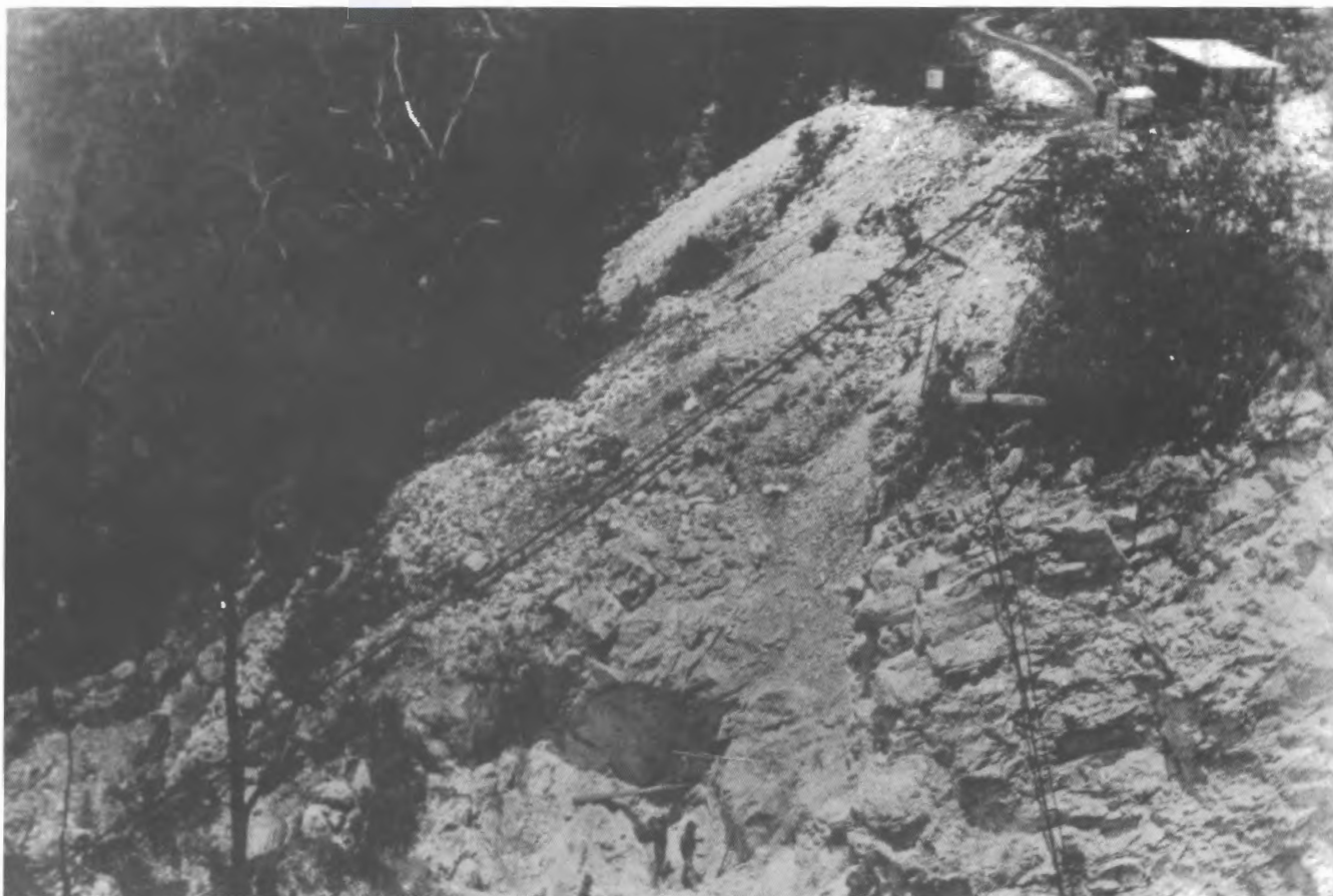
The Big Quarry Incline. When the working faces in the Big Quarry descended below the main tramway level, a powered incline was necessary. Beyond the crude shed housing the boiler and steam winch is the track running to the main incline. Photo: Bulahdelah Historical Society Collection
