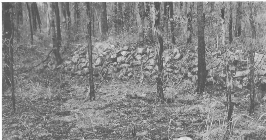
A dry stone embankment leading to a small bridge site at the left of this photo. The abundant sandstone rocks on the centre hill sections of the Markwell tramway made excellent construction materials. Long sections of stone ledges, embankments and bridge abutments are still evident in this area. Photo: Ian McNeil.
