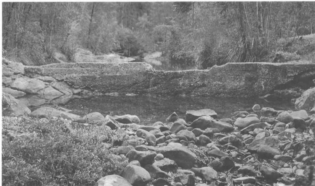
The Markwell sawmill dam built in 1913. This small concrete dam was built across Deep Creek adjacent to the mill. It is still mostly intact some 80 years later and forms a popular swimming hole in summer. Photo: Ian McNeil.
