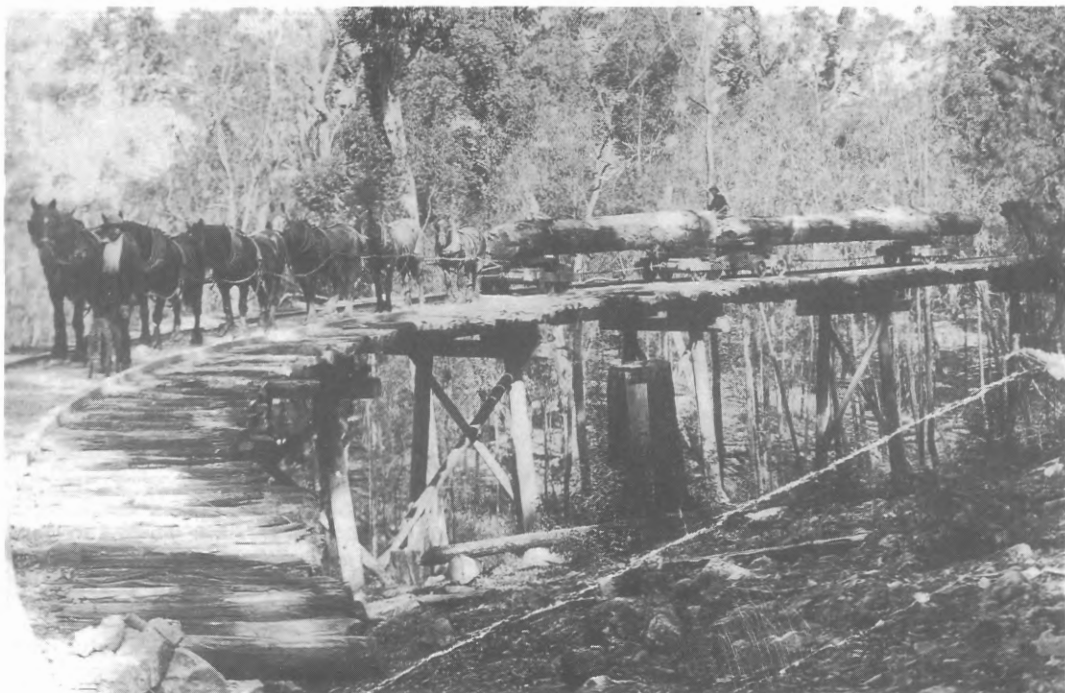
A horse team posed on the Markwell tramway with saw logs for the sawmill. This photo was taken from the downhill end of "The Camber", the 180 degree curved bridge 5.5 km out from the mill. There is a second horse-team just visible behind the first. Photo: Bulahdelah Historical Society per Roger Persson.
