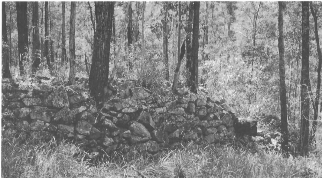
The top stone abutment of "The Camber" bridge. The approach embankment is on a very sharp curve nearly 40 metres long and built from local rocks. It is two metres high at the end. The wooden bridge continued on the same sharp radius, curving away to the left of the photo. Photo: Ian McNeil.
