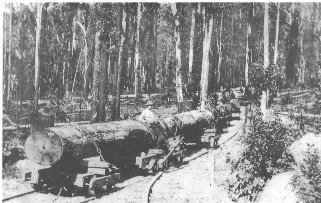
Saw logs on the Markwell Tramway headed for the mill circa 1912. The width of the standard-gauge log bogies is clearly evident in this photograph. The location of this tramway junction is a mystery because the relatively even nature of the terrain in this photo does not match the rugged topography of the junctions identified so far. Photo: Bulahdelah Historical Society per the Late Ted Baker.
