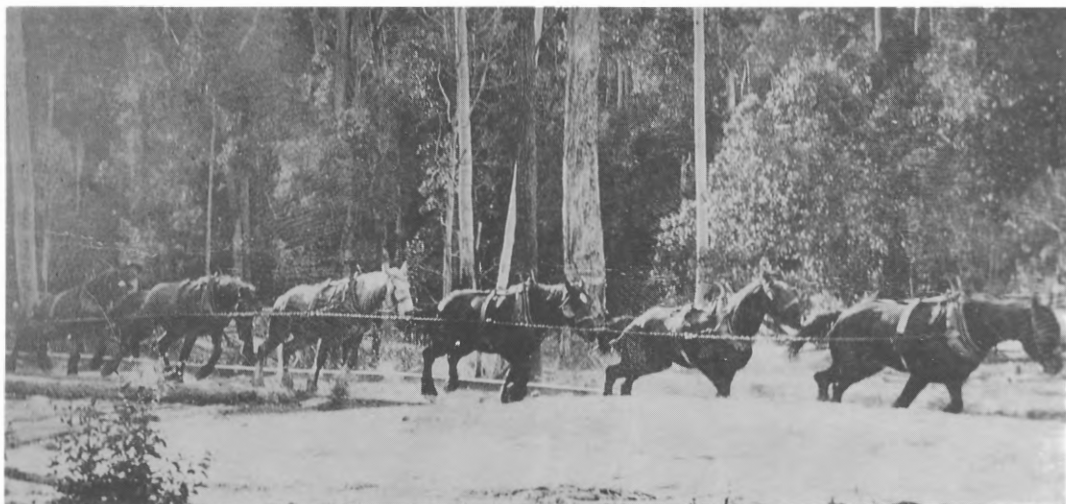
Not all the grades were in favour of the load as this action photo on the Markwell Tramway shows. A six-horse team is working hard on one of the short uphill sections on the way back to the mill. This photo was probably taken about 800 metres from the mill. Photo: Bulahdelah Historical Society per the Late Ted Baker.
