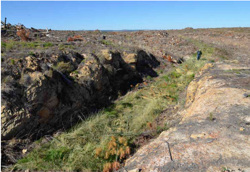
A short, 3-metre deep rock-walled cutting with a 2-metre high approach embankment (digitally enhanced) curving off to the left behind it. Clear-felling of the 30-year old pine plantation has left an unsightly lunar-like landscape, but in years to come the old formation will be preserved and enhanced as an avenue bordered by stately pine trees. Photo: Jeff Moonie
