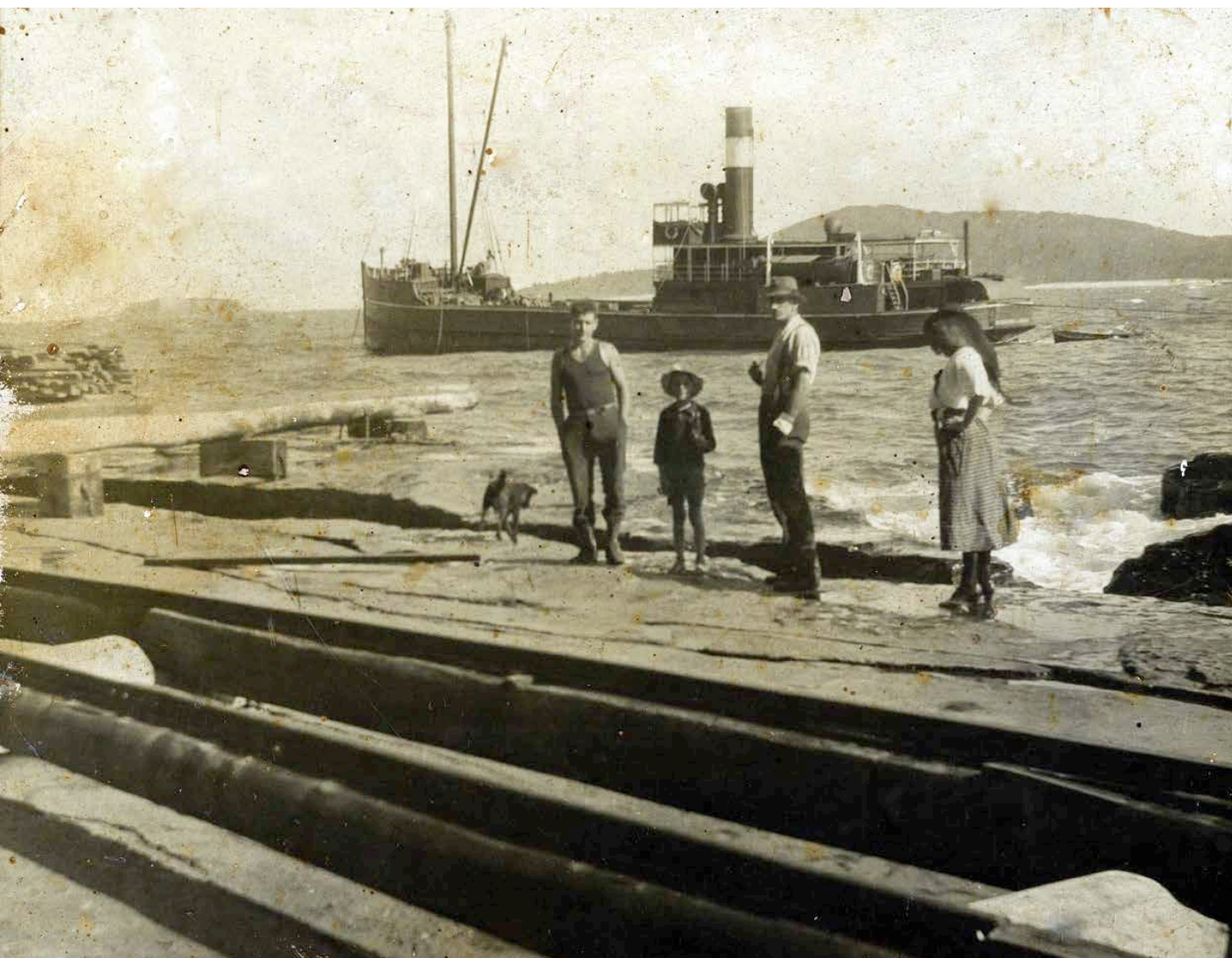
The loading area showing tramway, skids and the SS Bergalia offshore circa 1927.
