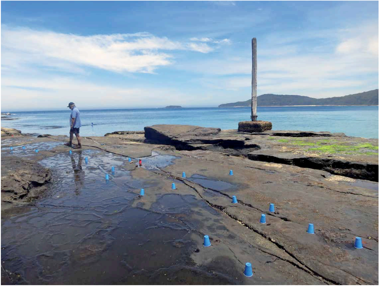
The loading area showing the use of paper cups to show bolt locations.
