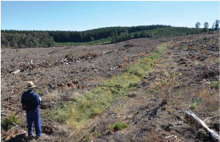
The tramway crossed this 2m high embankment (digitally enhanced) over a shallow drainage depression and entered a small cutting, seen in the distance, before entering the Mount David State Forest pine plantations. It extended a further 1.5km to the forest terminus but deep contour ploughing during pine planting had obliterated the light earthworks in this section. Photo: Jeff Moonie
