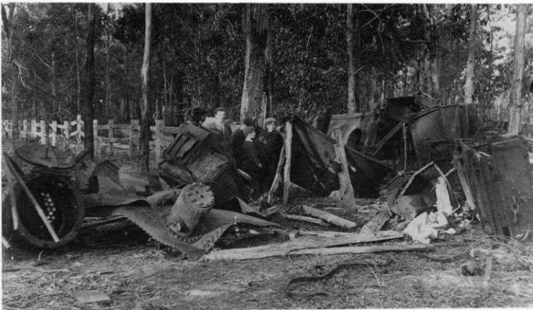
Left: The remains of Mona after the tragic boiler explosion on 1 September 1914, which killed the driver, Bill Dudley. The violence of the accident is clearly evident with the locomotive having been thrown several metres from the rails.
