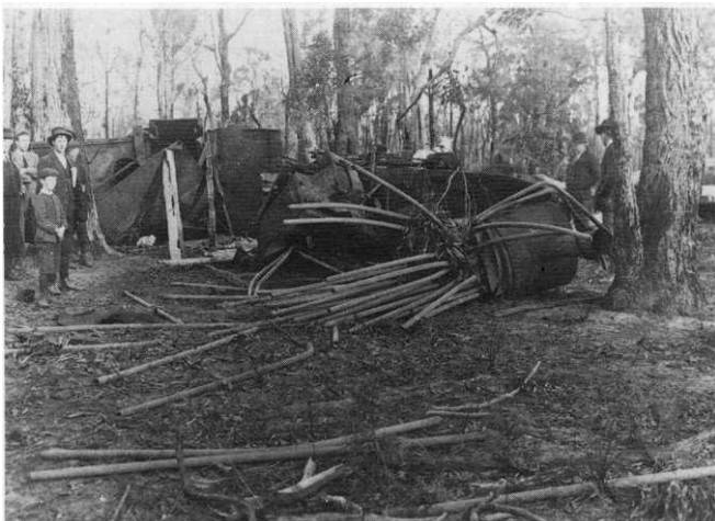
Right: The remains of Mona following the boiler explosion. It is clear from the photograph that the point of failure was at the back end of the boiler.
