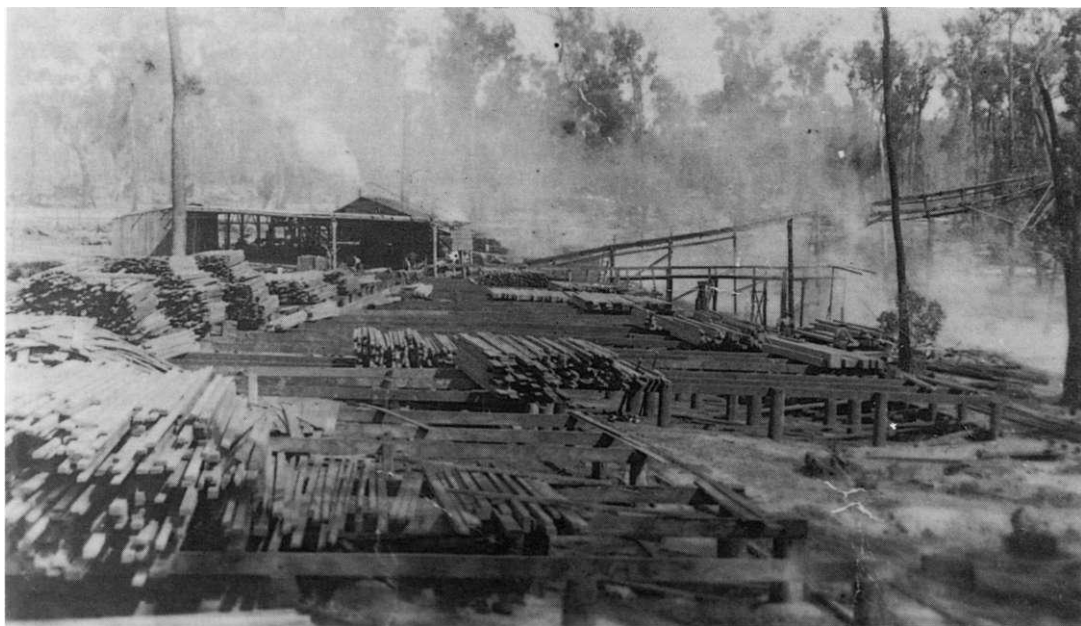
The Goodwood sawmill post the 1912 enlargement of the milling plant. Note the sawdust conveyor. In the context of Victorian sawmilling this was an innovative and unusual addition to the mill Photo: A. Robinson Collection
