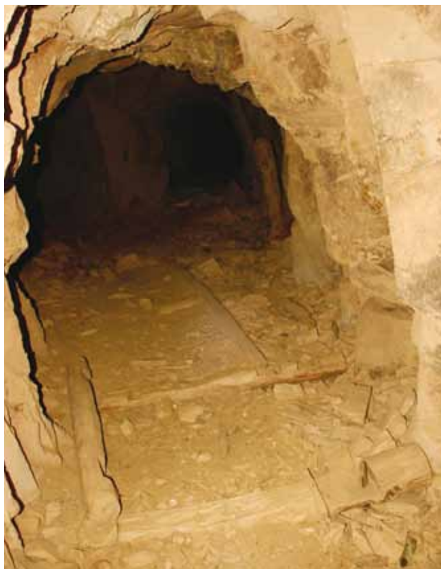
Remains of a wooden set of points in the lower adit underground at the Jeff Davis mine, 18 October 2008. The timber at right shows how the round sleepers were notched to accept the wooden rails. Photo: Andrew Swift
