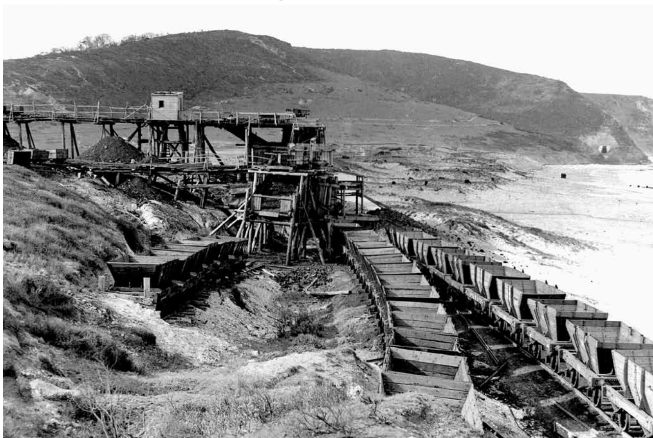
Glenrock Colliery screens and sidings: The basic nature of the screens and sidings for Glenrock Colliery No 2 and 3 entries is apparent in this photo taken, looking north, around 1940. Smelters Beach is on the right, and the southern portal of the No. 2 railway tunnel is clearly visible in the background, where the hills forming the Merewether Ridge sweep down to the ocean. Photo: ARHS Railway Resource Centre
