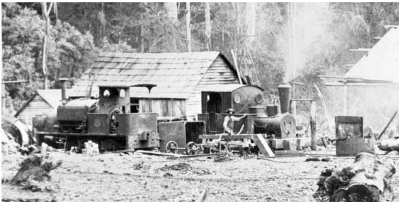
Locomotive maintenance area at Sanderson's Noonday Creek mill, c. 1904. On the left is Hudswell Clarke 0-6-0ST TOM CUE (B/No. 378 of 1891), and on the right Bagnall (B/No. 682 of 1885) 2-4-0T, WESTWARD HO (formerly KHARTOUM). Like PARROT, WESTWARD HO was not built for use on a timber tramway, and was underpowered. On the other hand, TOM CUE performed well, as did identical locomotives working on timber tramways in Tasmania and Western Australia. Photo: LRRSA collection
