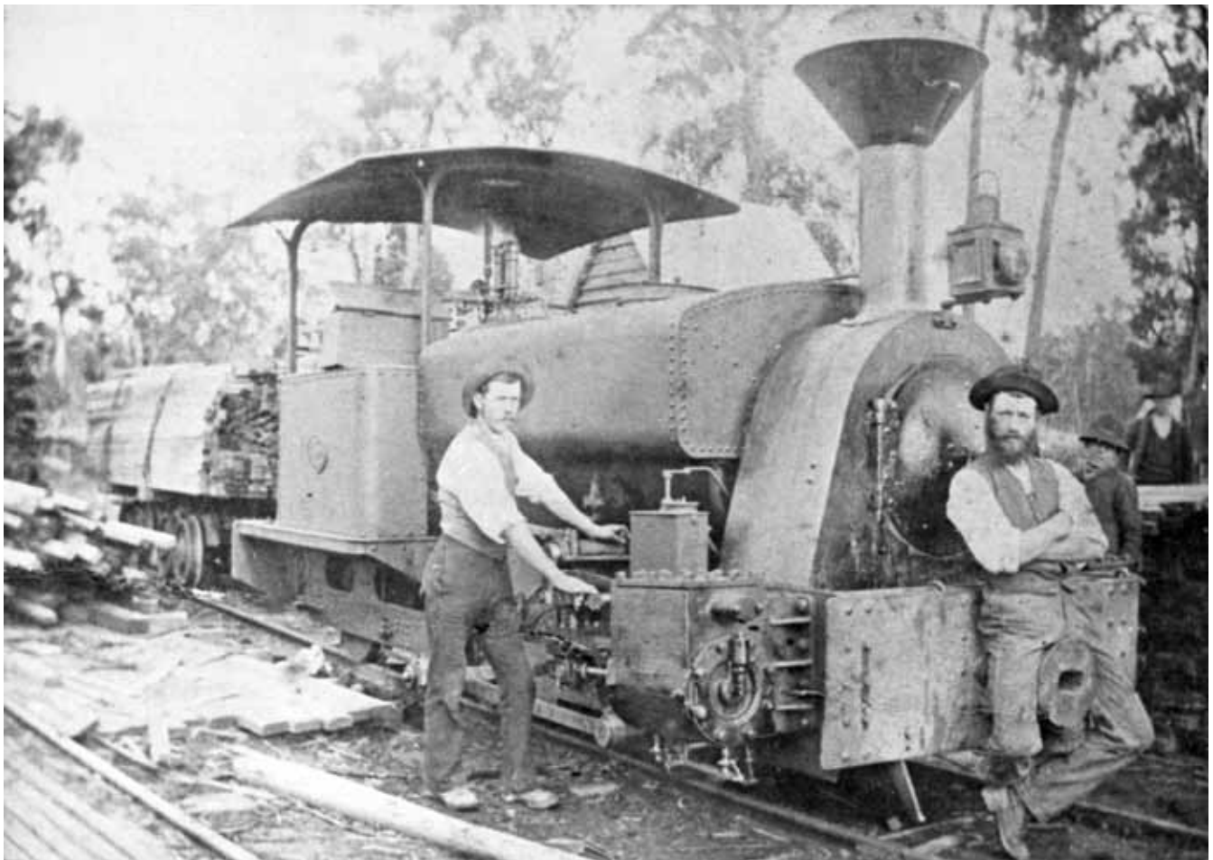
3ft gauge Fowler 0-4-2ST locomotive (B/No 5851 of 1888) seen at Cropley's Darnum-Ellinbank tramway c. 1892. Cropley Bros bought it new and used it for 14 years, by which time it was in very poor condition. Photo: LRRSA collection
