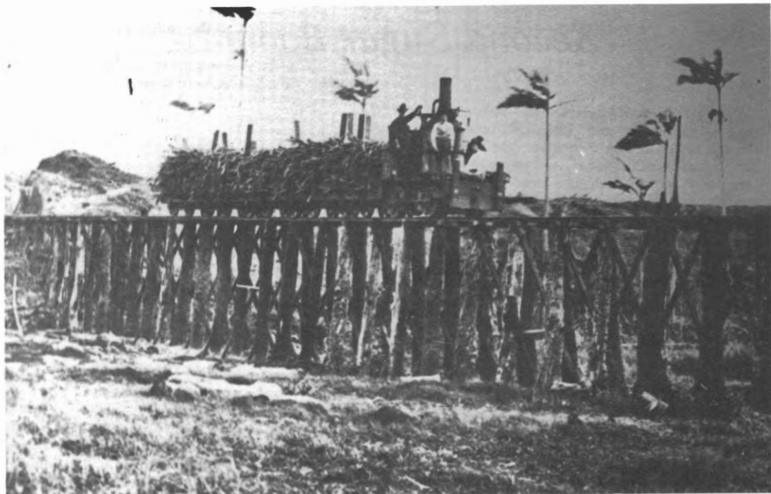
Vertical boilered 0-4-0 locomotive built by Victoria Foundry, Mackay in 1880 for Spiller's River Estate tramway.
