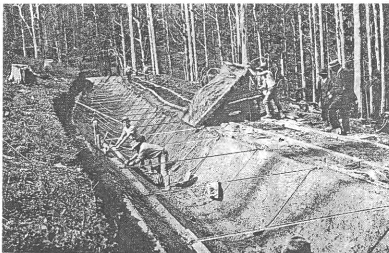
Portable mixing board discharging mortar into the channel.
