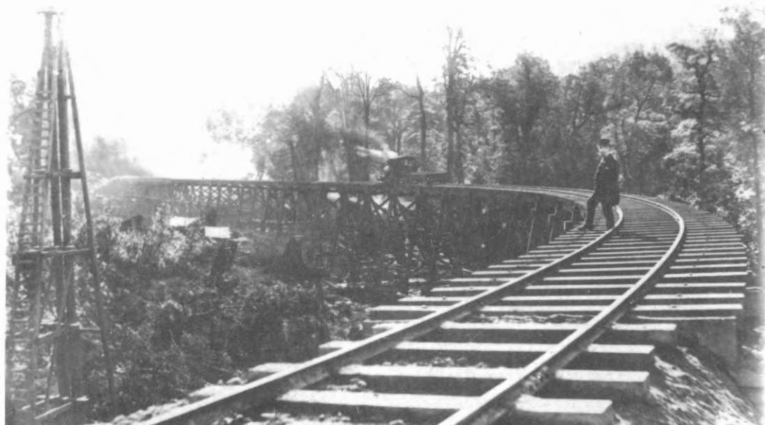
The King River Bridge on the Mt. Lyell Railway soon after the bridge had been completed, and probably taken late in 1895 or early 1896. Note the pile driver beside the bridge in the foreground, and the camp of the bridge construction gang behind. The 0-4-0ST Malvolio (Baldwin 7108/1884) is seen pushing two trolleys loaded with rail across the newly completed bridge.
