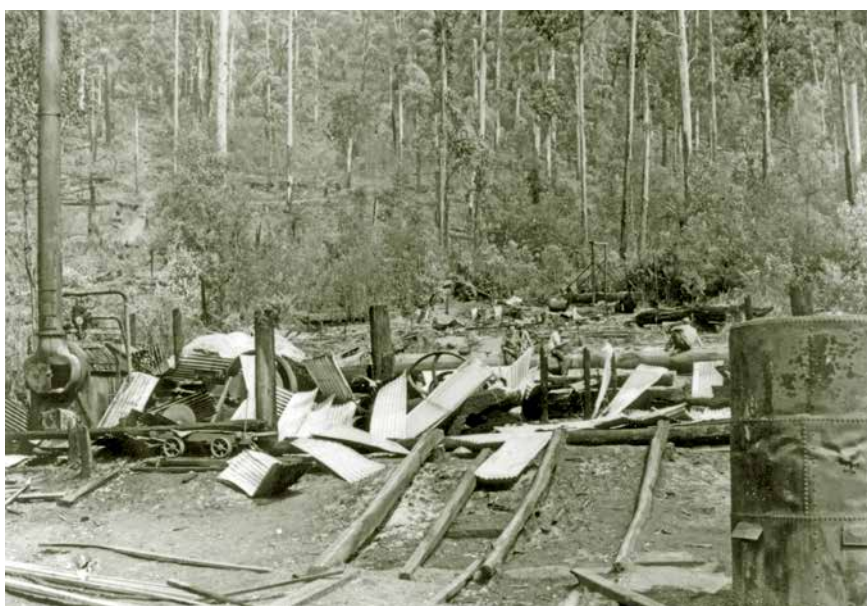
Padgett's / Robbie's mill after the 1939 bushfire. The mill boiler is to the left and, just to its right (partially obscured by sheets of corrugated iron), is the Tangye engine powering the mill. The mill's sawdust burner (an old boiler standing upright) is in the right foreground. Photo: PROV
