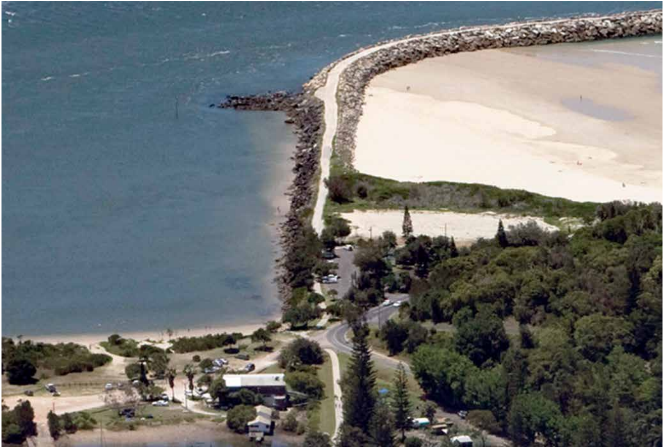
An aerial view of the South Breakwater. The straight section in the foreground was built on Moriarty's watch in the 1860's, the remainder 100 years later. The short stub projecting into the river is the T-piece, formed in the 1890's when a storm washed away the end of the breakwater.
