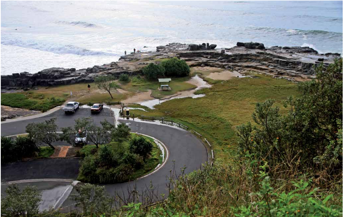
South Head Quarry, 2013, with the South Breakwater in the background. The quarry floor is now a car park and a picnic area. Rock was quarried out to below sea level, leaving only a narrow rim as protection against breaking waves. Photo: Robin Knight
