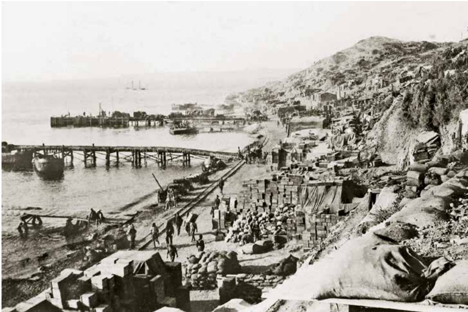
Left: Anzac Looking north across Anzac Cove to Ari Burnu. Three jetties are visible, the two more distant seemingly having 2ft-gauge tramways, accessed via a turntable at the jetty base. In the distance, the tramway continues around the headland (Ari Burnu) to North Beach, seen in the photos on the previous page and, behind the photographer, to Brighton Beach
