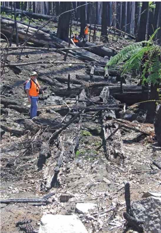
E: Scott Gould examines the remains of a bridge just north of the Black Range Road. Photo: Peter Evans
