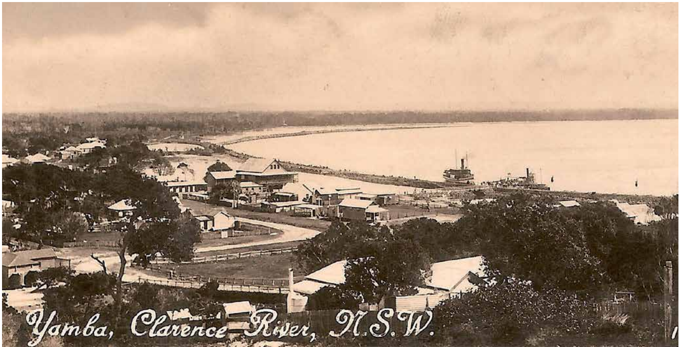
An 1888 panoramic view of the South Training Wall extending up river towards Rabbit Island. The two small coastal steamers are docked at Yamba's public wharf. The bays behind the wall were filled in with dredge spoil during the 1950s and 60s. Photo: Port of Yamba Historical Society
