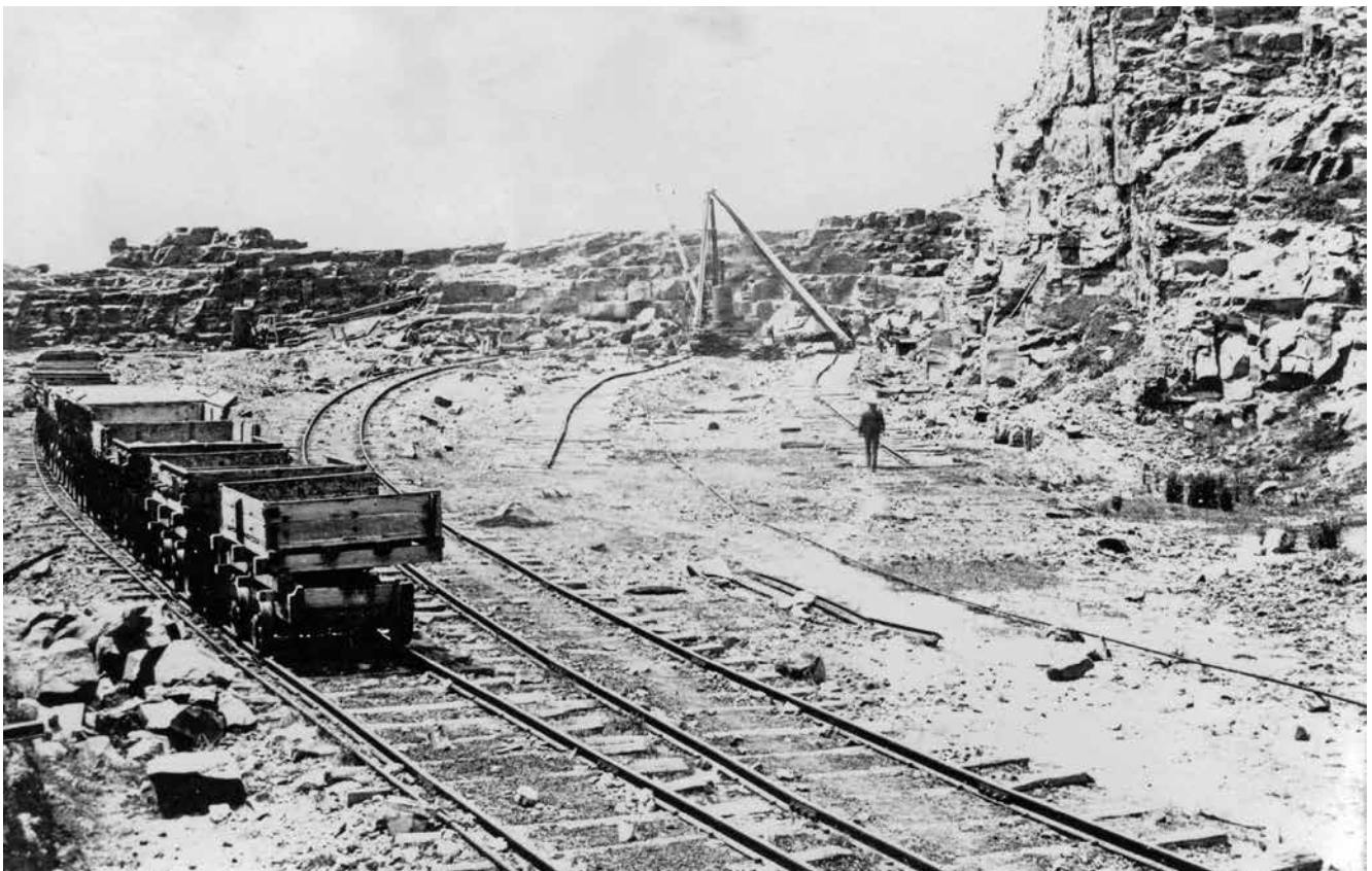
South Head Quarry circa 1888. Empty standard gauge tip wagons stand on the quarry sidings while in the background is a small steam derrick crane and a steam drilling rig.
