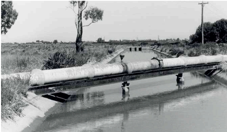
The former tramway bridge in use carrying a water main over the No 1 Channel near the Red Cliffs Pumping Station in 1974. Photo: Mike McCarthy
