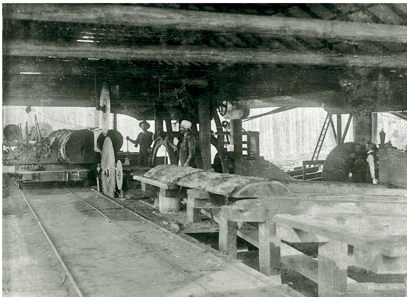
The Nondaville Mill's big Waterous Canadian log saw cost £1,450 and was imported from Brandford, Canada. Its twin circular saw configuration was capable of ripping through a 20 ft long log in under 30 seconds. The mill was laid out on a slope so that sawn slabs slid down runners from one saw bench to the next then and on to rail trucks waiting on the Boambee Tramway. Photo: NSW State Library
