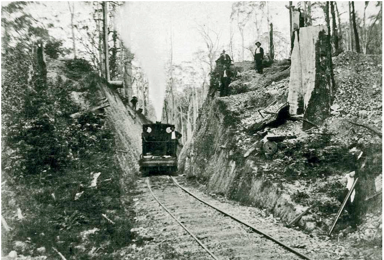
0-4-0ST Andrew Barclay 237/1881 poses with well-dressed company officials in a narrow cutting on the Boambee Tramway. The presence of freshly-excavated spoil above the cutting suggests the photograph was taken either during or shortly after the opening of this section of the line in 1914. The figure in the right foreground is thought to be the photographer's assistant holding a flash-powder stand. Photo: NSW State Library
