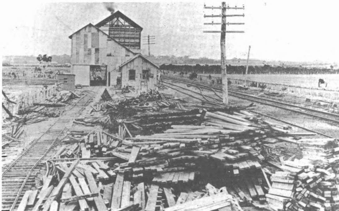
The Marshall pipe factory in the course of erection. The railway siding can be seen on the right while in the centre foreground are stacks of rails and sleepers for the tramlines. GRHC photo
