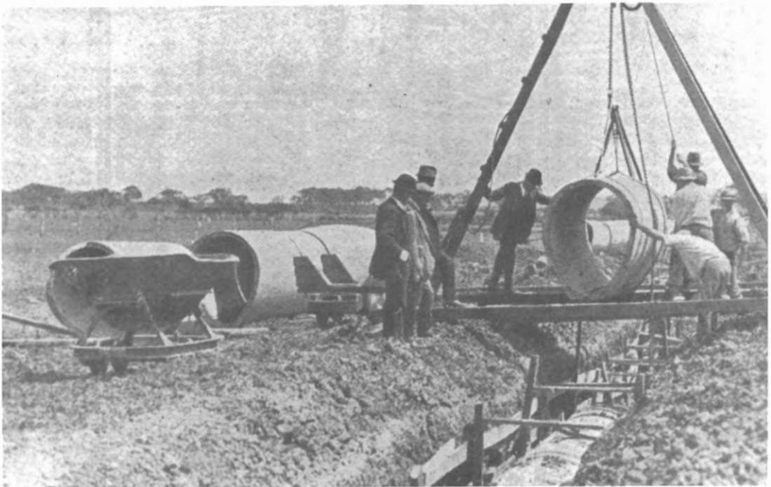
Laying pipes in the trench. A skip and pipe truck stand on the tramline to the left.
