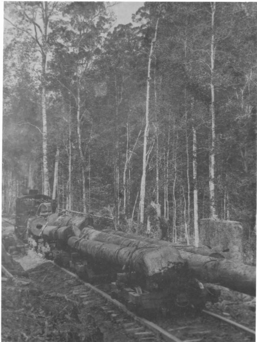
A log train running on the original wooden rail track. Photo: Courtesy P. Sellers.
