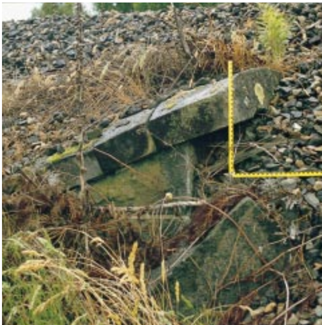
Wing wall of the bridge over the Surry River anabranh.
