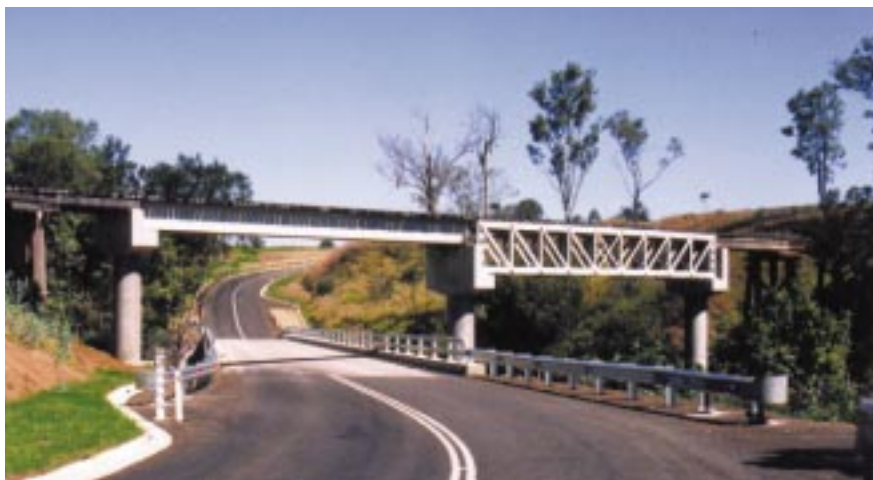
Bingera Mill's Currajong Creek bridge at Wallaville (see LR 143 p.18) as rebuilt shows a combination of concrete, iron and timber construction. The iron lattice span over the creek is ex-QGR and said to date from the 1860s!
