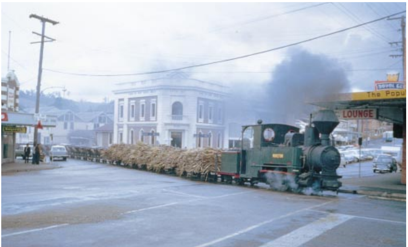
A favourite subject for photographers then, as now, was a loaded cane train crossing the Bruce Highway at Nambour, about to tackle the final short grade up into the mill yard. Here, in September 1965, the motive power is MORETON, and its train consists of a mixture of loaded whole-stick cane wagons and empty side-tipping ballast hoppers.
