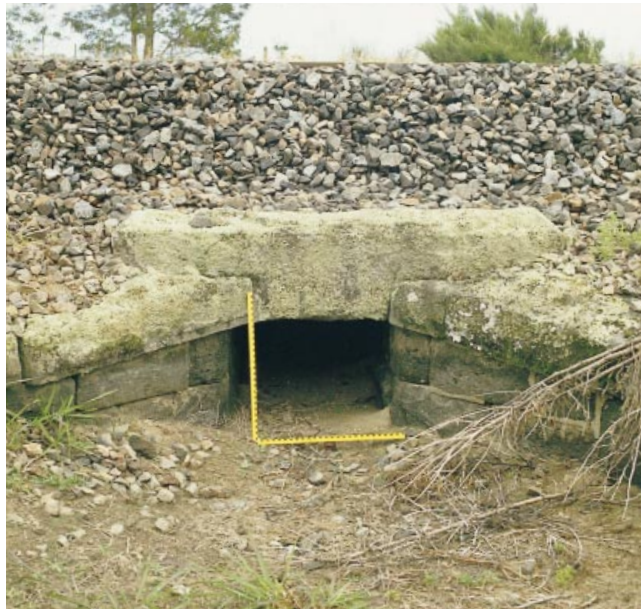
Culvert 1 km north of the Surry River. The coping was added during the construction of the railway.
