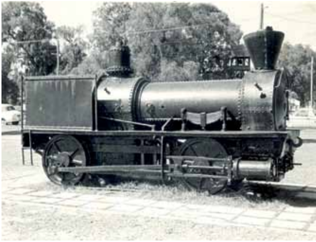
BALLAARAT 'in Victoria Square, Busselton, c1950s Photo: Rail Heritage WA Collection
