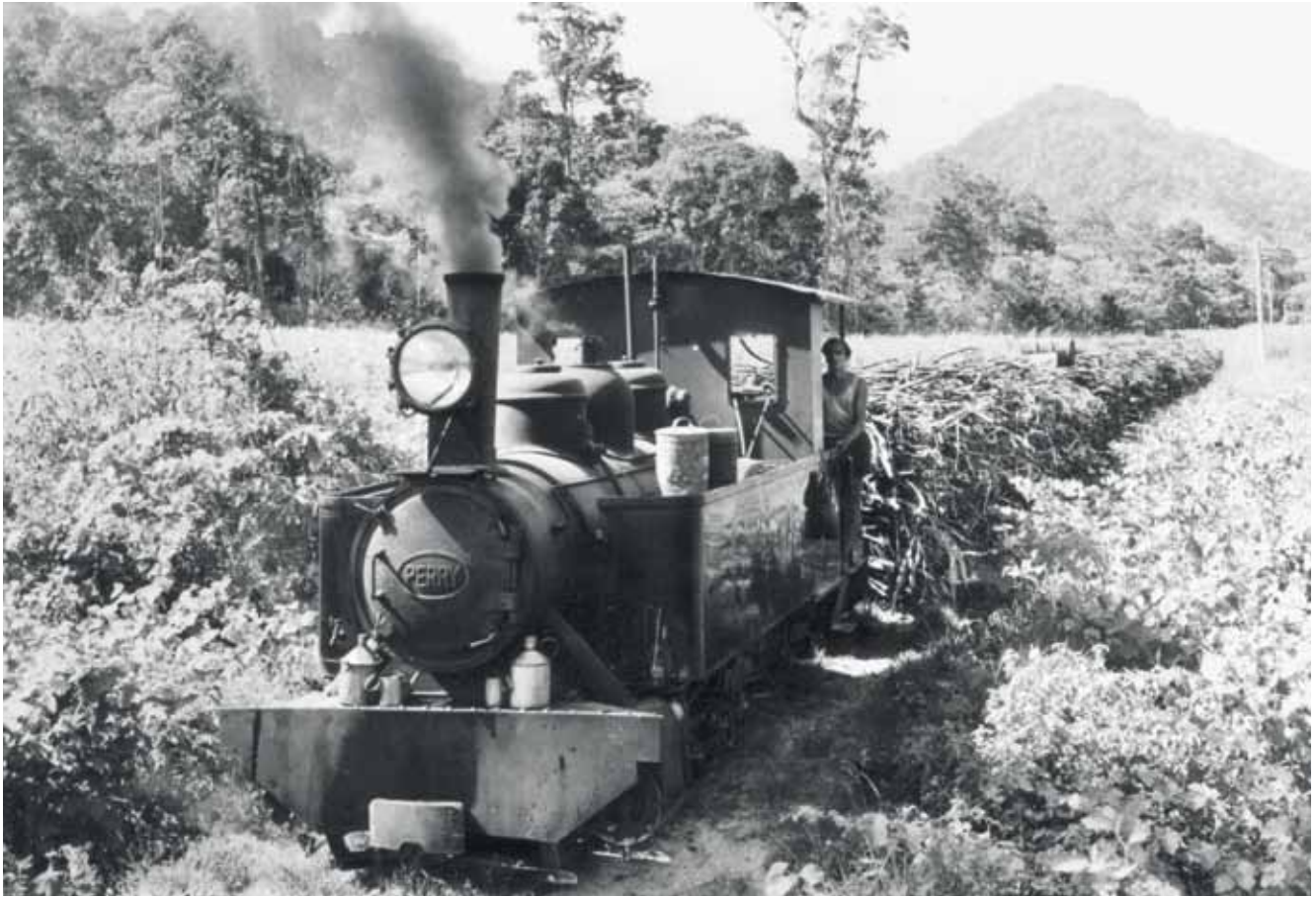
With shiny side tanks, a clean number 7 Perry loco (7967.50.2 of 1952) was photographed during the 1954 season as it neared the top of the range just before crossing what is now the old Bruce Highway.
