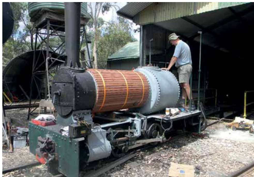
Karri timber lagging being applied to the stripped-down boiler of 0-4-0STMARGARET (Bagnall 1801 of 1907) at the Cobdogla Irrigation & Steam Museum in February 2012.
