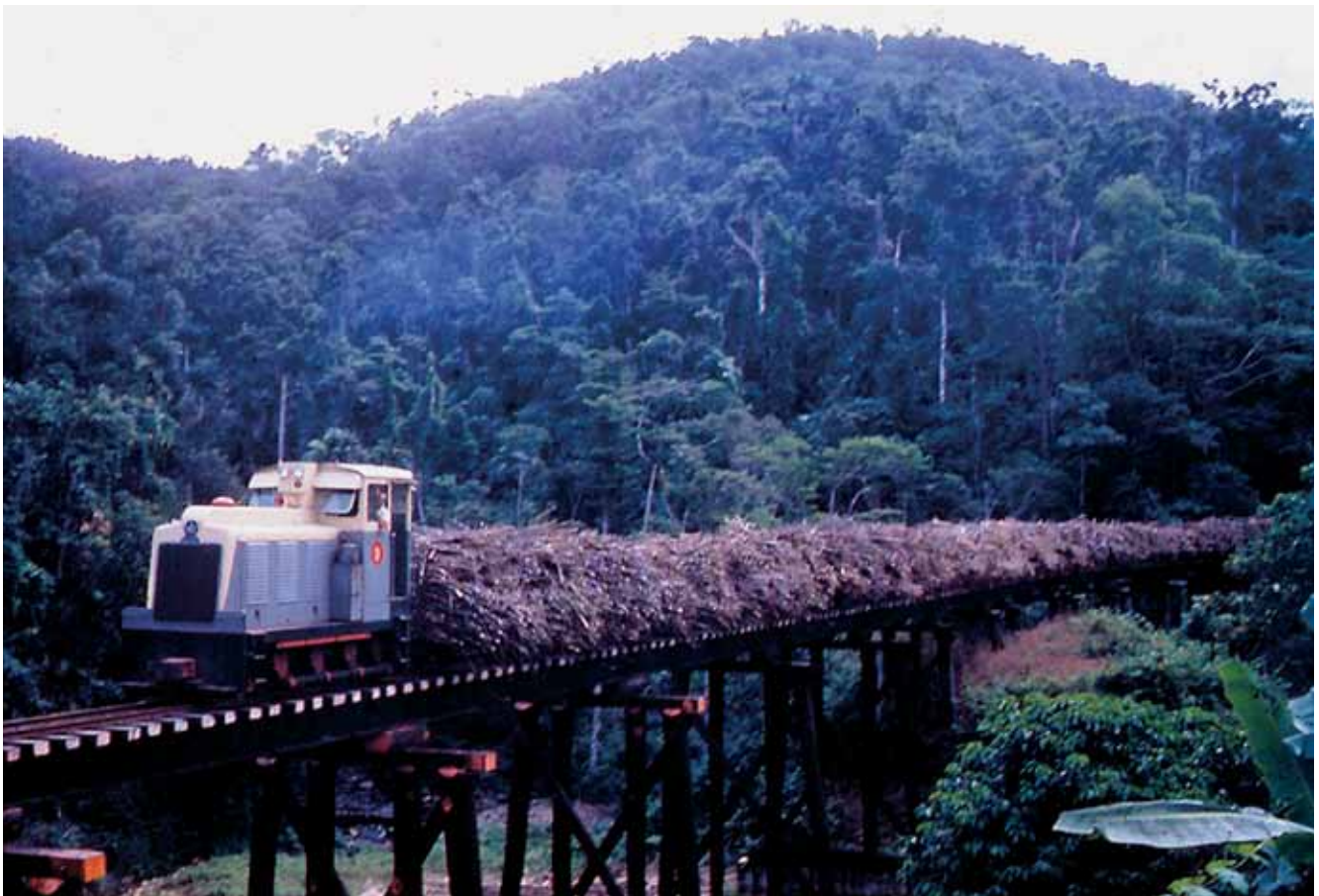
Clyde 0-6-0DH 9 (DHL 4 of 1954) crosses the Hogan's Creek bridge with a full rake. The photographer is standing at the old Range Camp depot. Photo: Len Heaton
