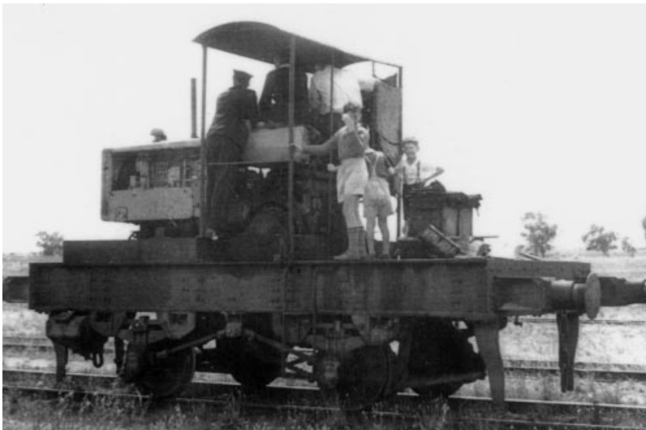
The rebuilt locomotive, now fitted with a rudimentary cab, runs around the baloon loop at Outer Harbour in 1949. An SAR guard (back to camera) supervises the operation, while some local children enjoy the ride. Photo: Colin McLachlan
