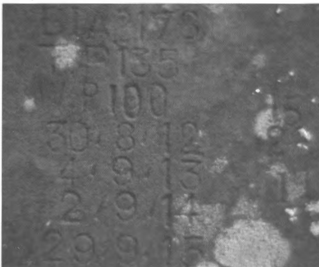
BLA 2178 was Marshall 28708 of circa 1902, a portable steam engine first registered to Toombullup sawmillers Hill & McPherson, and last used to drive Clark & Pearce's "Old" No.4 sawmill in the Rubicon Forest. The photograph shows the typical stamps applied by the boiler inspector at the time of registration. Note the regularity of the subsequent yearly inspections. Photo: Peter Evans
